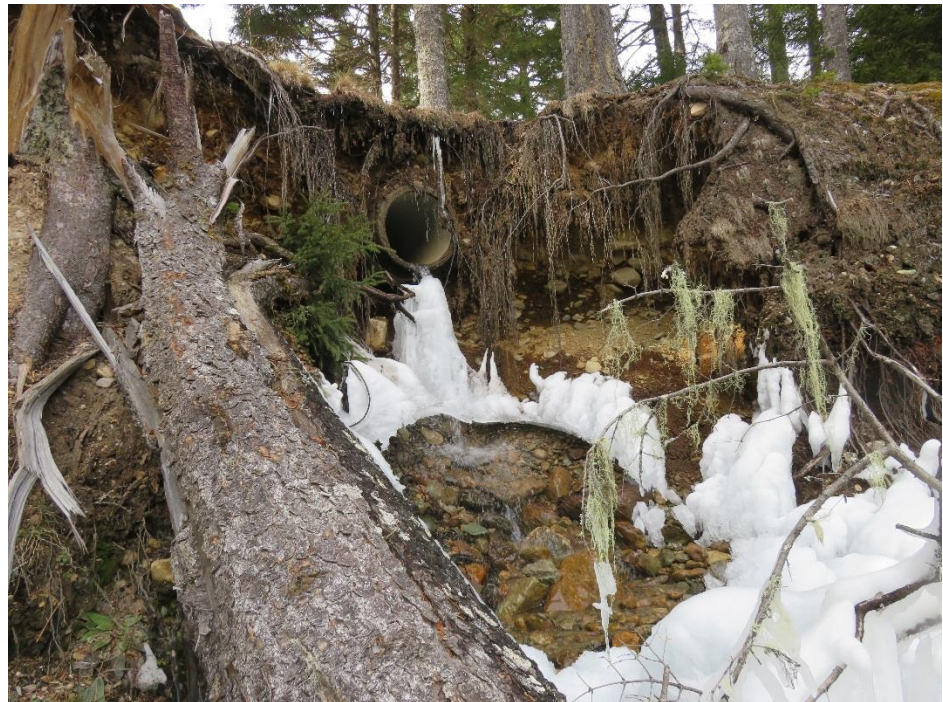
Figure 7: Displacement of Vegetation, Organic Material and Soil
