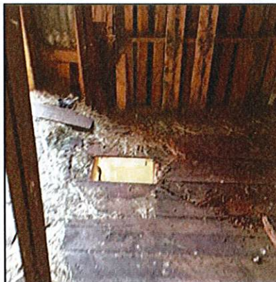
Photo 13: Missing floor boards
