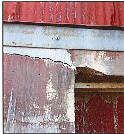
Photo22: Cracks in repair mortar
