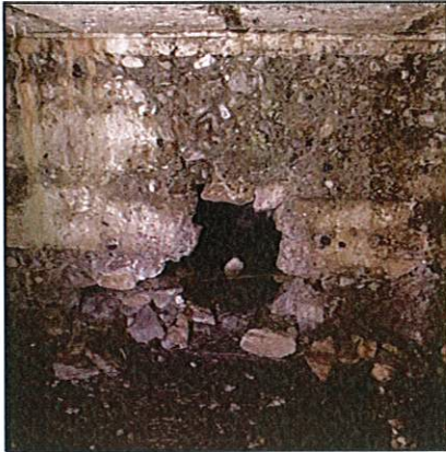
Photo 25: Intermediate wall support in collapse state
