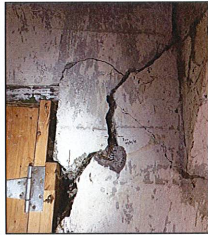
Photo 17: Major cracks around openings
