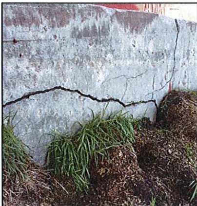
Photo 23: Repairs attempt with bearing angles and repair mortar
