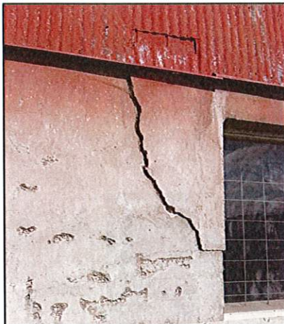
Photo 18: Major Cracks around openings
