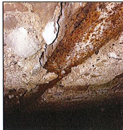
Photo 24: Improper bond between stone and steel reinforcement
