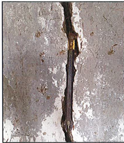
Photo 16: Major vertical full depth cracks
