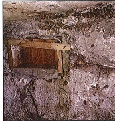
Photo 26: Foundation wall in poor deteriorate state.
