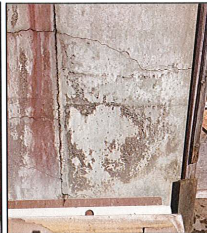
Photo 20: Vertical and horizontal cracks + honey combing on wall
