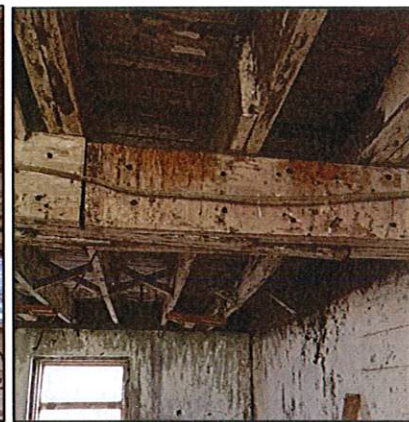
Photo 11: Missing beam and improper splice
