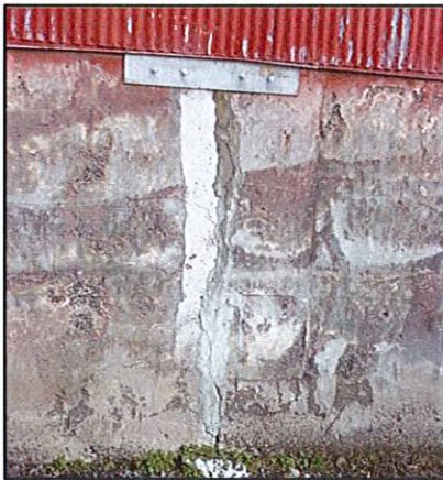
Photo 21: Repairs attempt with bearing angles and repair mortar
