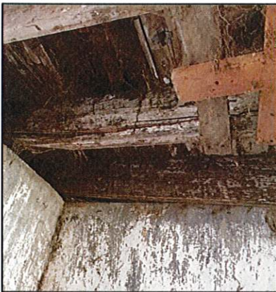
Photo 9: Typical broken joist
