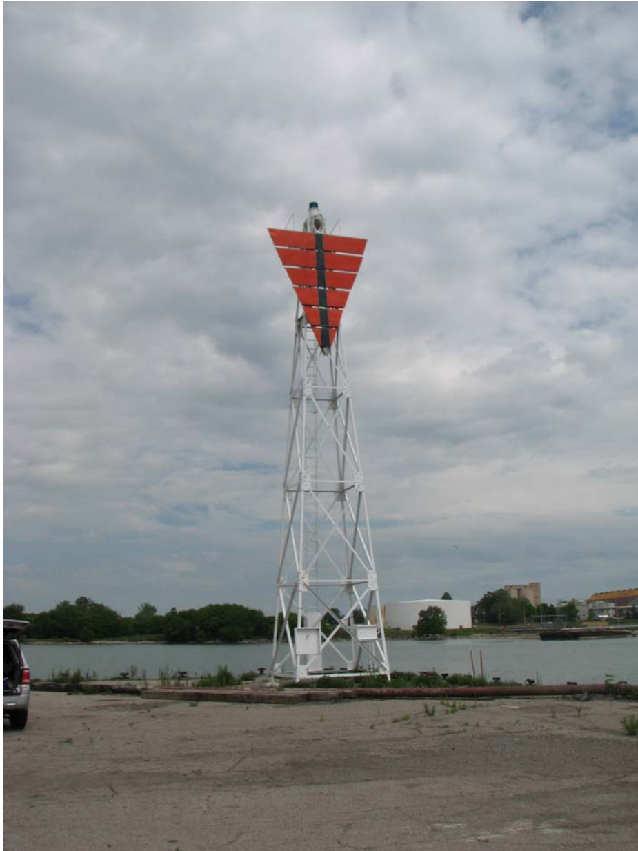
Figure 5: Existing Tower to be Demolished
