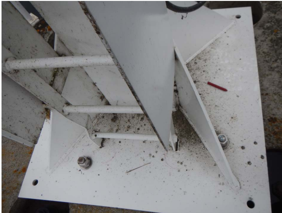
Existing tower anchors
