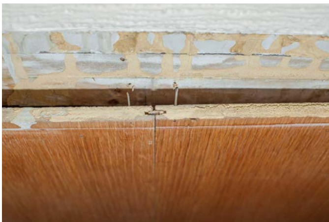
Figure 39: Splined edge joint of panels and attachment to wall by face-nailing (chair rail removed).
