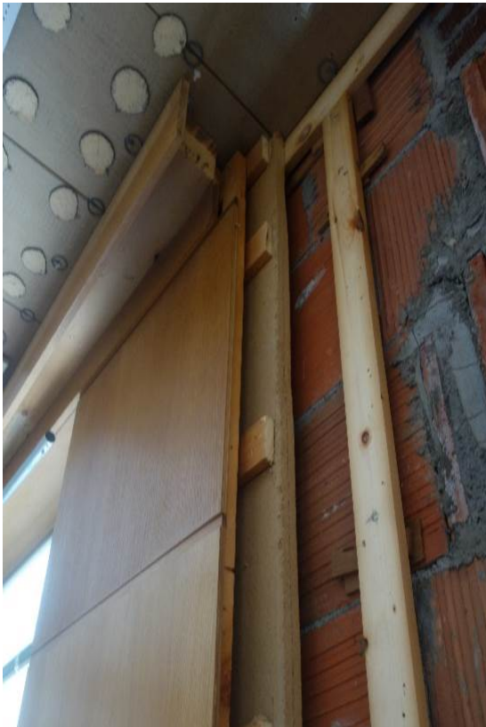
Figure 34: Cross-section of wall and window blind pocket assembly (wood cornice removed) (Photo: Heritage Conservation Directorate, 2016).
