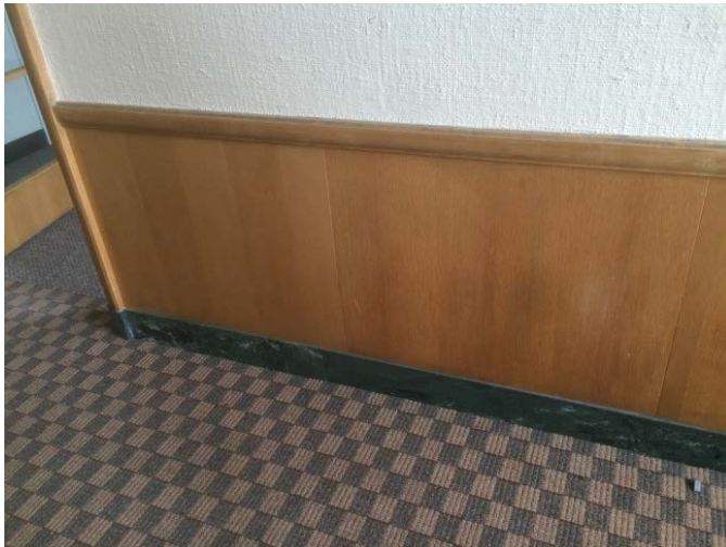
Figure 38: Example of wood wainscoting and chair rail (Room 5014).
