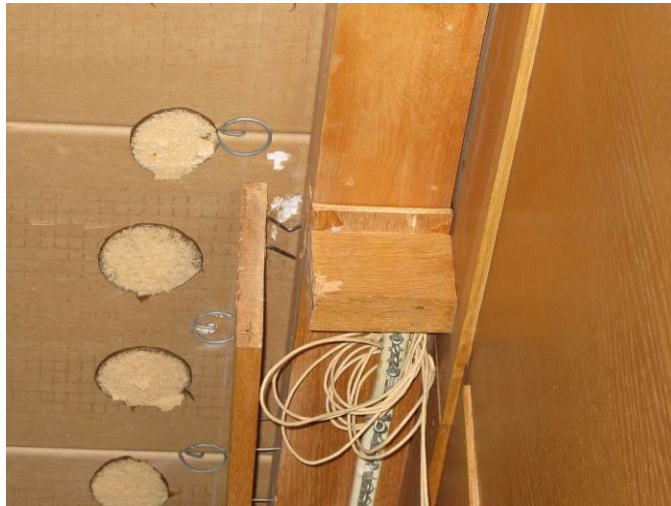
Figure 37: Cross section of window blind pocket assembly. Note: cornice removed and front face partially pried away. (photo: Heritage Conservation Directorate, 2016)
