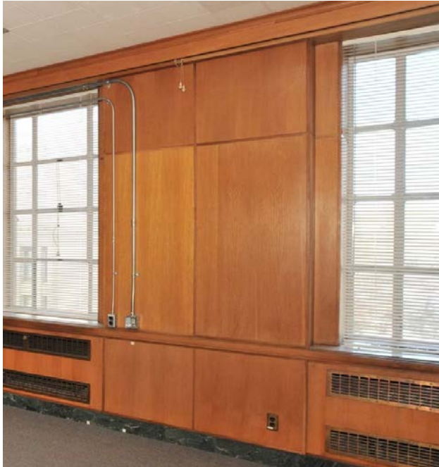
Figure 33: Full wall height wood panelling on interior face of the exterior wall with windows. (Photo: Heritage Conservation Directorate, 2016)
