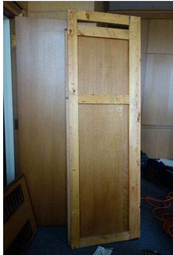
Figure 35: Rear of upper panel (removed) showing backing frame.
