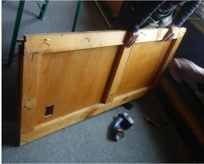
Figure 36: Rear of lower panel (removed) showing backing frame.
