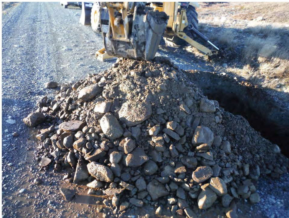
Test Pit TP-10 Spoil Pile
