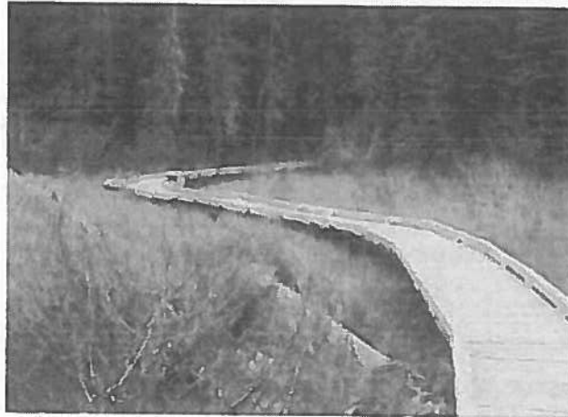
Figure 4.1 Wood treated with waterborne preservatives is often used for decking, such as in this wetland boardwalk (Lebow and Tippie, 2001).
