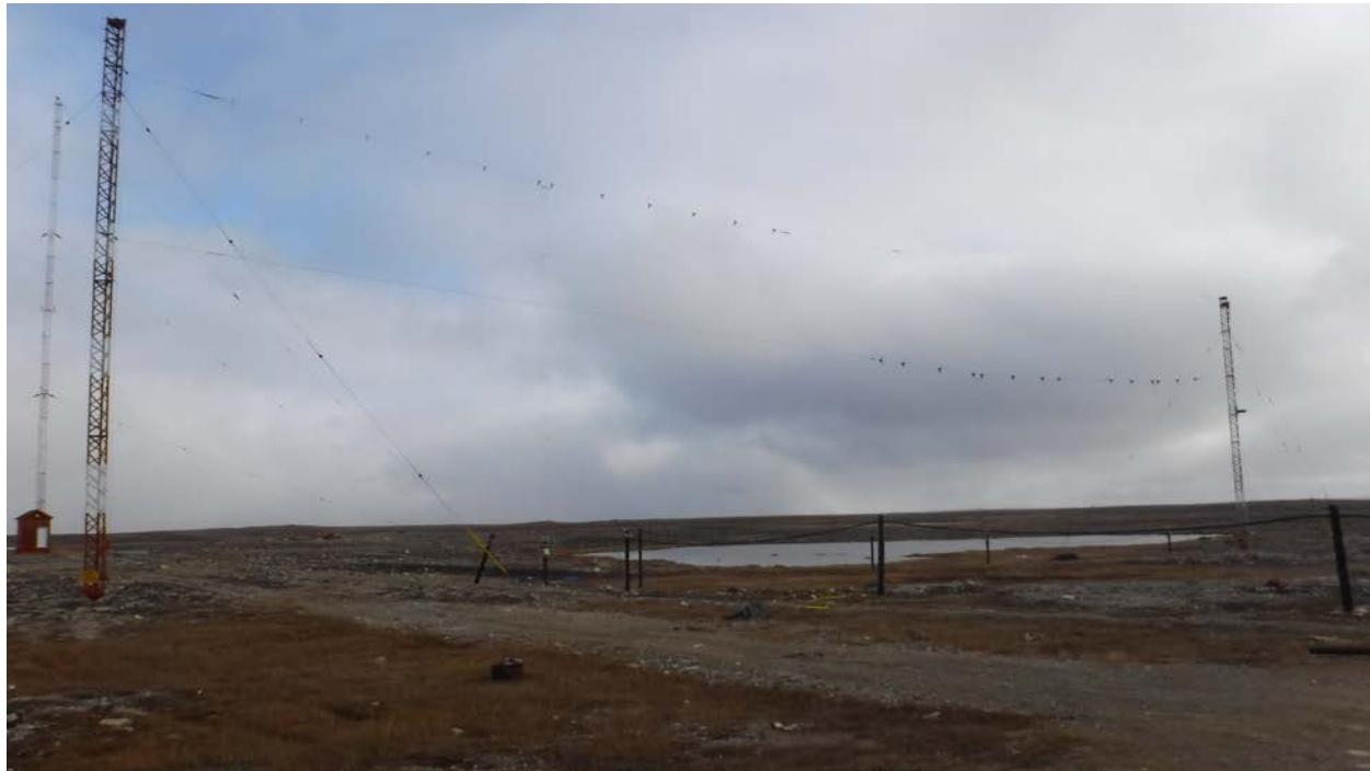
Figure 4: M6 and M10 towers to be replaced
