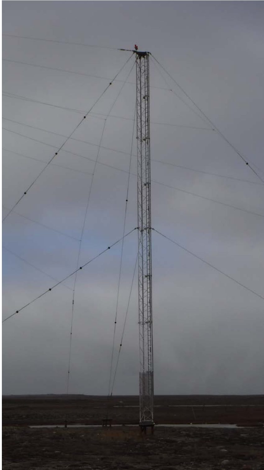
Figure 9: North Tower - RX Site Paint touch up required
