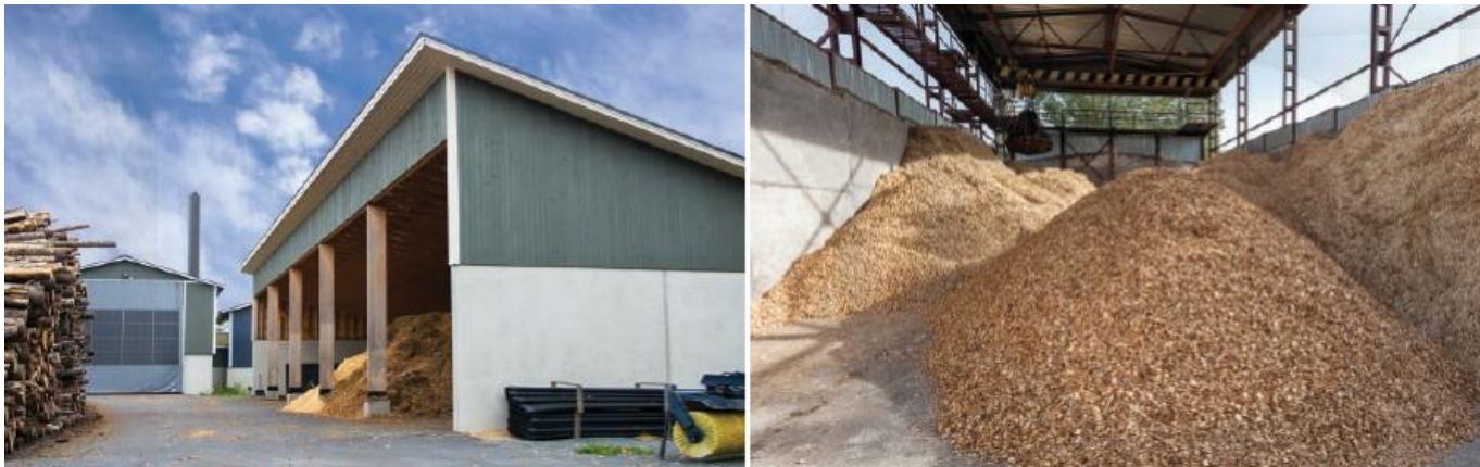
Figure 2. Covered storage for wood chip piles
