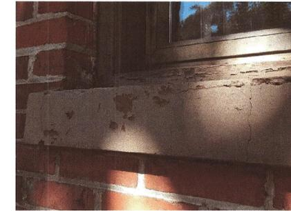
PHOTO 3: EXAMPLE OF DAMAGE TO EXISTING CONCRETE SILL
