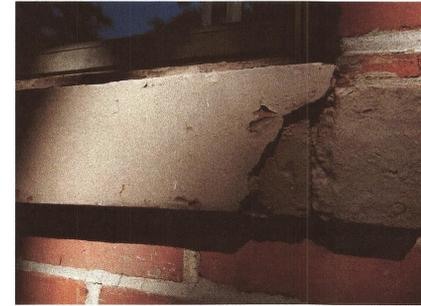
PHOTO 2: EXAMPLE OF DAMAGE TO EXISTING CONCRETE SILL
