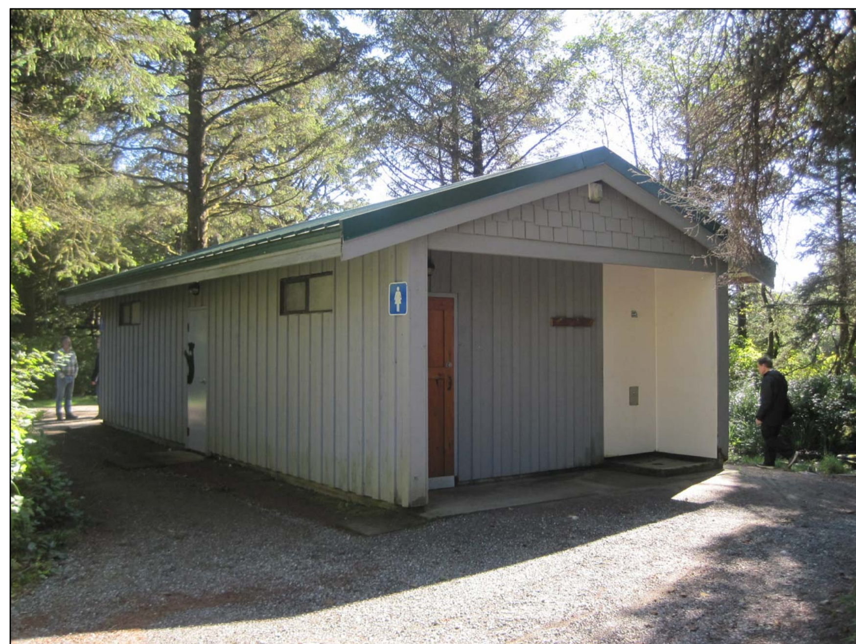
EXISTING LONG BEACH SOUTH (TO BE DEMOLISHED)
