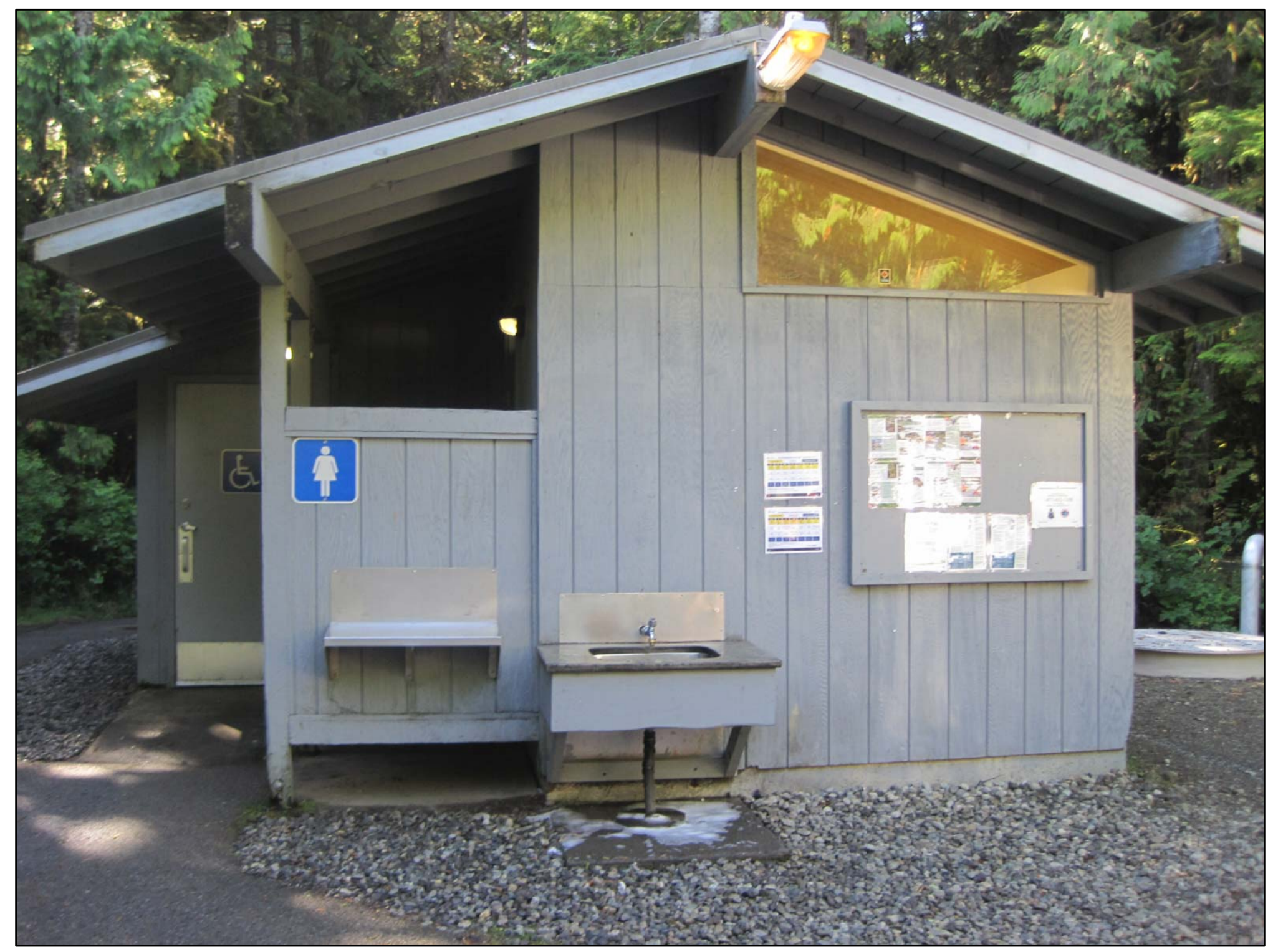
EXISTING GREEN POINT WASHROOM #1 (TO BE DEMOLISHED)
