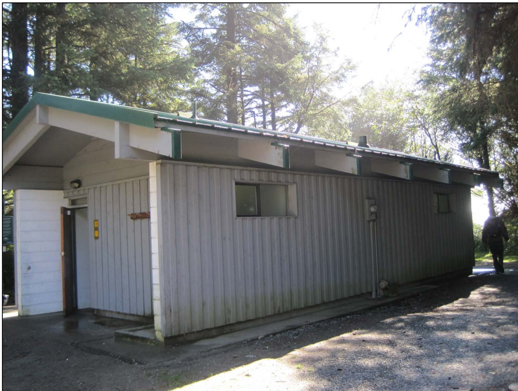
EXISTING LONG BEACH NORTH (TO BE DEMOLISHED)
