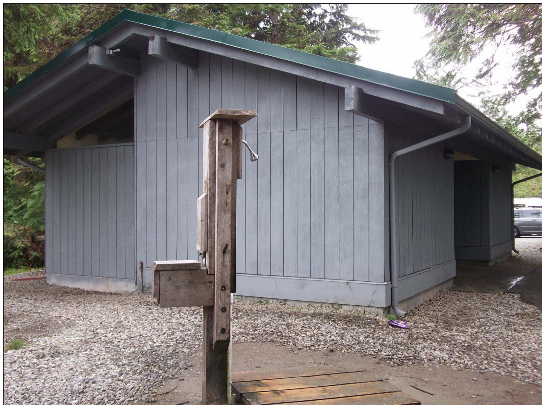
EXISTING WICKANINNISH BEACH WASHROOM ( TO BE DEMOLISHED)
