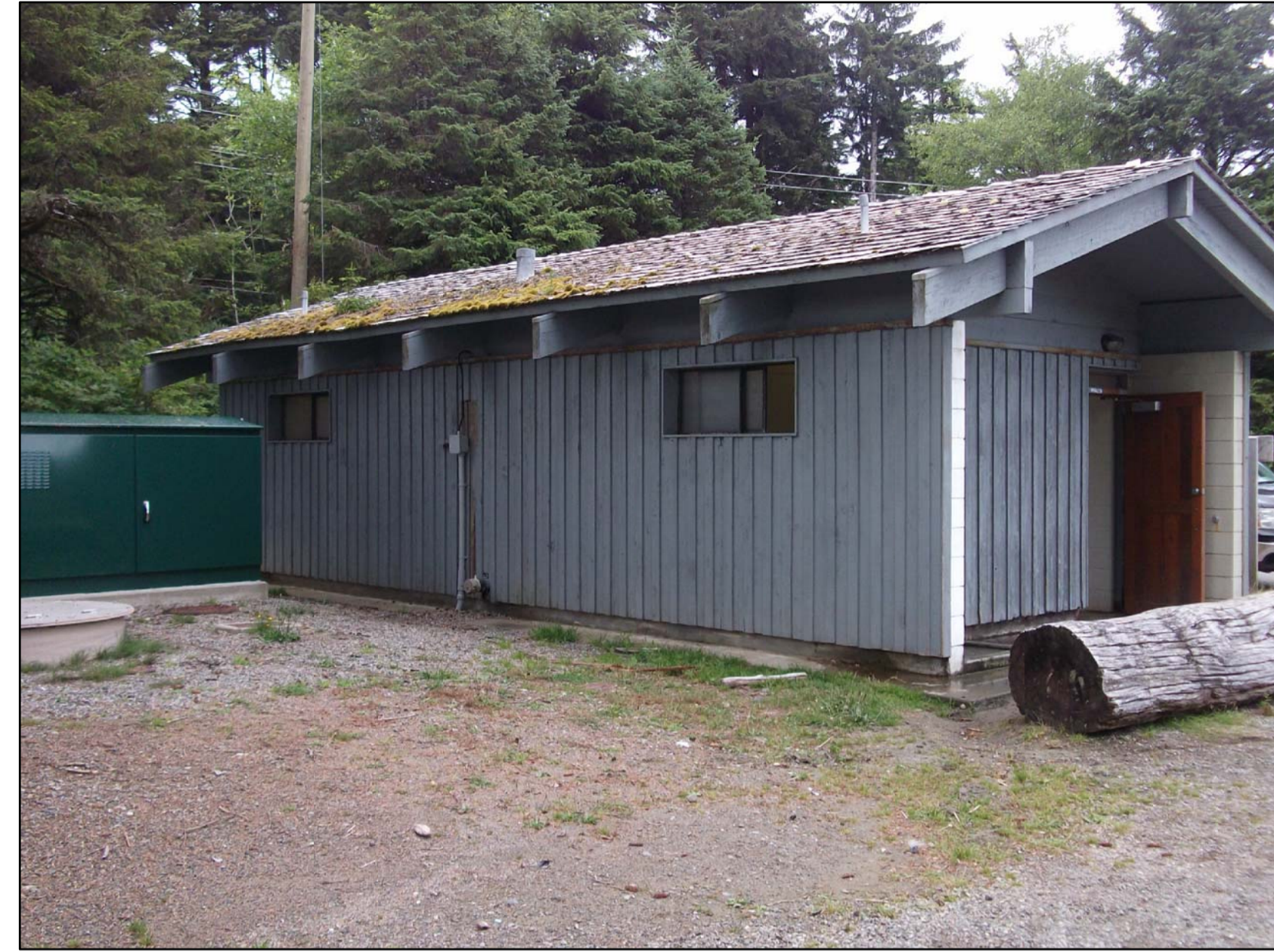
EXISTING INCINERATOR ROCK WASHROOM (TO BE DEMOLISHED)
