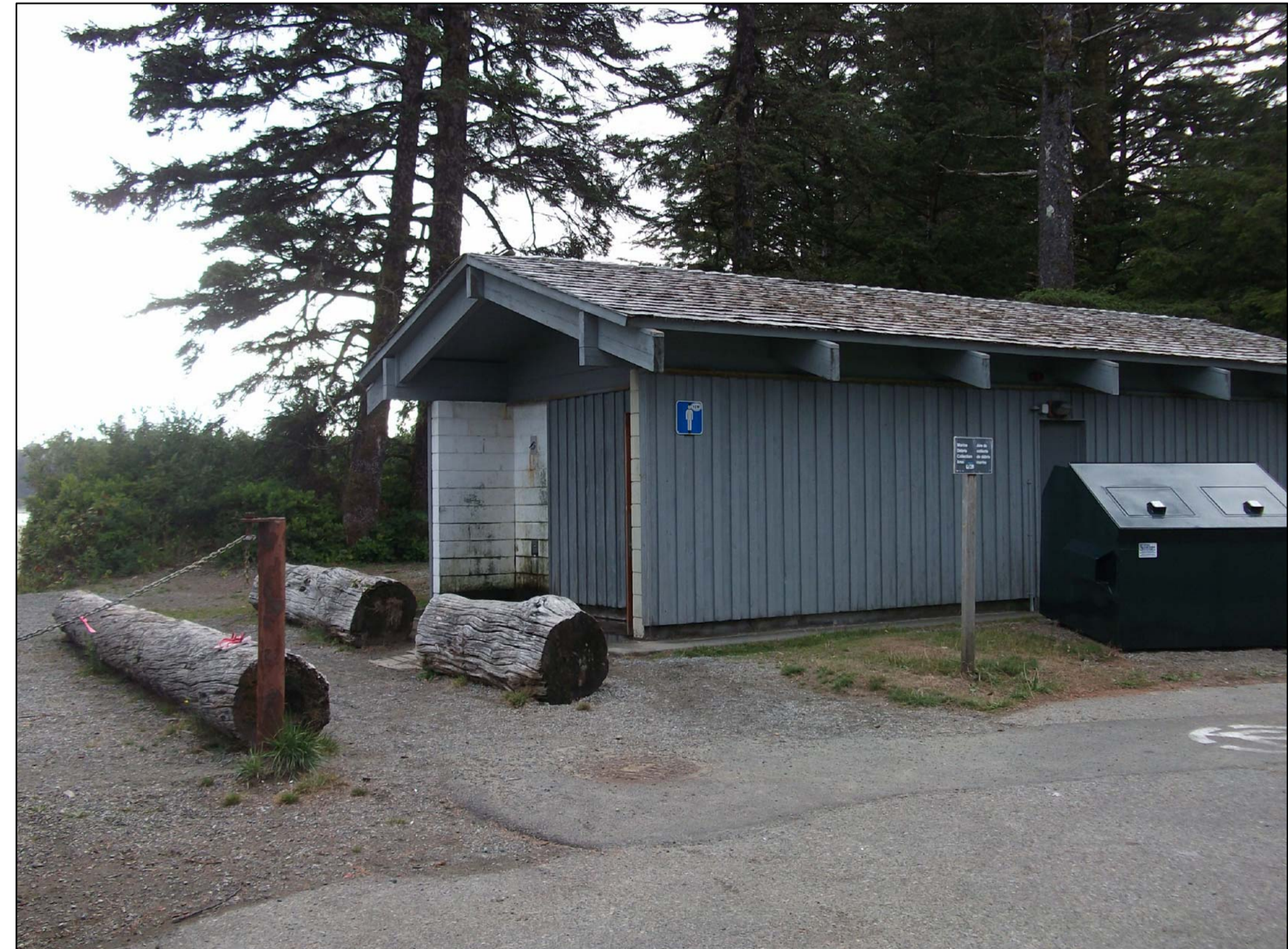
EXISTING INCINERATOR ROCK WASHROOM (TO BE DEMOLISHED)
