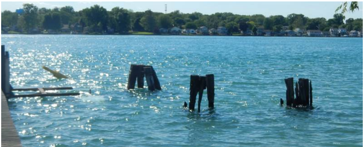
Figure 2: Existing abandoned dolphin foundations (not to be removed unless required)
