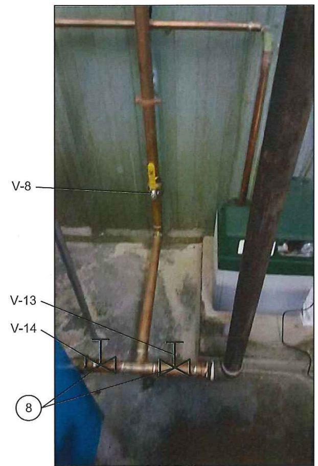
03 DETAIL 2 RETURN LINES M2.3 SCALE: NTS
