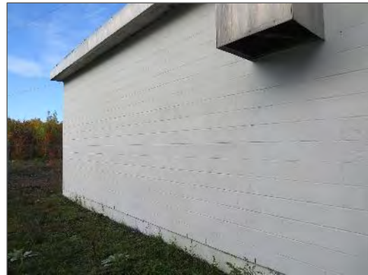
Photo 9: White on concrete block, insignificant lead concentration.
