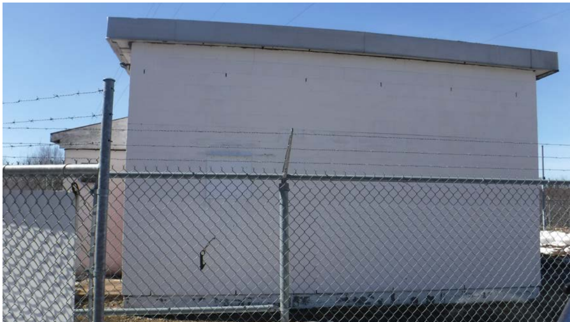
Figure 4: Old radio equipment building facing [North] (to be demolished)
