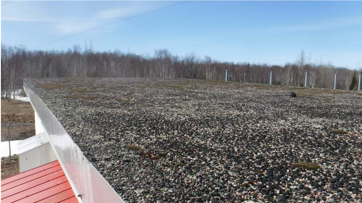
Figure 10: Gravel on Built-up roof (to be demolished)
