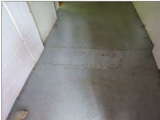
Photo 8: Grey paint on concrete floor, insignificant lead concentration.
