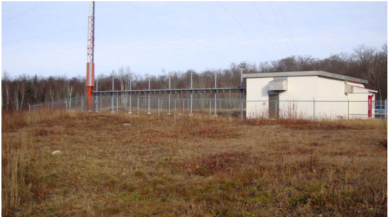
Figure 17: Waveguide Bridge to be demolished. There are 7 posts, the post adjacent to the tower is not to be demolished. New building is not shown in this picture.
