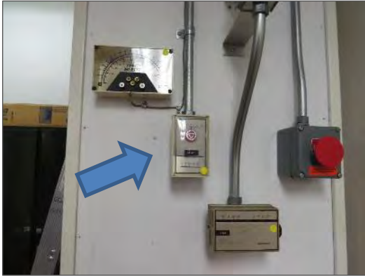
Photo 12: Mercury-containing thermostat.
