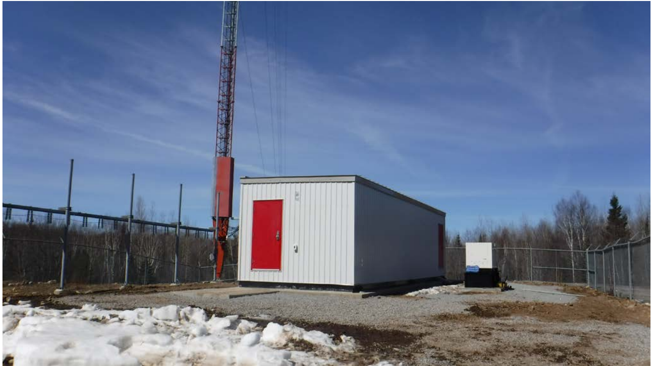
Figure 20: New equipment building ( not to be demolished ). Stair systems to be installed in front of red doors. Waveguide bridge to the left of the building is to be demolished.
