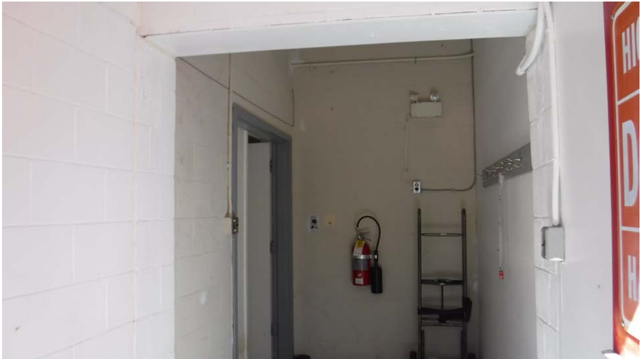
Figure 8: Old equipment interior (to be demolished)
