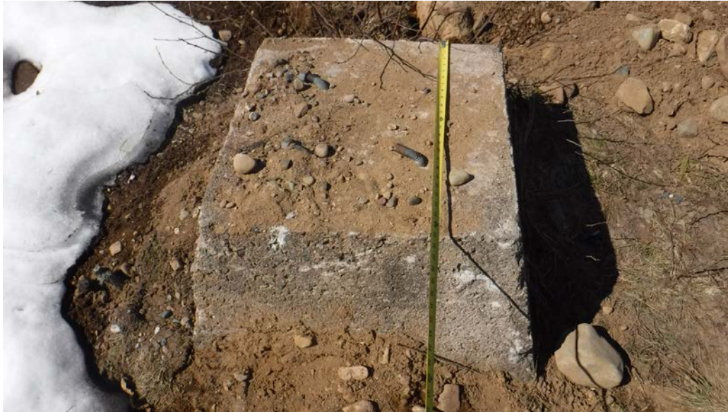
Figure 12: Abandoned concrete anchor (to be demolished)
