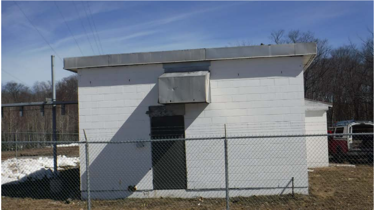
Figure 5: Old equipment building [South] (to be demolished)
