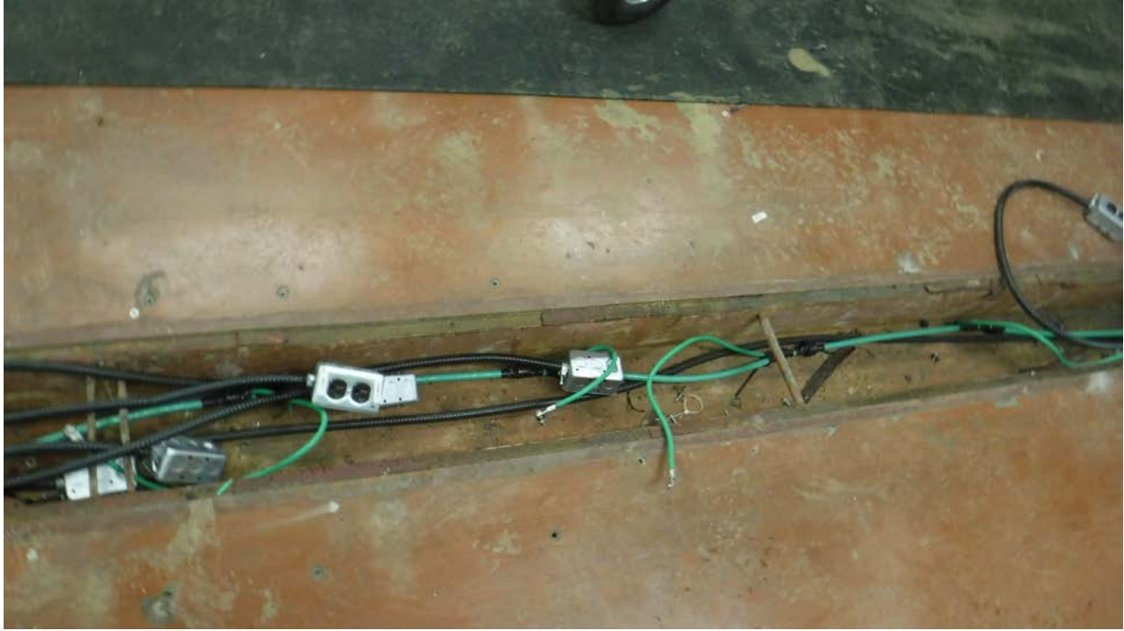
Figure 7: Typical cable troughs (to be demolished)
