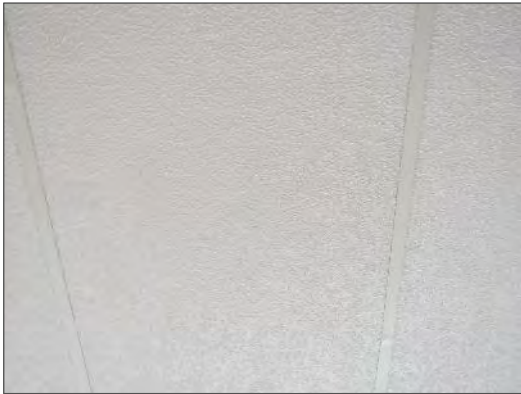
Photo 2: 2' x 4' fibreglass lay-in ceiling tile, does not contain asbestos.
