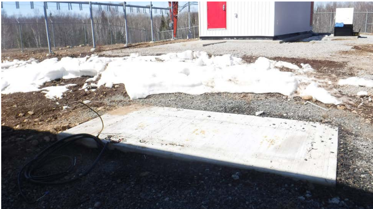
Figure 13: Abandoned diesel generator foundation slab (to be demolished) [bottom of picture].
