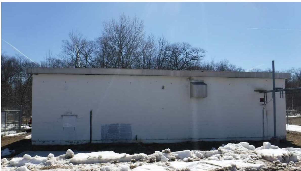
Figure 2: Old radio equipment building [West] (to be demolished)
