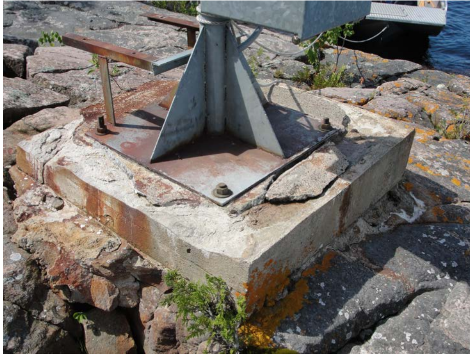
Figure 11: Existing LL1432 Three Pine Island). Foundation to be demolished.
