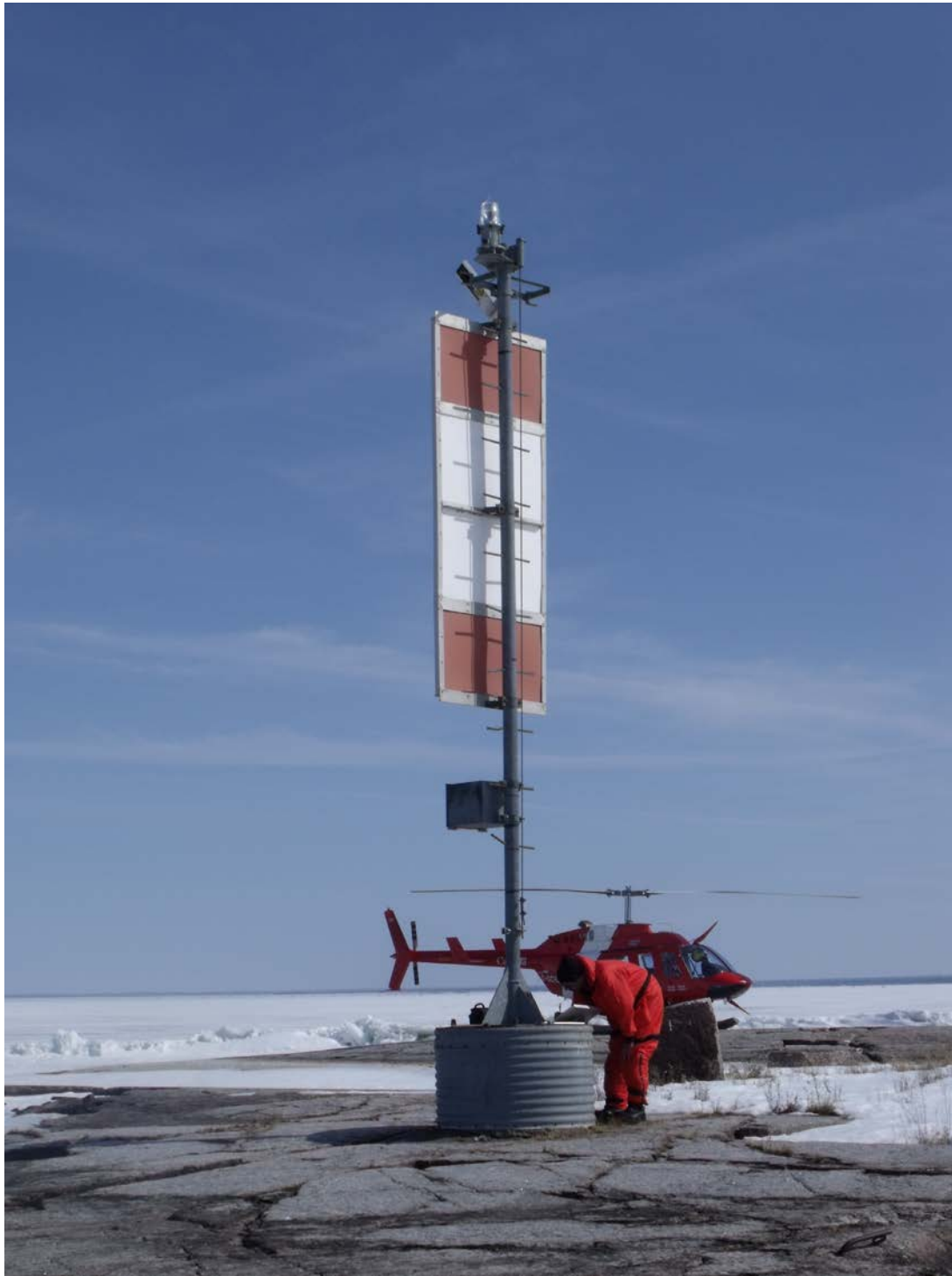
Figure 15: Existing LL1427 Gull Rock. Foundation not to be demolished.
