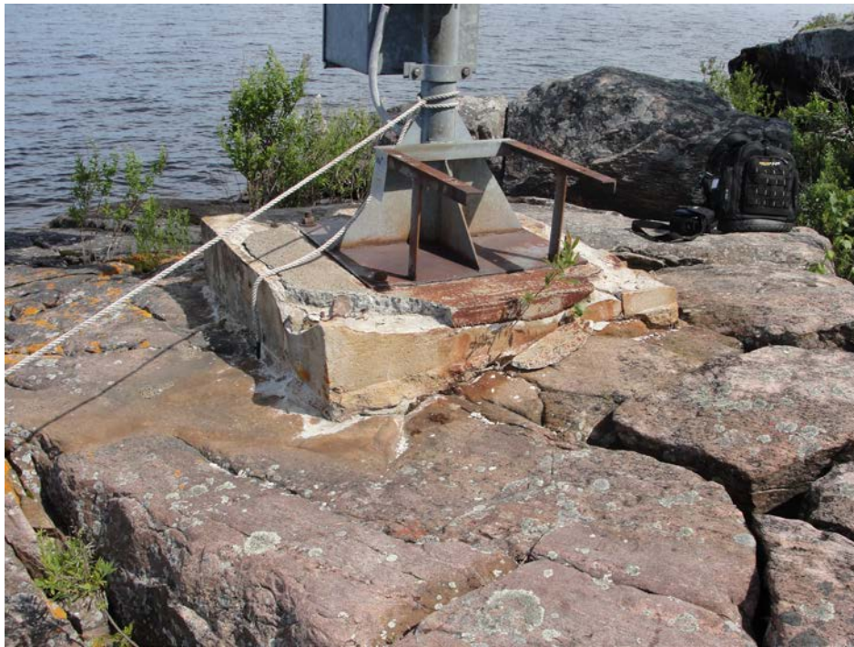
Figure 12: Existing LL1432 Three Pine Island. Foundation to be demolished.
