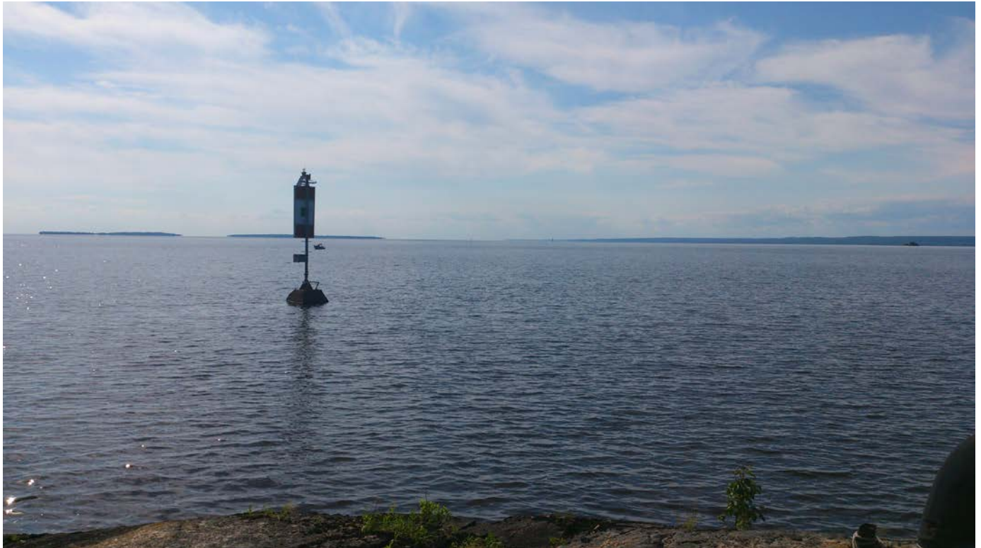
Figure 2: Existing LL1420.8 La Vase River Entrance as seen from shore (to be removed)
