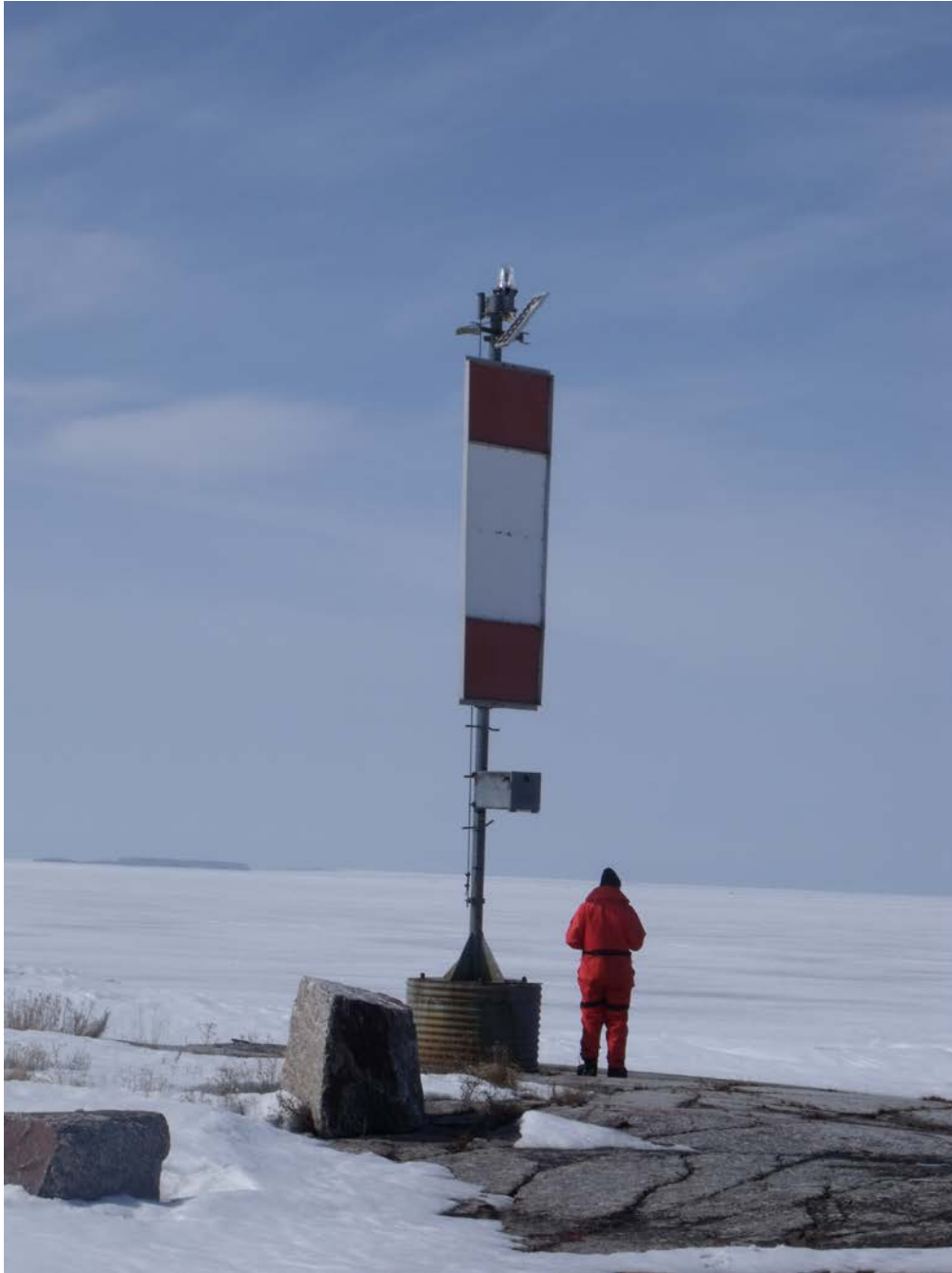
Figure 14: Existing LL1427 Gull Rock. Foundation not to be demolished.
