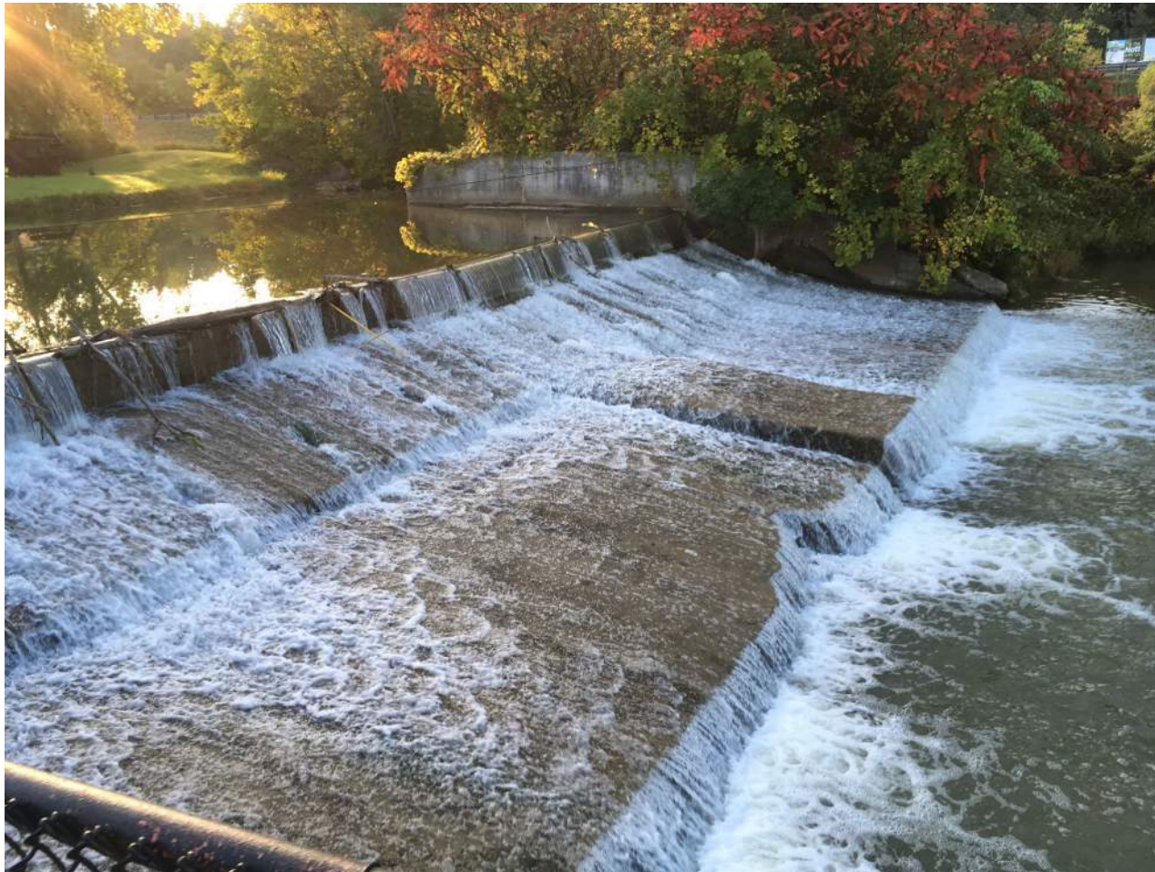
PHOTO 1 Location: North Dam
