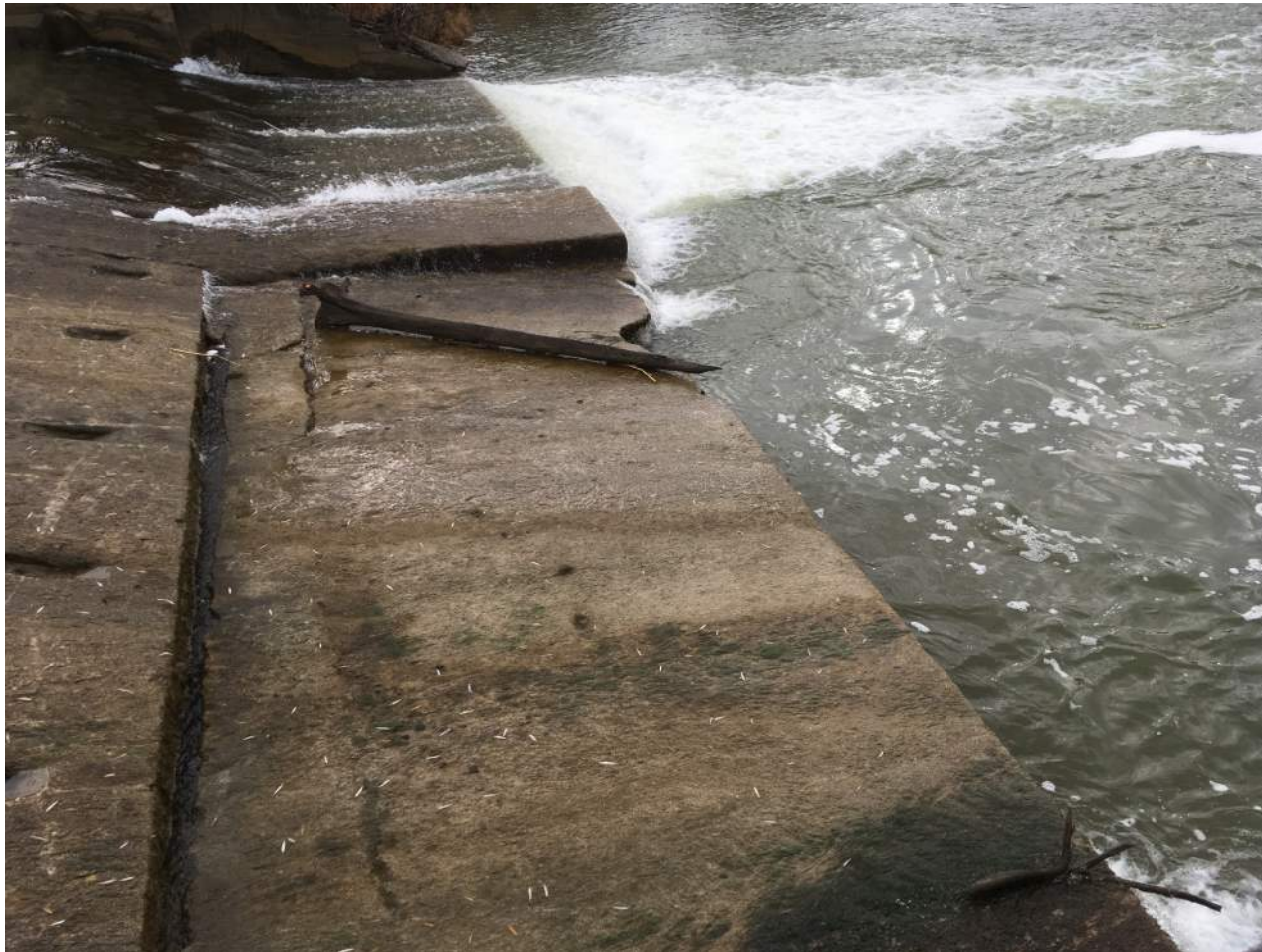
PHOTO 4 Location: North Dam
