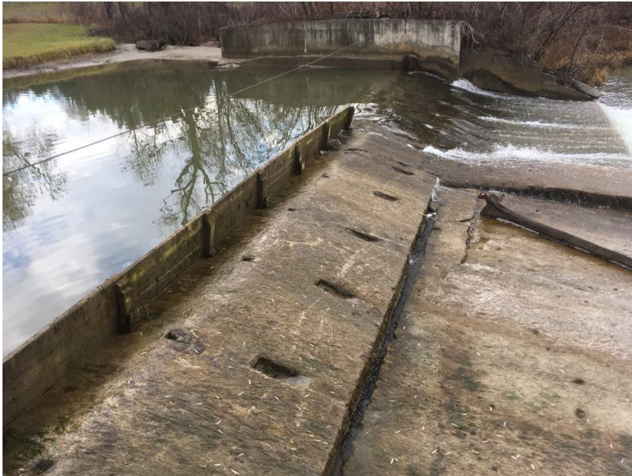
PHOTO 3 Location: North Dam
