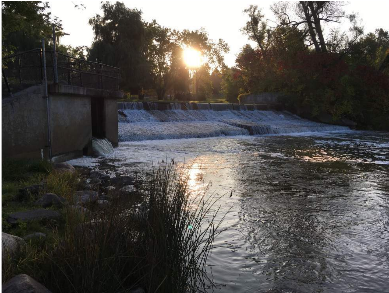
PHOTO 2 Location: North Dam
