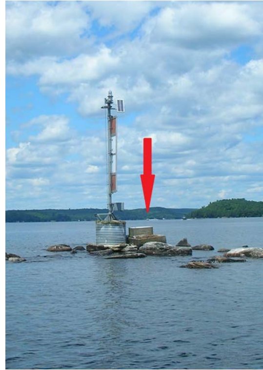
Figure 4: LL1415 Gull Rocks Note abandoned foundation to be removed
