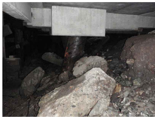
PHOTO C17-07 FORESHORE RIPRAP DIRECTLY UNDER STEEL PILED CONCRETE DECK
