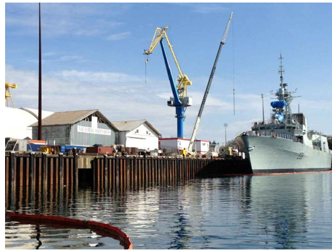
PHOTO C14-01 SOUTH JETTY SHEET PILE WALL - NOTE SMALL BOAT ACCESS OPENING
