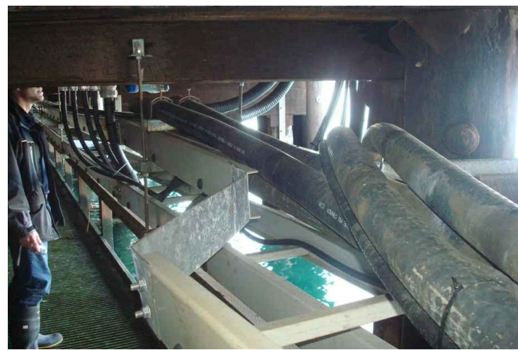
PHOTO C16-07 UNDER-PIER CATWALK AT KIOSK LOCATION - LOOKING EAST
