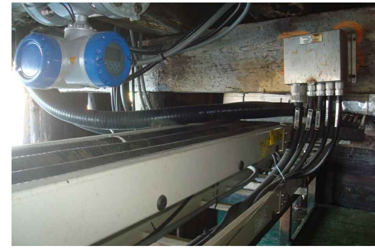
PHOTO C16-05 UNDER-PIER CATWALK AT KIOSK LOCATION - LOOKING WEST
