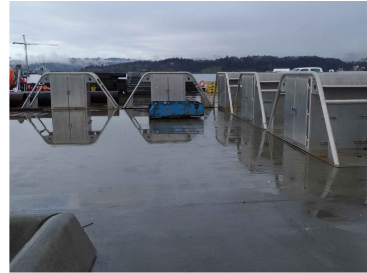
PHOTO C47-03 REMOVED MECHANICAL KIOSKS
