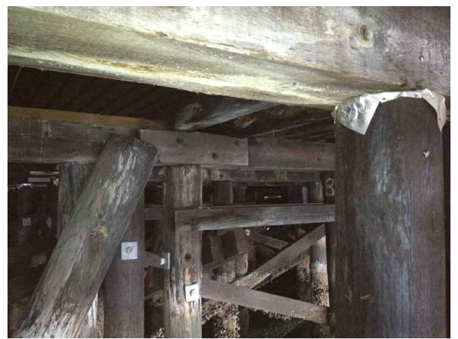
PHOTO C15-07 TIMBER PILED JETTY – TYPICAL VIEW UNDER WEST CRANE PAD
