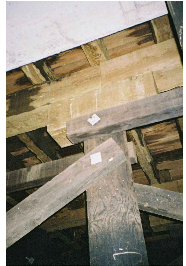
PHOTO C15-08 TIMBER INFILL DECK CONSTRUCTION – NOTE CONDITION OF TIMBER AT THIS STRUCTURE
