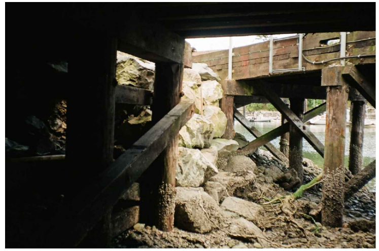
PHOTO C15-01 TIMBER PILED JETTY AT EAST APPROACH – NOTE RIPRAP FORESHORE SLOPE
