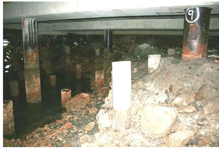
PHOTO C17-04 FORESHORE FILL MOUND UNDER STEEL PILED CRANE PAD – LOOKING WEST
