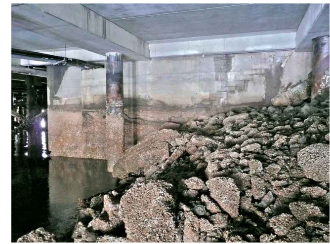
PHOTO C17-06 SOUTH FACE OF TIMBER CRIB AND RIPRAP FORESHORE SLOPE
