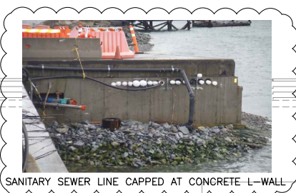
SANITARY SEWER LINE CAPPED AT CONCRETE L-WALL
