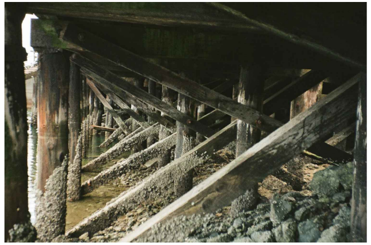
PHOTO C15-02 TIMBER PILED JETTY – TYPICAL VIEW AT EAST APPROACH JETTY LOOKING WEST
