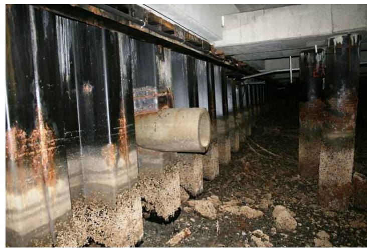
PHOTO C14-08 STORMWATER OUTFALL AT SHEET PILE BULKHEAD
