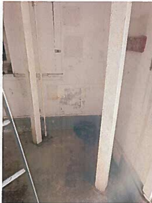
Photo 22 – Angle Columns and Tie-rods
