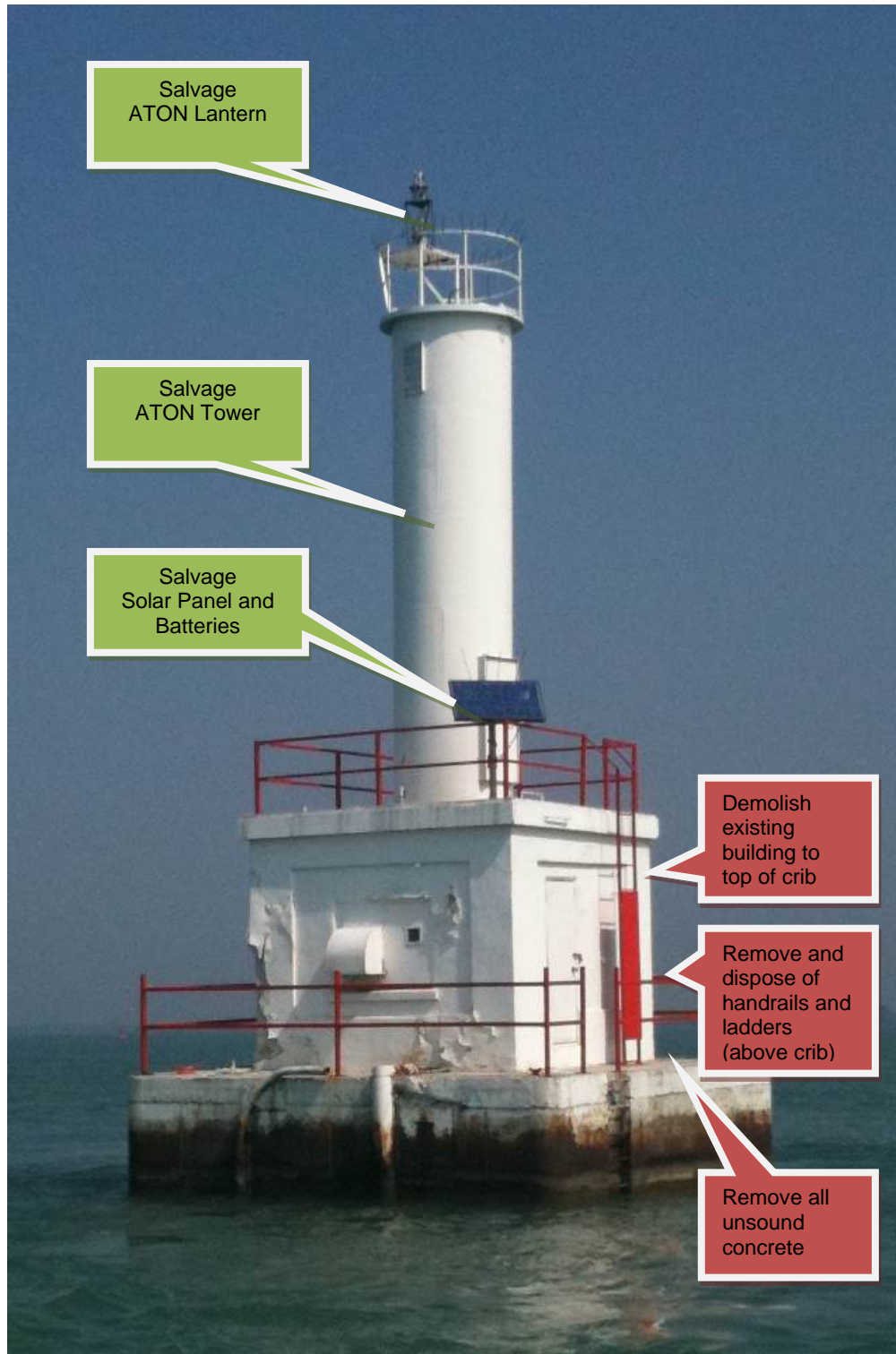
Existing conditions and expected action Additional photos are provided in Appendix B4
