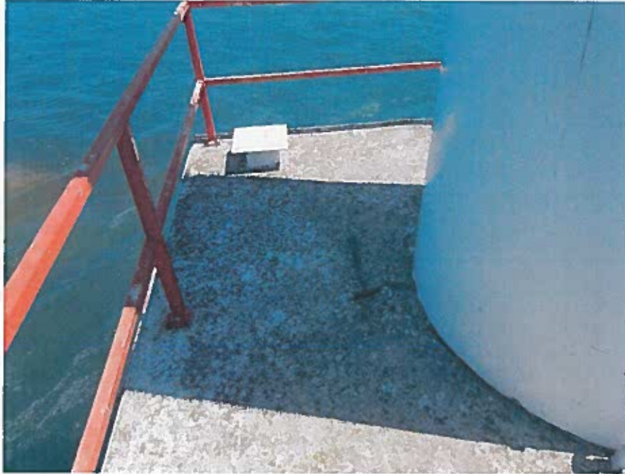
Photo 25 – Typical Building Roof
