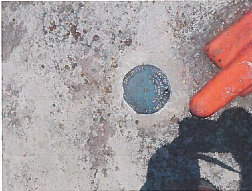
Photo 27 – Survey Monument at North Corner of Crib Cap
