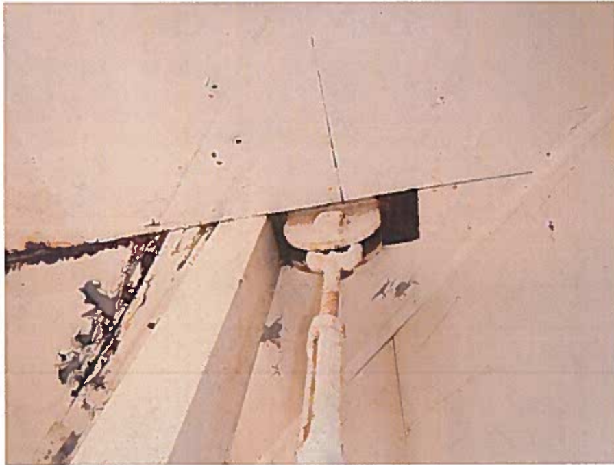
Photo 23 – Typical Angle Column and Tie-rod Connection at Ceiling
