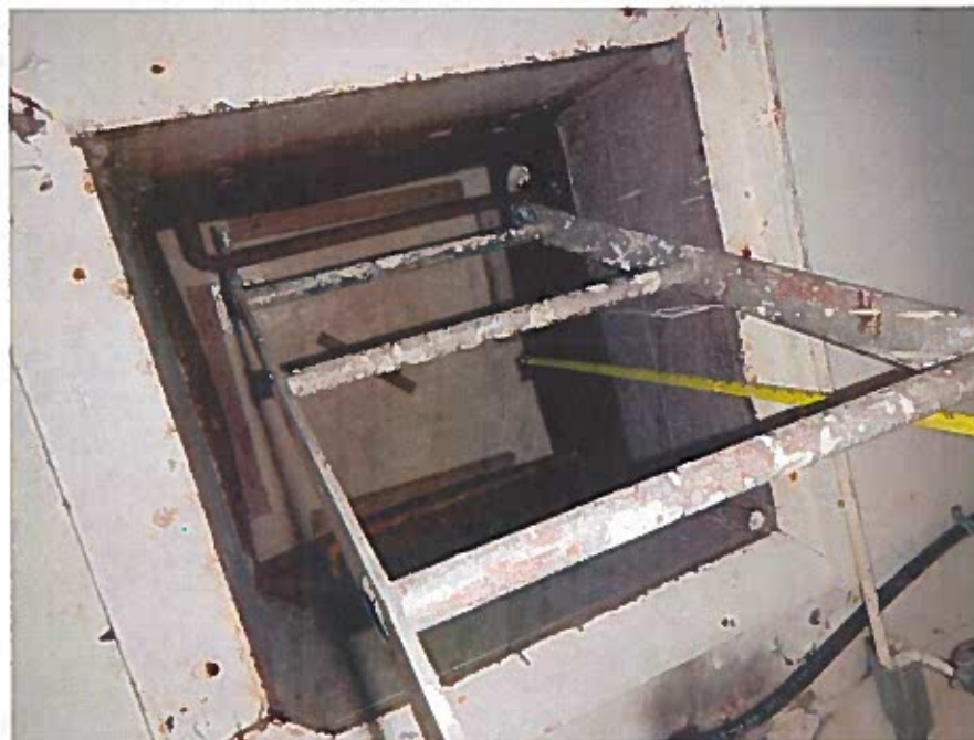
Photo 28 – Roof Hatch to Access Tower
