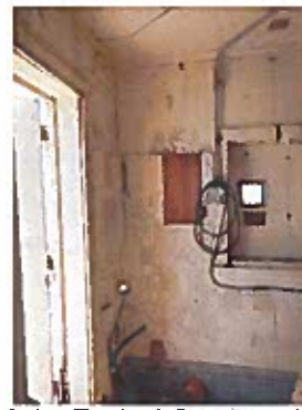
Photo 2.4 – Typical Condition Inside of Building
