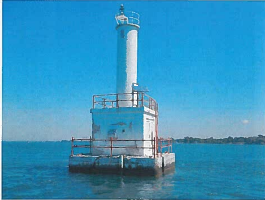
Photo 1 – LL 677 Livingstone Channel Aid Tower
