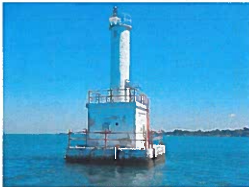
Photo 2.1 – Overview of Structure
