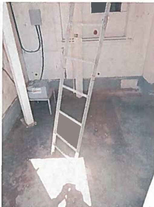
Photo 17 – Crib Cap / Floor of Building
