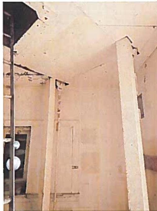
Photo 20 – Northeast Wall and Ceiling
