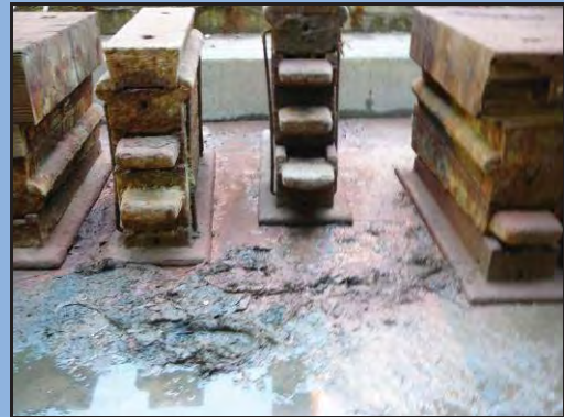
Sediment from the harbour often settles on dock bottom after dewatering. This may become contaminated with paint, etc. and must be disposed of.
