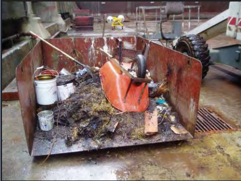
Store all waste grit away from drains, to prevent contaminated water migrating into the marine environment.
