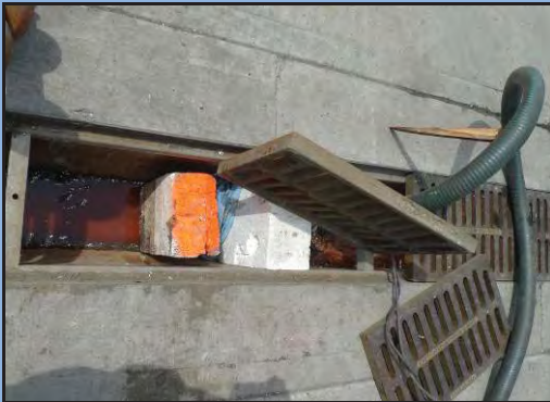
Example of styrofoam blocks used as a drain blocker on the NLW.
