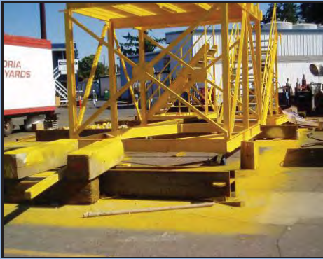
Ensure tarps are in place to prevent overspray impacting the surrounding work area.
