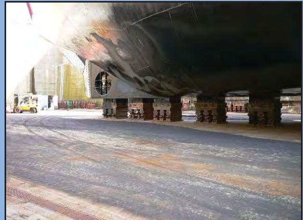
Example of a dock floor that would not pass inspection.
