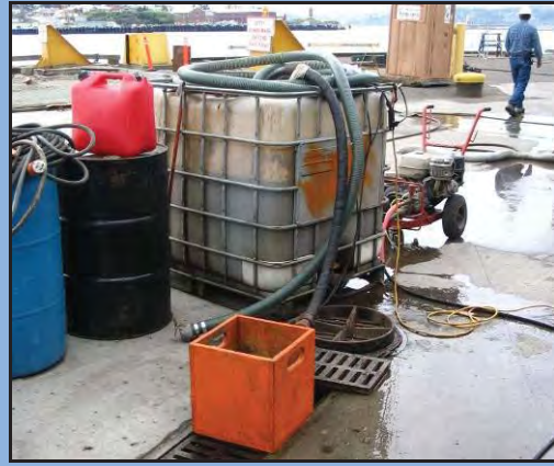
The trench drain is blocked and a sump pump is installed to collect wash water into a tote.
