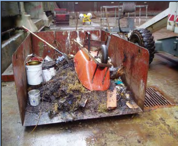
When cleaning dock bottom, skips of waste sandblast grit may leak contaminated water and should be removed as soon as possible.
