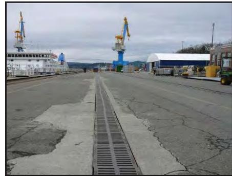
**Fire Holes:** On the South Jetty the fire holes flow directly into the harbour. If any containers fail near the fire holes, the material will not be able to be recovered once it is in the harbour..
