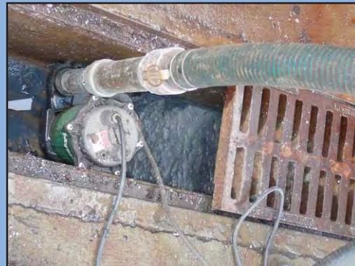
Example of a pump set up used to collect wash water on the NLW.
