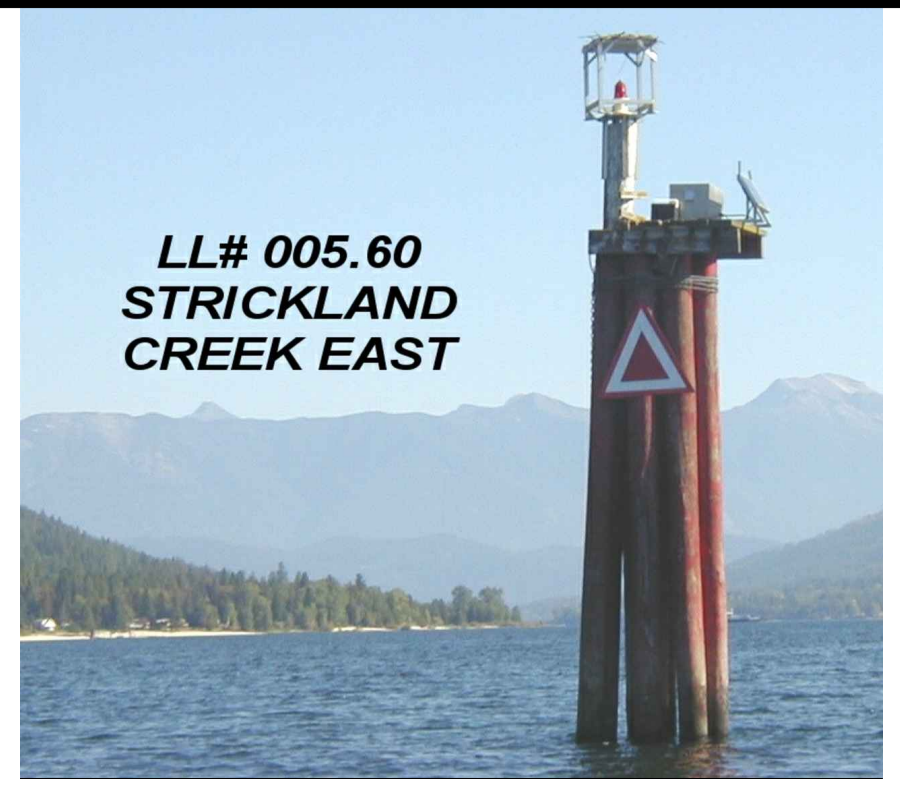
LL 5.6 STRICKLAND CREEK EAST EXISTING STRUCTURE
