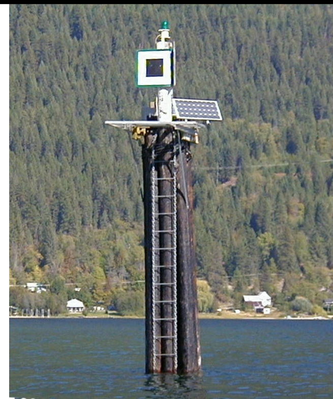
LL 5.3 KOKANEE POINT EAST EXISTING STRUCTURE
