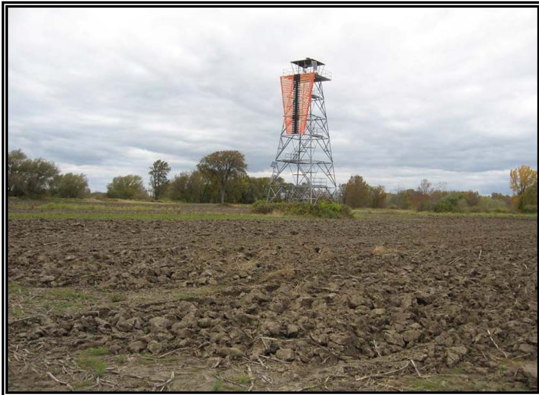
Photograph no. 1: Northbound view of the rear range light (RRL) for navigation on Île Bouchard.
