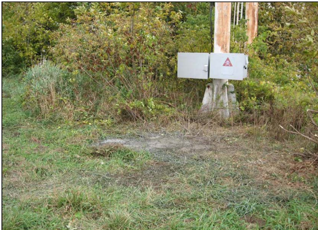
Photograph no. 4: Status after drilling borehole F-01.
