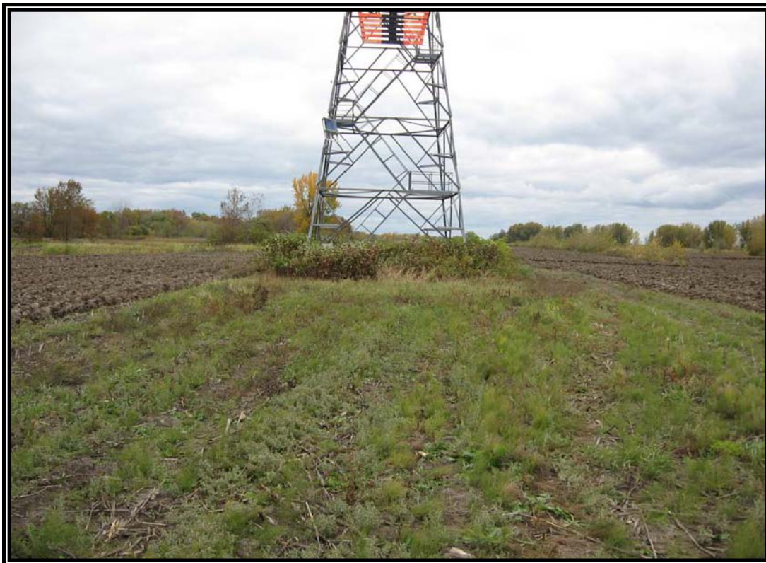
Photograph no. 2: Status prior to drilling borehole F-02.
