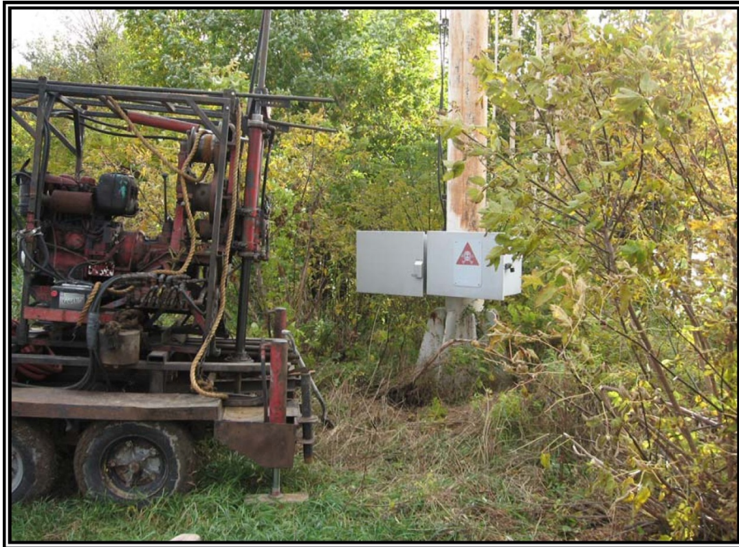
Photograph no. 3: Location of the drilling equipment to make borehole F-01.
