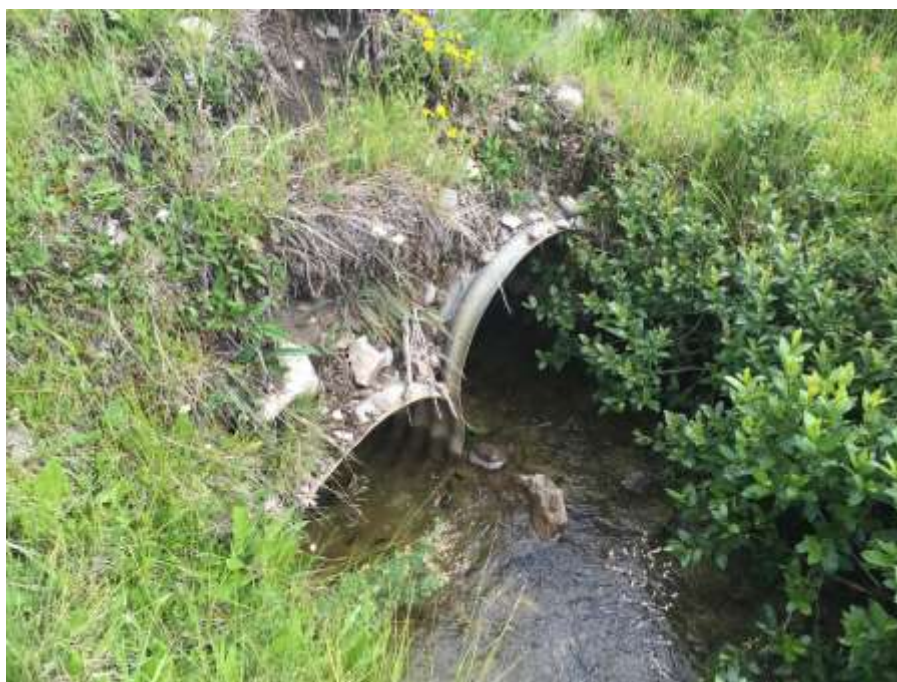
Photo 4 – Double culvert carrying Shelby's Creek under the old road bed/proposed new highland road alignment
