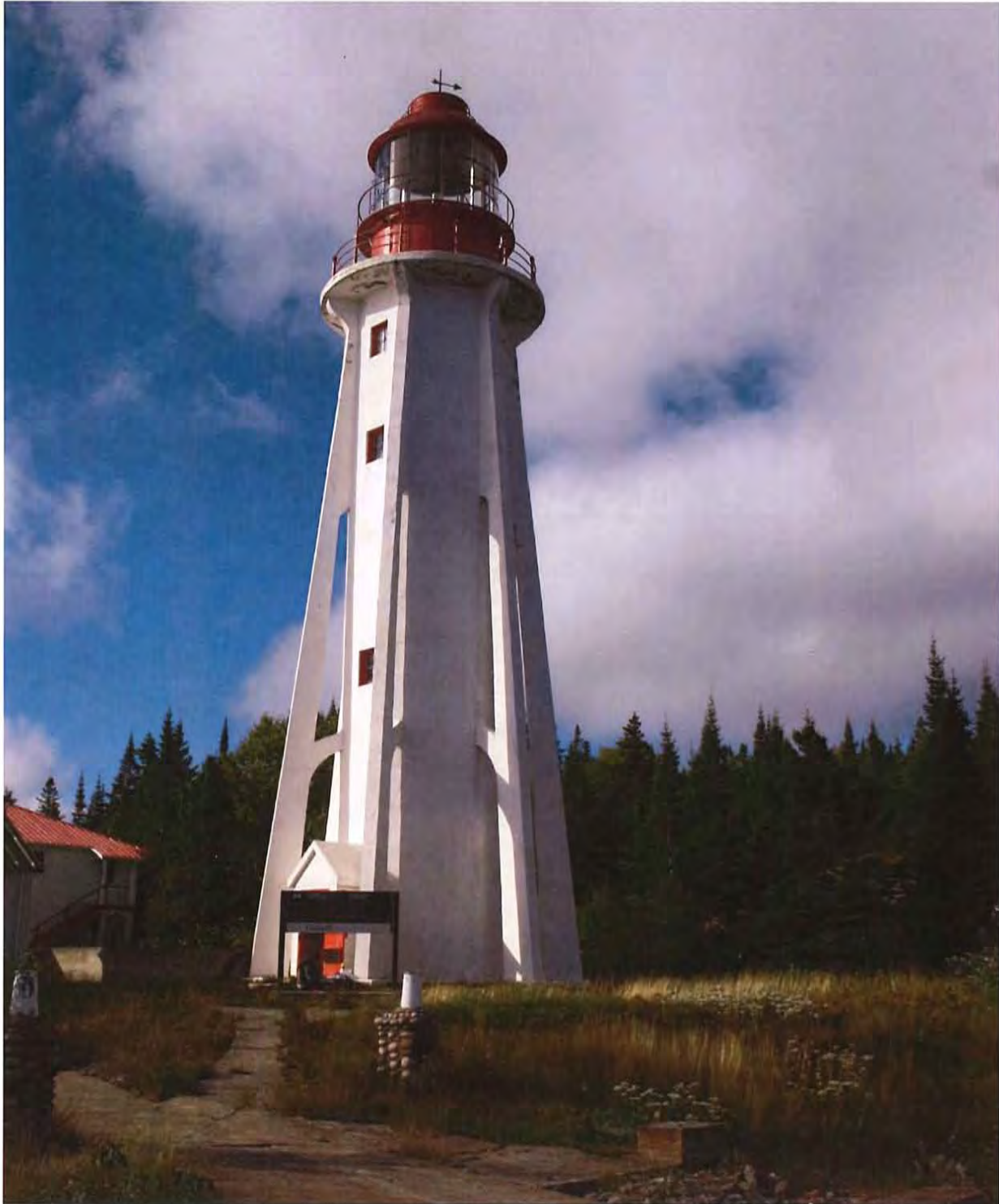
Overall view of Lighthouse. Six flying buttresses. Top floor extends as exterior concrete platform.
