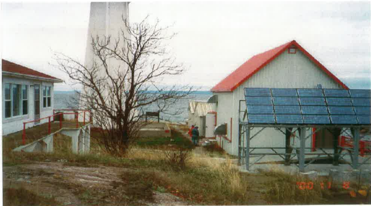
PHOTO 2 SAMPLING LOCATIONS NEAR CONCRETE DYKED TANK FARM, LOOKING NORTH.
