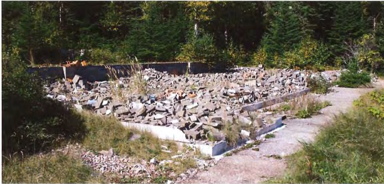
Part-demolished concrete block foundations.
