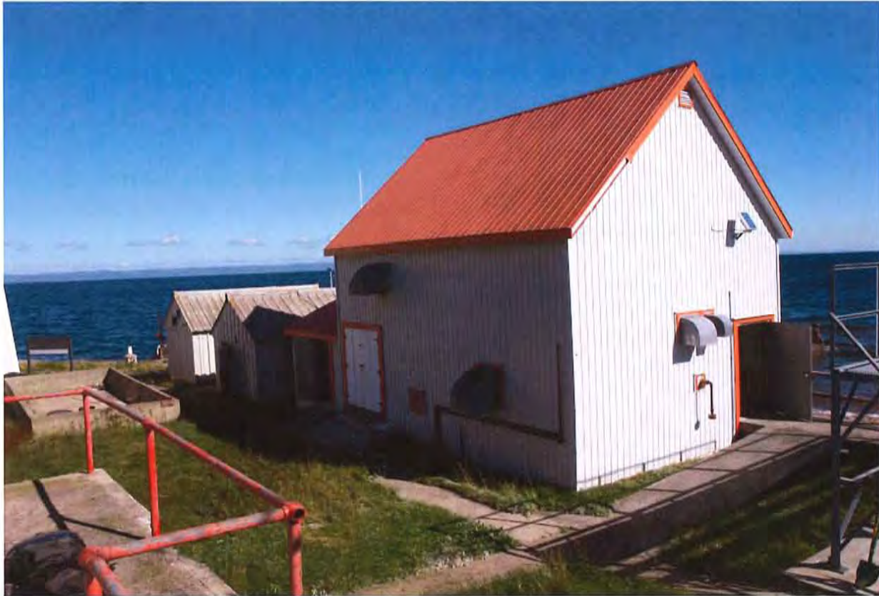
Overall view of generator building, annex in shadow, and two small storage buildings beyond. Metal cladding in good condition, one fascia piece missing.
