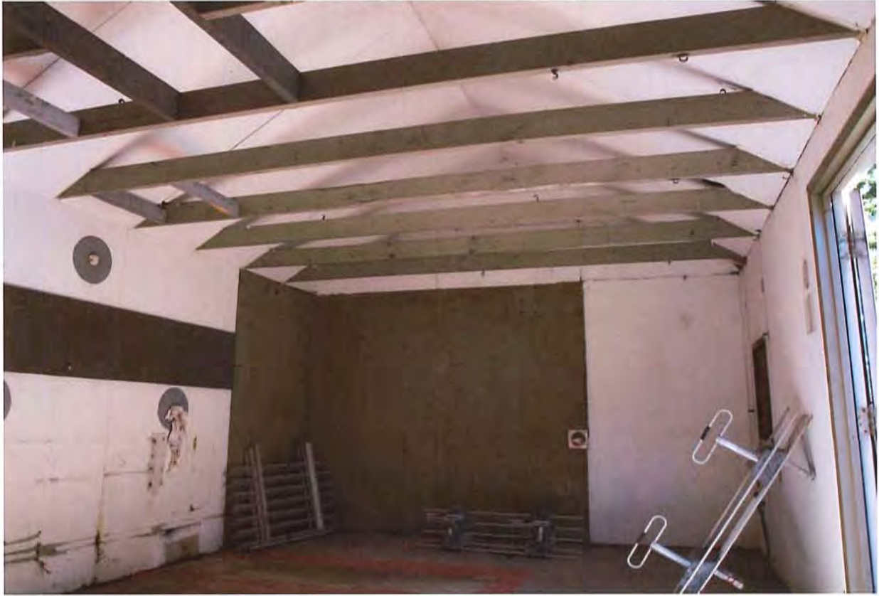
Annex to Generator Building: Interior view.
