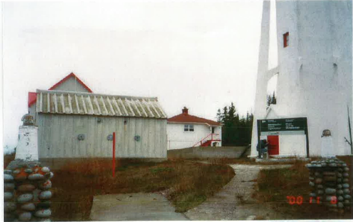
PHOTO 1 MICHIPICOTEN ISLAND, LAKE SUPERIOR. AREA NORTHEAST OF GENERATOR BUILDING, LOOKING SOUTH.
