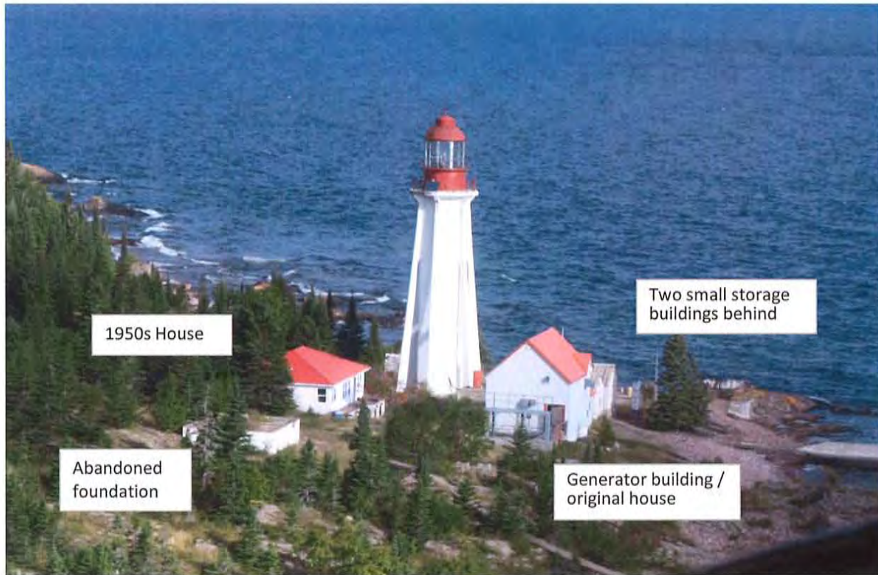
Overall view of Light Station
