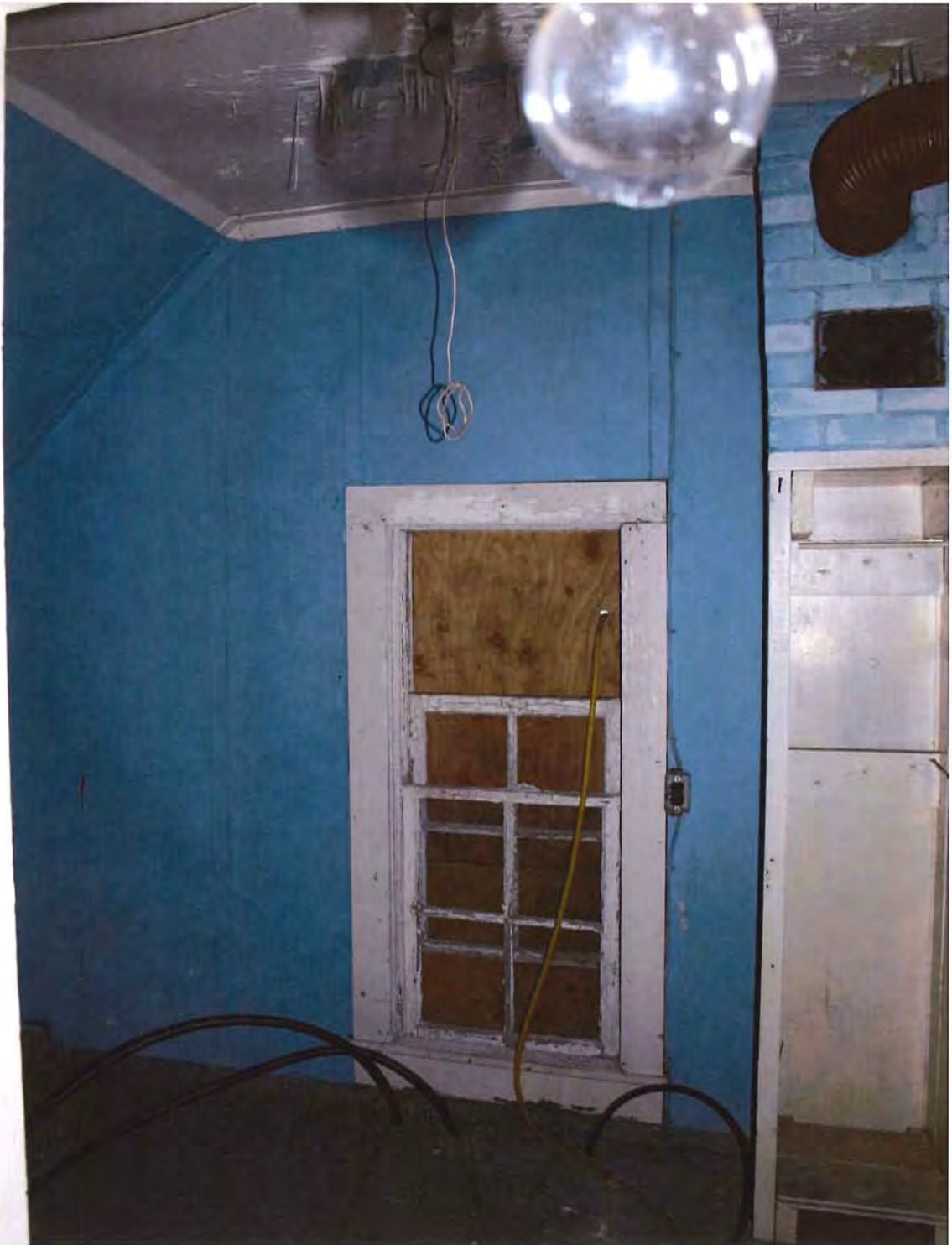
Generator Building: Second floor - boarded-over window, original finishes.
