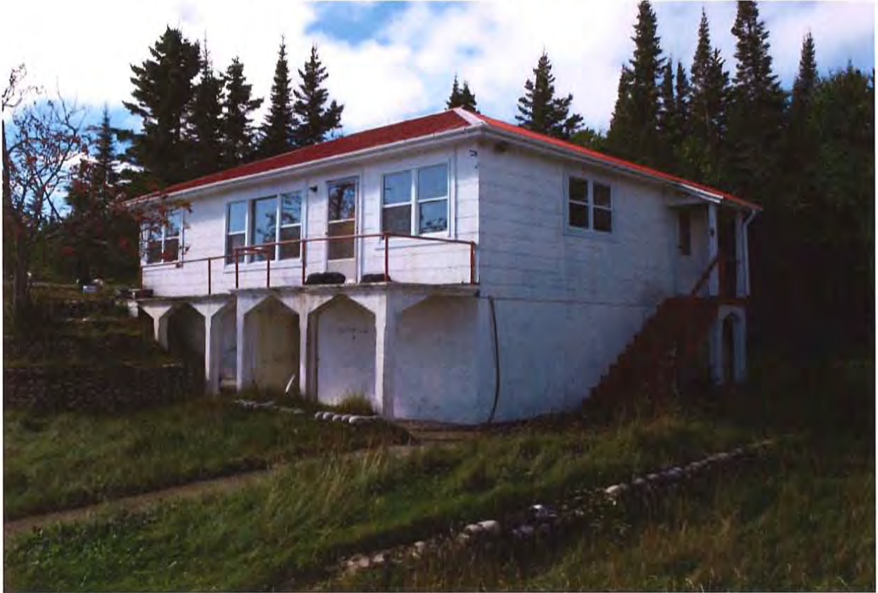
Overall view of house. Concrete balcony, concrete landing at side door. Roof, siding & windows in good condition.
