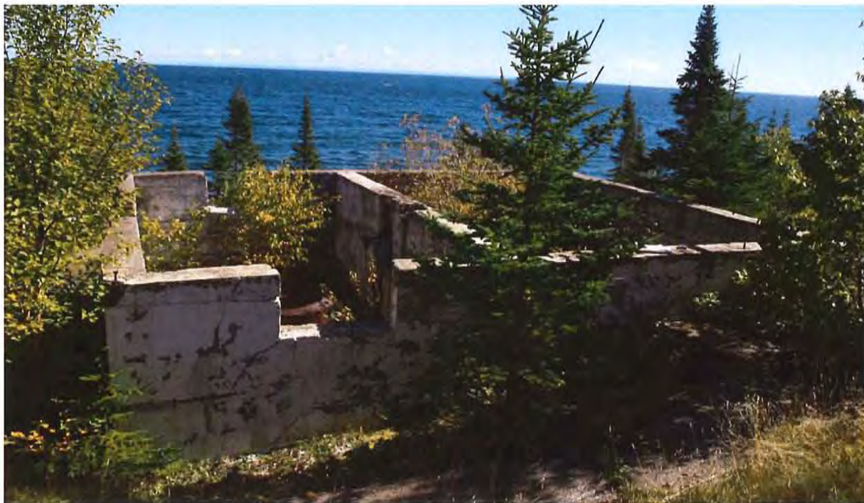
Abandoned concrete foundations.
