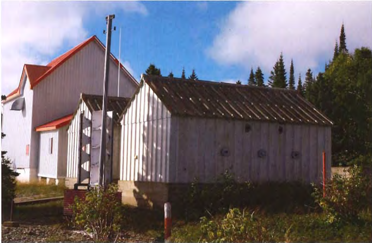
Two small storage buildings. Generally good condition.
