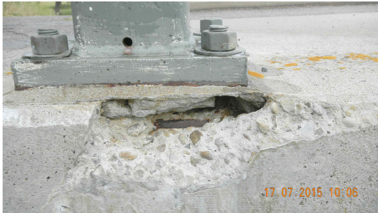
BASE PLATE REPAIR - DETAIL 3 (TYPICAL 4 LOCATIONS POST P6, P11, P16 & P20) Scale NTS
