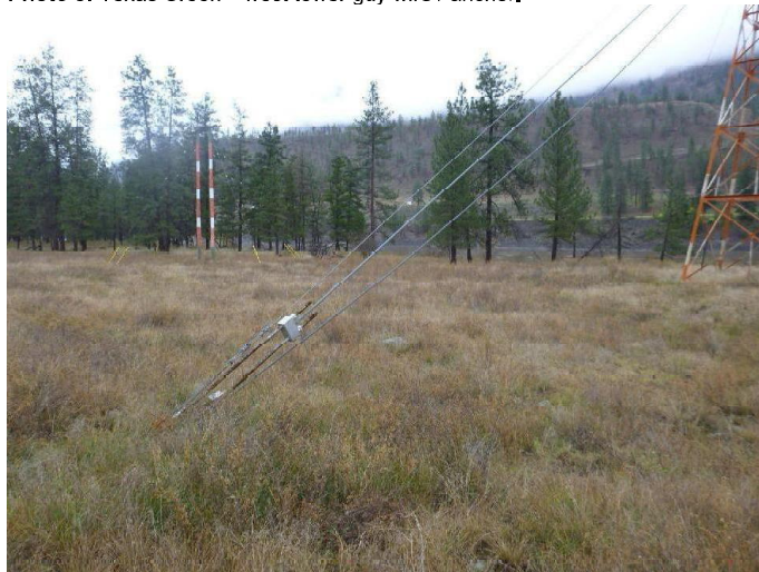
Photo 8: Texas Creek — west tower guy wire / anchor.
