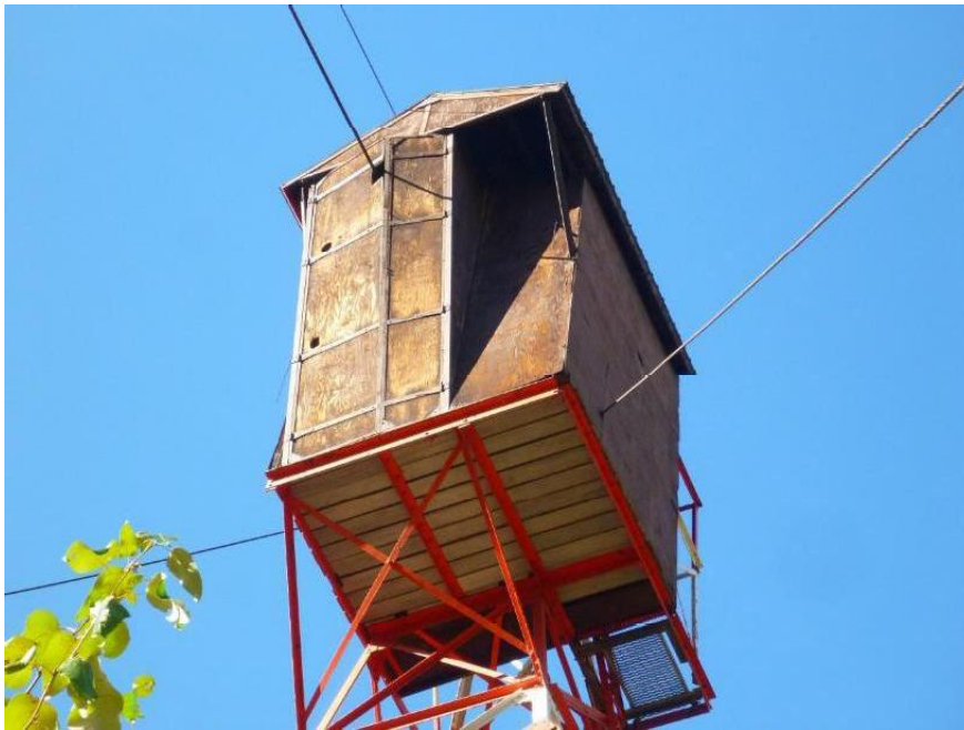
Photo 2: Birchbank Tower – west side – illustrating holes in the wood created by nesting birds.
