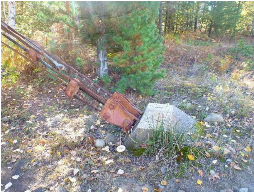
Photo 4: Anchor – west tower.
