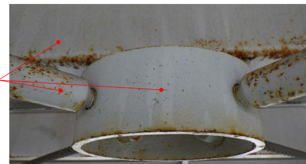
5 STEEL BRACING A300 TYPICAL EXTG CONDITION OF STEEL RINGS, ROD AND SUPPORTS
