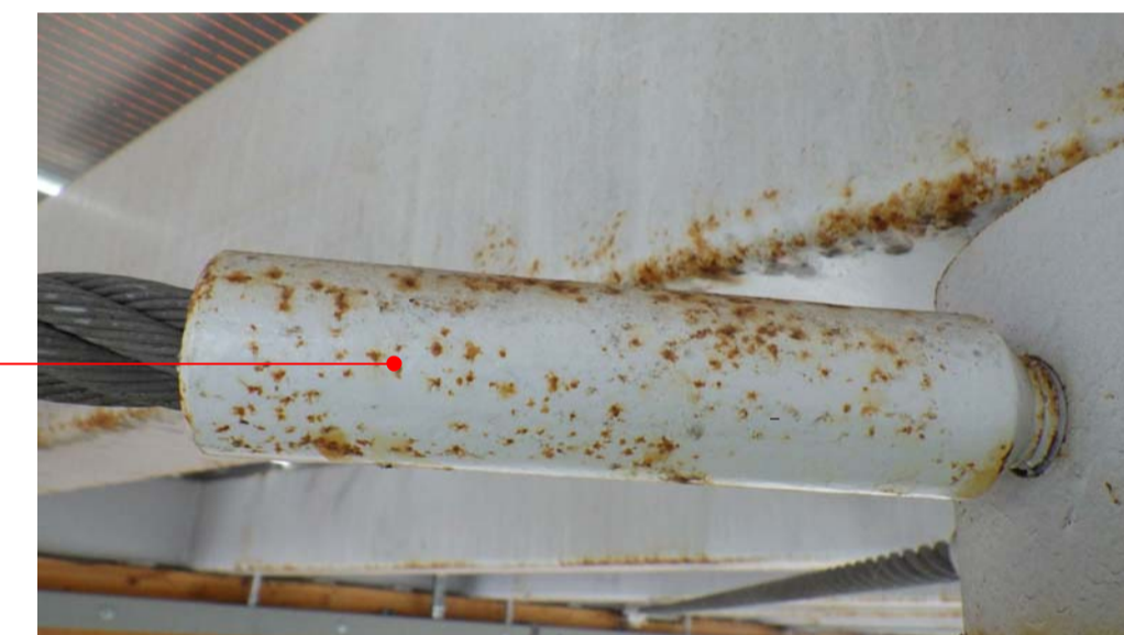
5 STEEL BRACING A300 TYPICAL EXTG CONDITION OF STEEL RINGS, ROD AND SUPPORTS
