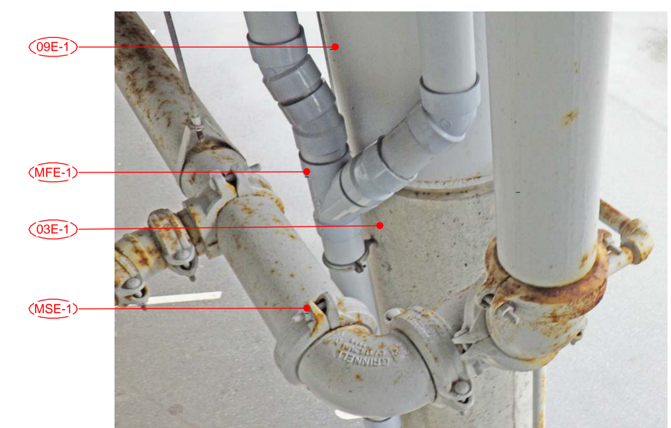
7 SIATIA SPRINKLER & RAINWATER LEADER A304 TYPICAL EXTG CONDITION OF FIRE PROTECTION PIPING
