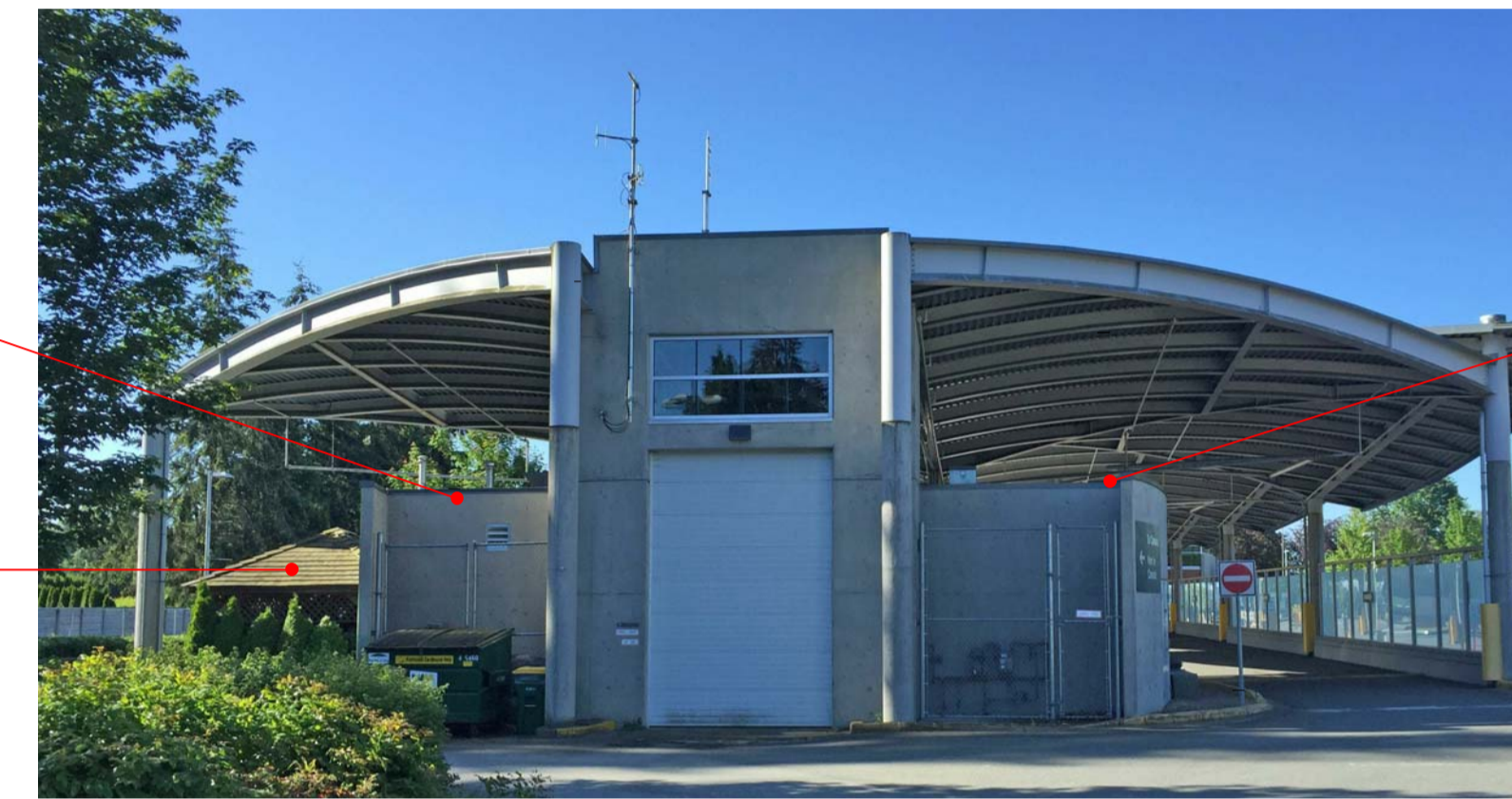
5 TIA - NORTH ELEVATION A306 TYPICAL EXTG CONDITION OF TIA CANOPY
