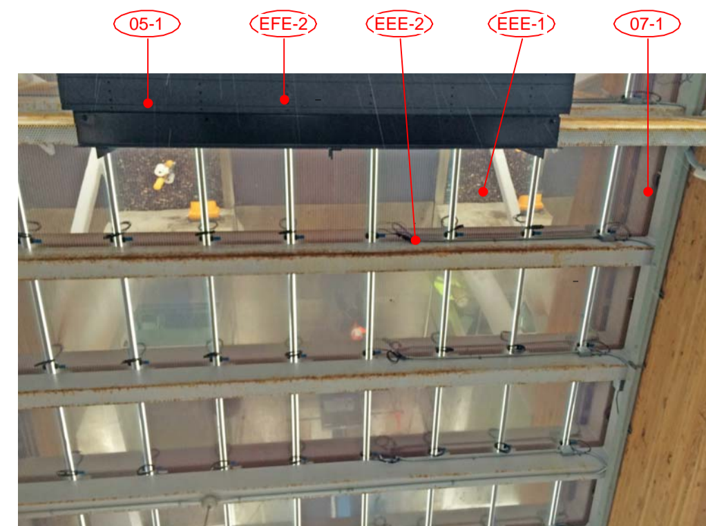
3 PHOTOVOLTAIC PANELS A300 TYPICAL EXTG CONDITION OF PV PANEL UNDERSIDE
