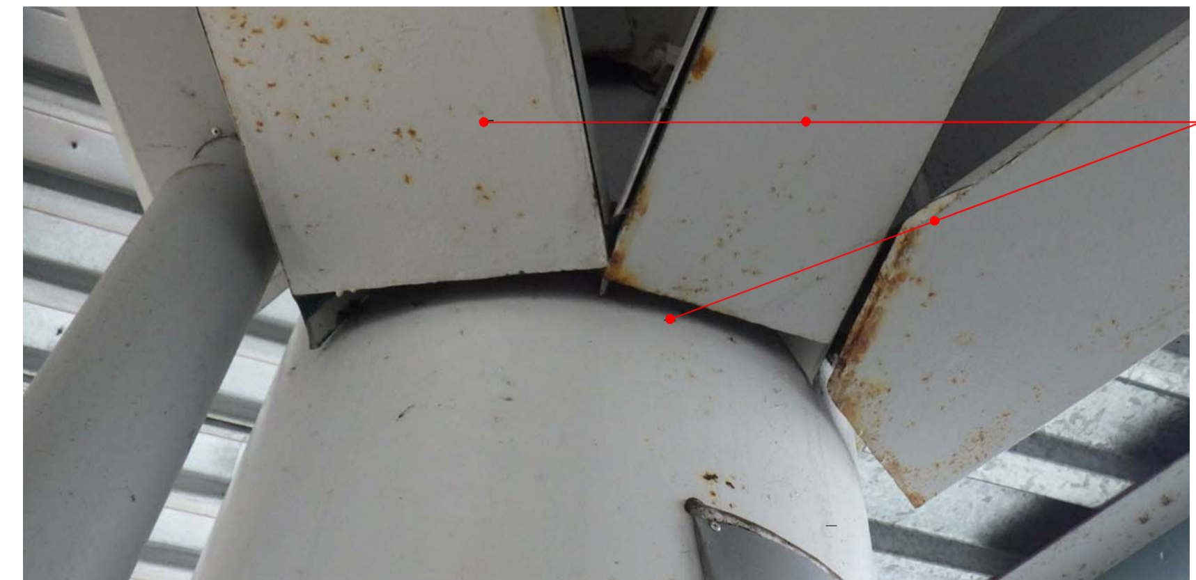
3 SIA CANOPY - TOP OF COLUMN A304 TYPICAL EXTG CONDITION OF STEEL COLUMN AND MEMBER INTERFACE
