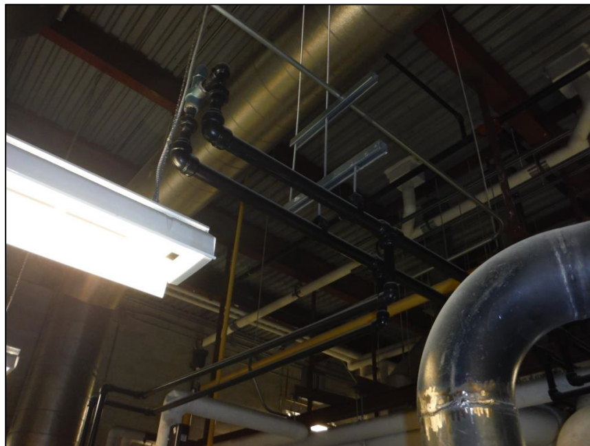
Photo 12 – Existing diesel supply and return piping to boilers to be removed.
