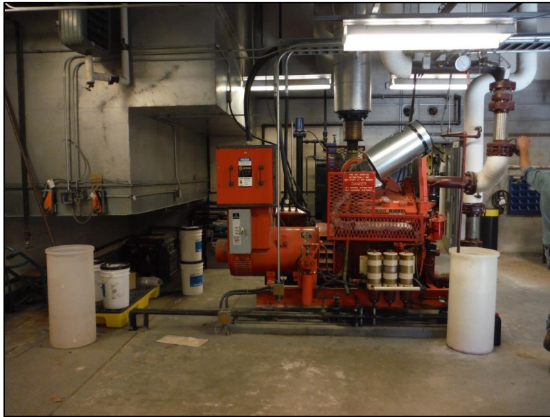
Photo 9 - Existing diesel generator. Existing fuel supply and return piping to be removed and replaced.
