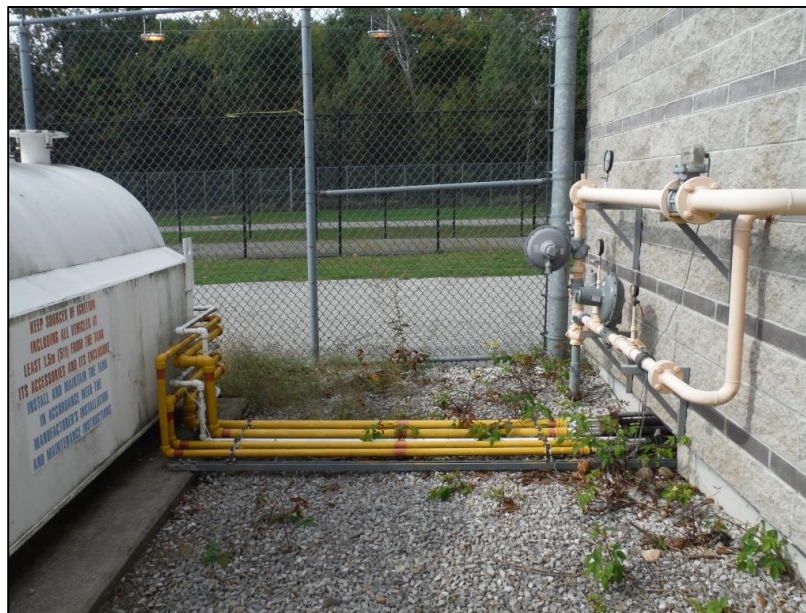
Photo 6 - Fuel piping and electrical conduit to be removed. Natural gas equipment must be protected against damage by Contractor at all times.
