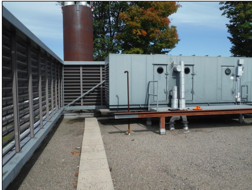
Photo 7 - Existing day tank vent (centre of photo) to be removed, and roof deck penetration to be sealed.
