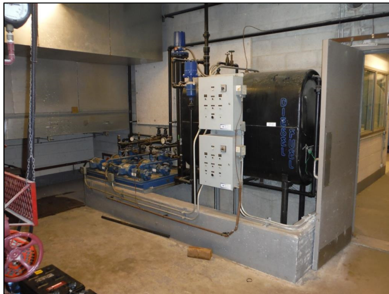
Photo 10 - Existing day tank, fuel pump sets, pump controls and level switches to be removed (generator controls to remain). New tanks to be installed in existing dike.
