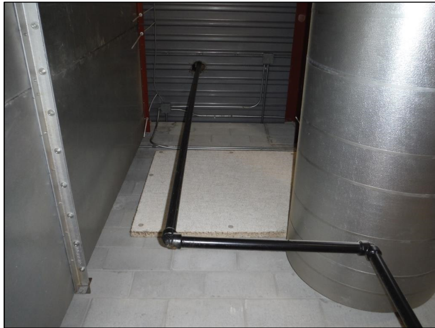
Photo 11 – Existing day tank vent to be removed, and roof deck penetration to be sealed.
