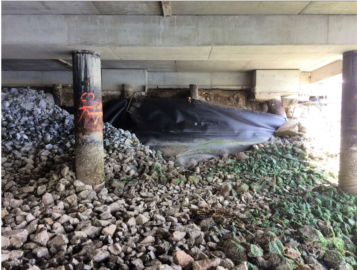
Fig. 4: View of under deck, showing exposed geofabric
