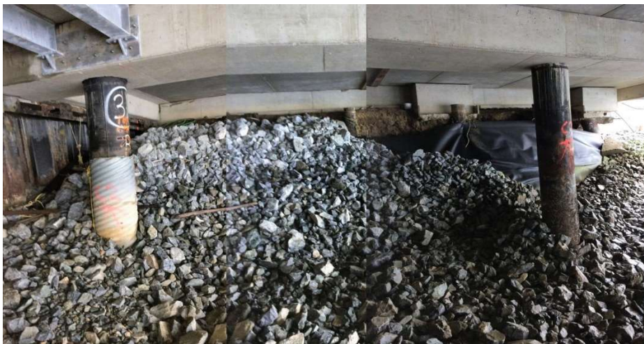
Fig. 3: View of under deck, showing exposed geofabric
