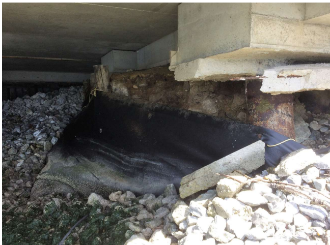
Fig.5: Exposed geofabric
