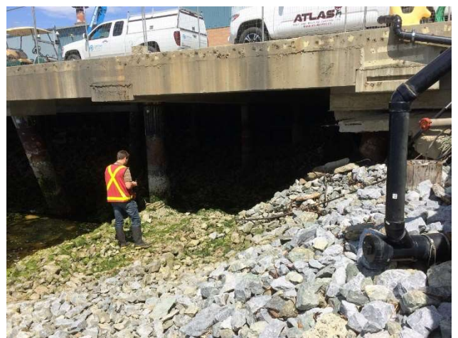
Fig. 6: Opening height = 2.8m, width from pile to slope = 2.4m
