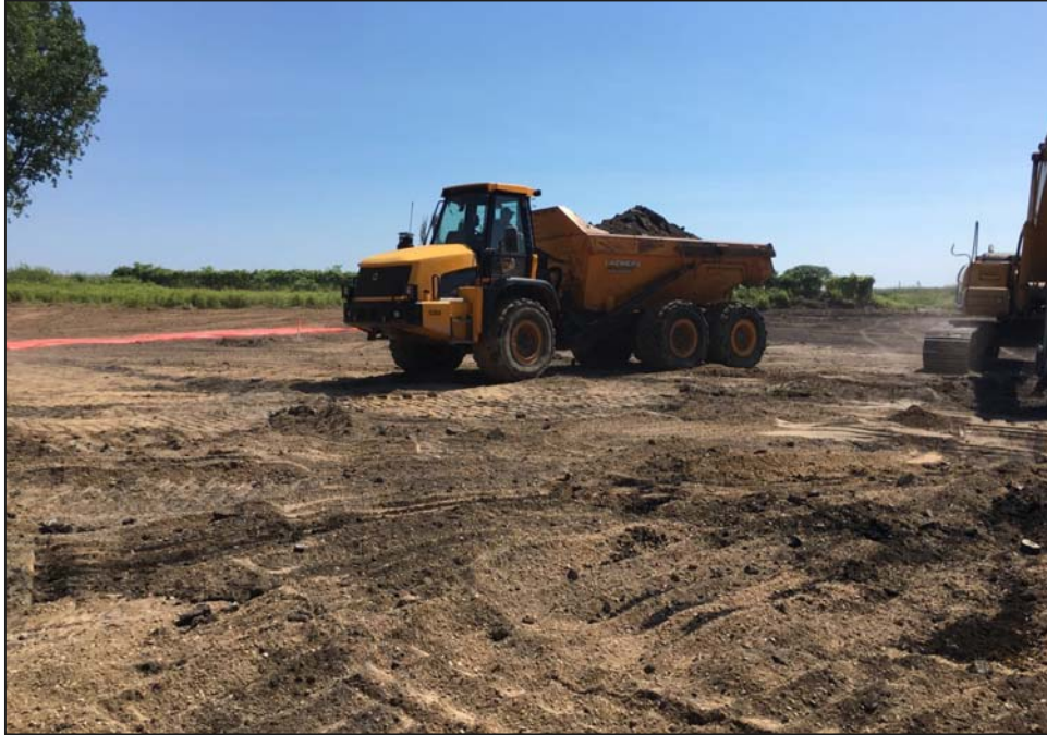
Trucks carry excavated soil to staging area
