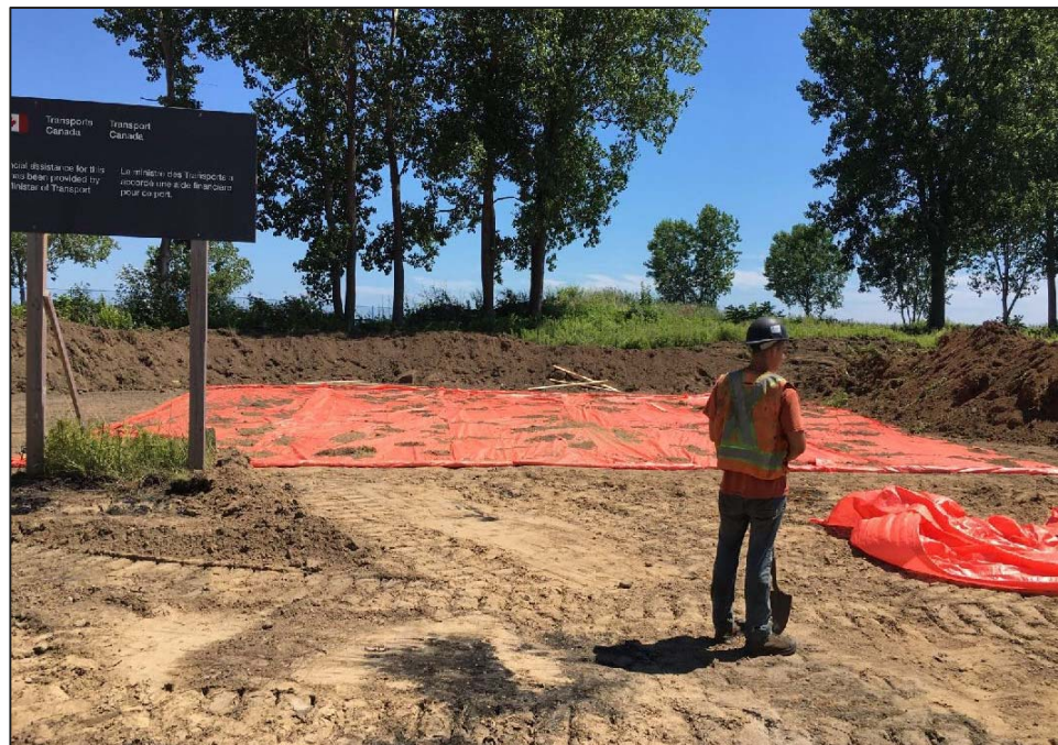
Workers laying staging area for excavated soil
