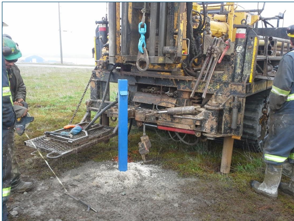
Photo 18: Monitor well MW16-2 complete with stick-up, June 16, 2016
