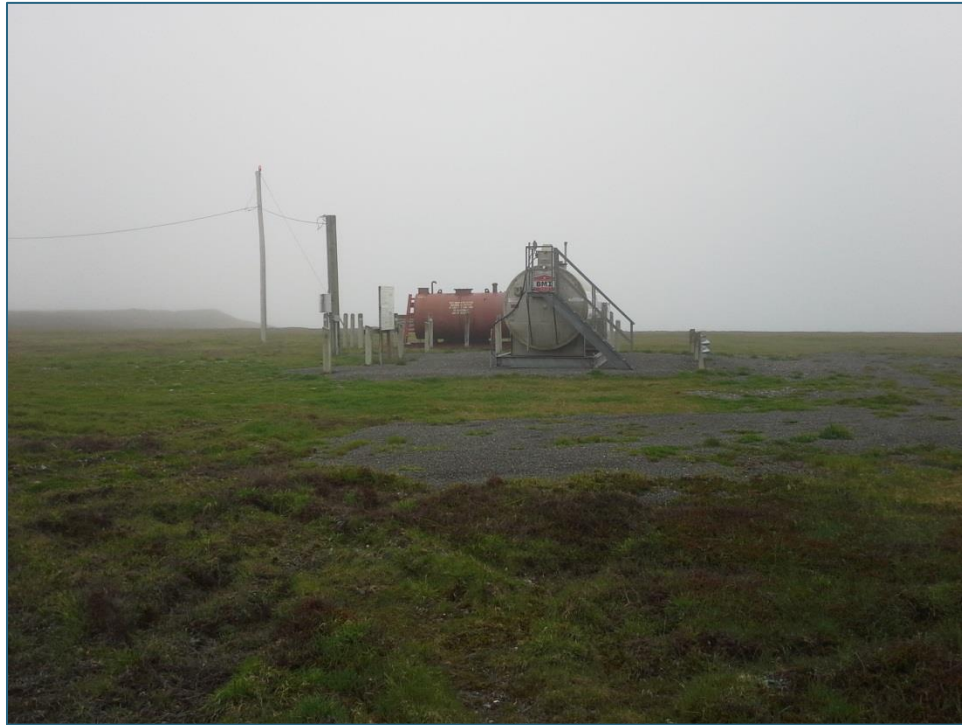
Photo 13: Two 9,090 L above ground storage tanks containing jet fuel located at the CCG helipad behind the MCTC building
