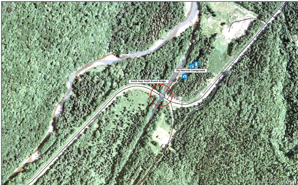
Figure 1. Showing the location of the North Aspy South River Bridge and Big Intervale Campground in Cape Breton Highlands National Park.
