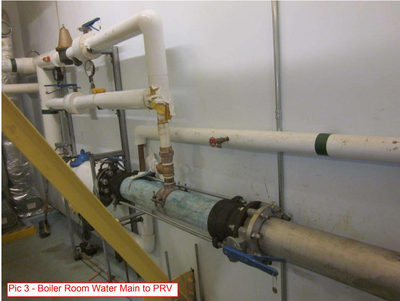
Pic 3 - Boiler Room Water Main to PRV
