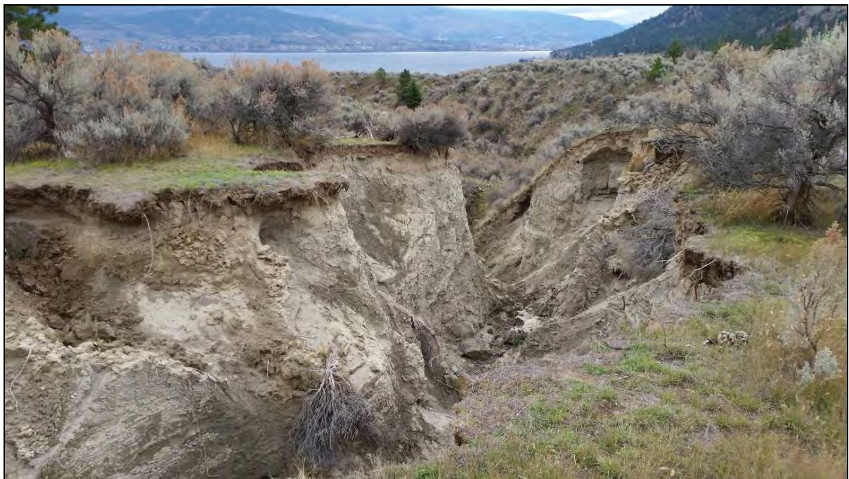
Photograph 2: South south-east view of the failure taken from the plateau
