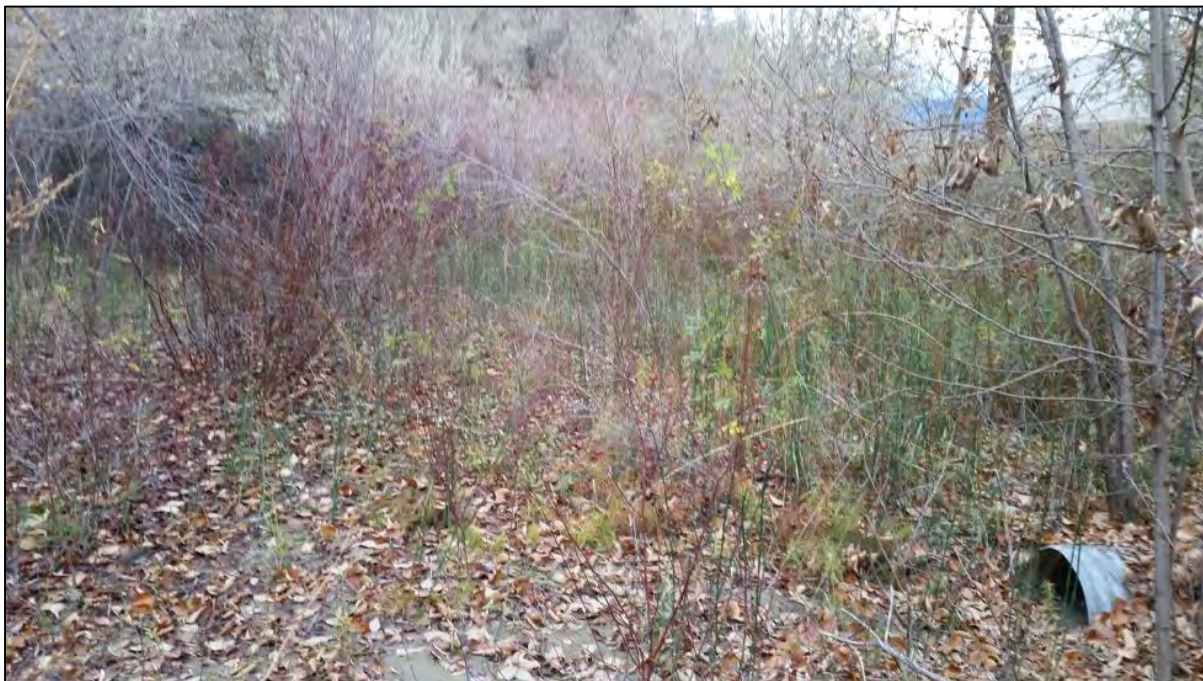
Photograph 14: North facing view toward culvert which runs toward Okanagan Lake beneath Highway 97.
