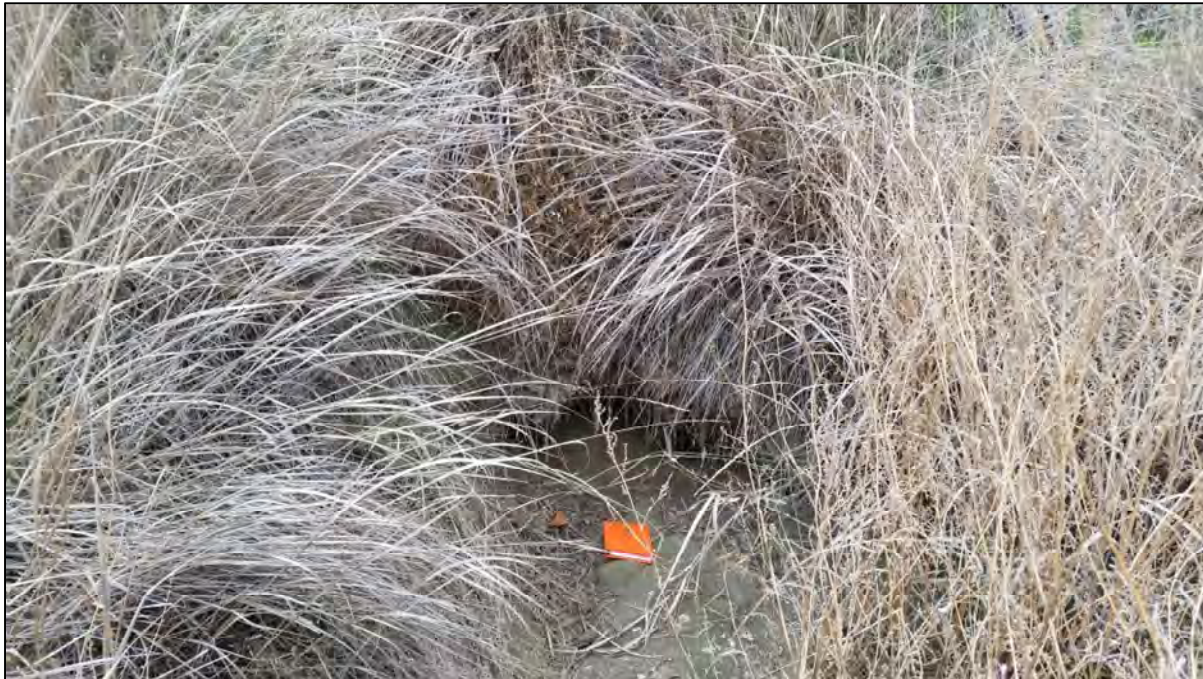
Photograph 13: Cavity at base of steep slope from which water has emerged.
