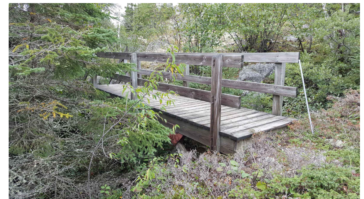
VIEW OF STRUCTURE - FACING SOUTHWEST
