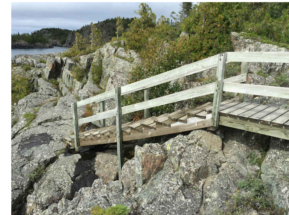
VIEW OF STRUCTURE FACING NORTHEAST
