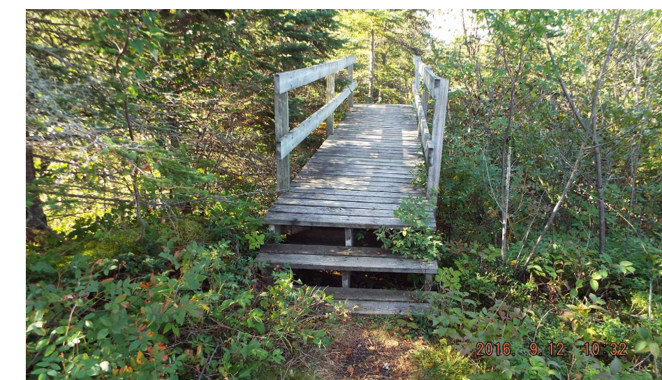
VIEW OF STRUCTURE FACING SOUTH
