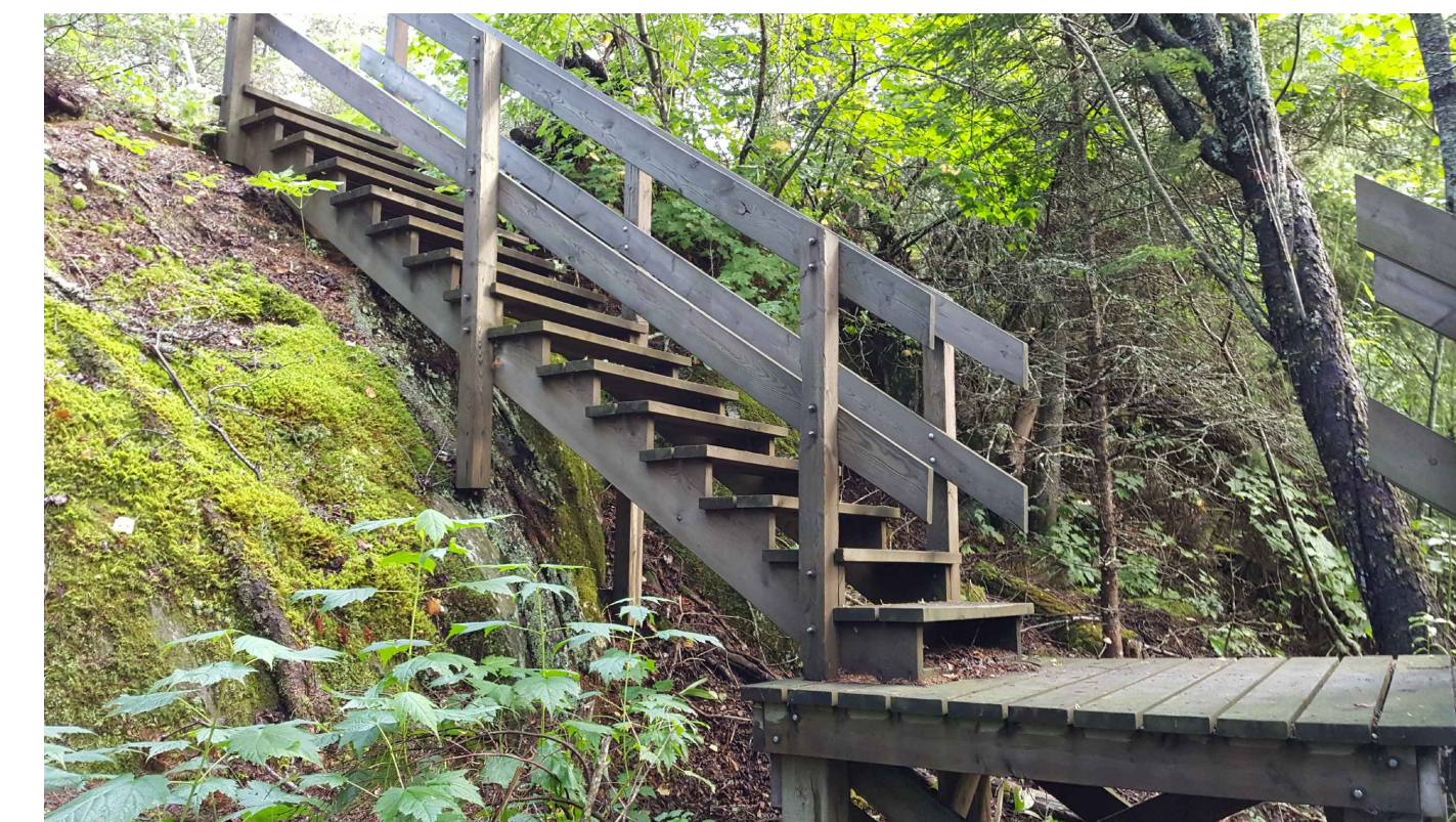
VIEW OF STRUCTURE FACING NORTHEAST
