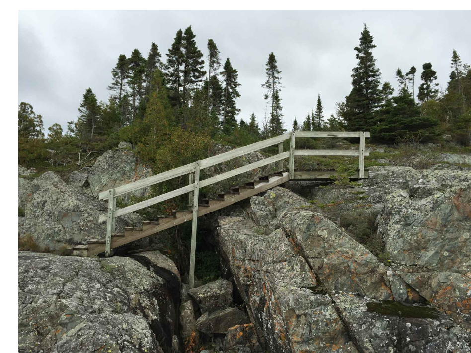
VIEW OF STRUCTURE FACING EAST
