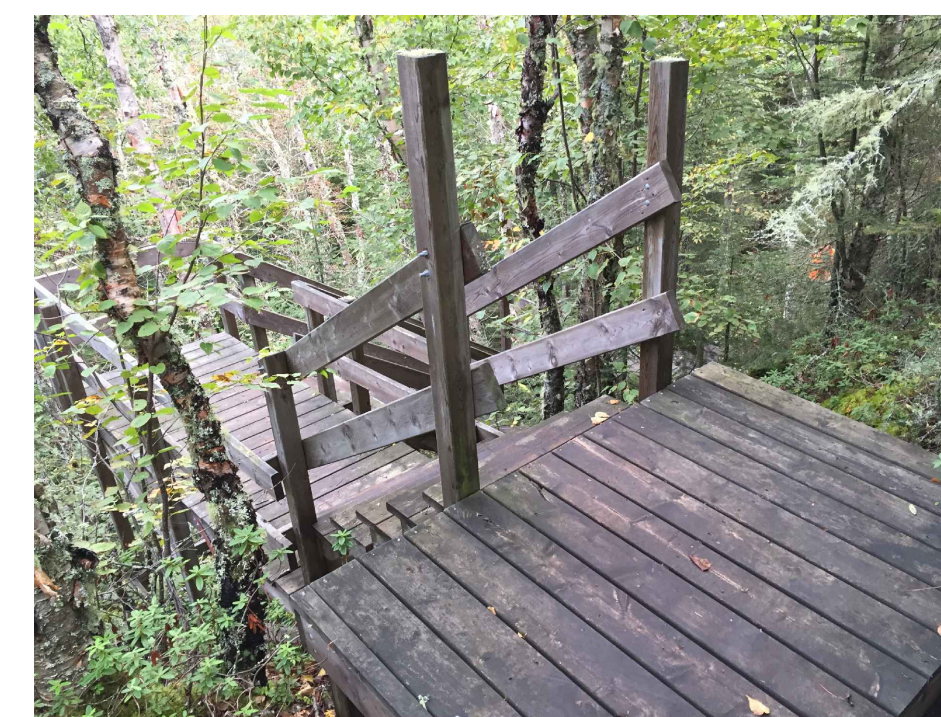
VIEW OF STAIRS #4 FACING SOUTHEAST
