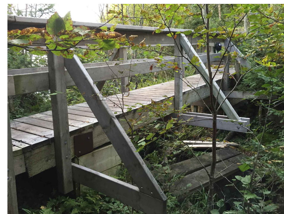
VIEW OF RAVINE CROSSING FACING SOUTHWEST
