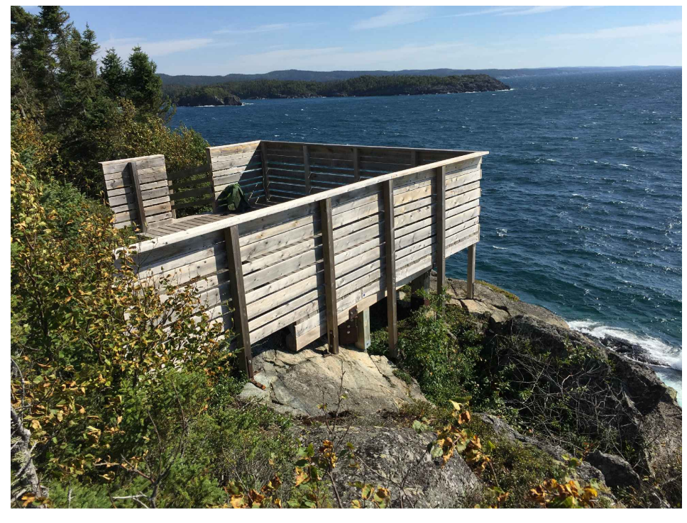
VIEW OF STRUCTURE FACING SOUTHWEST
