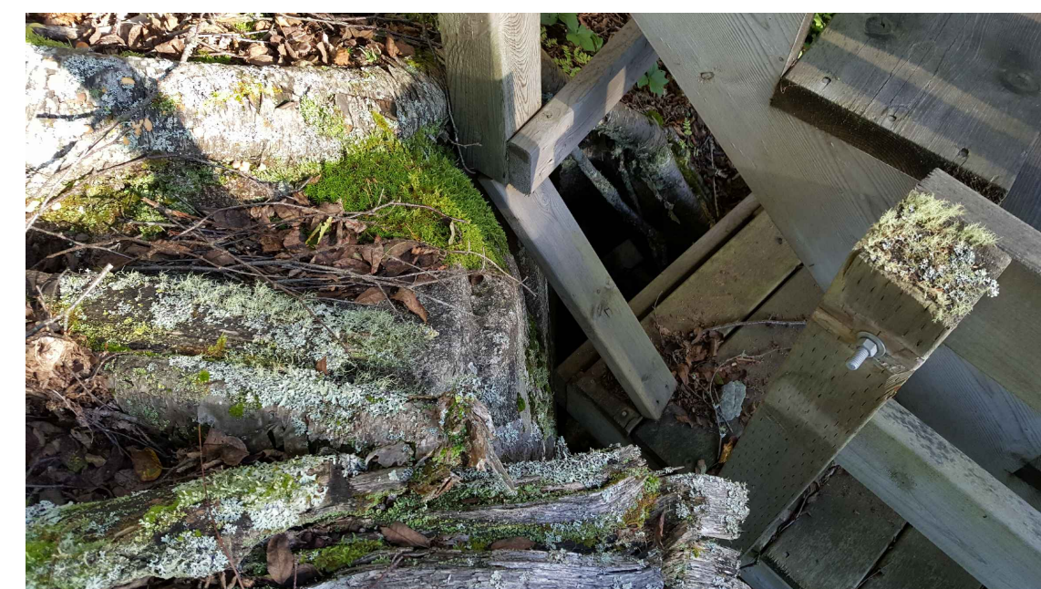
VIEW OF SUPPORT POST TO BE ANCHORED TO BEDROCK
