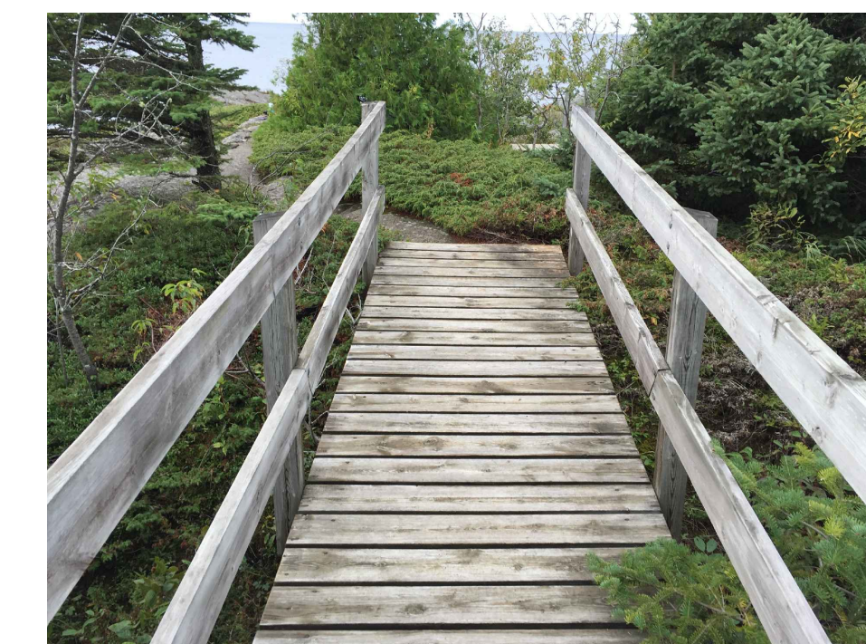
VIEW OF STRUCTURE FACING SOUTH
