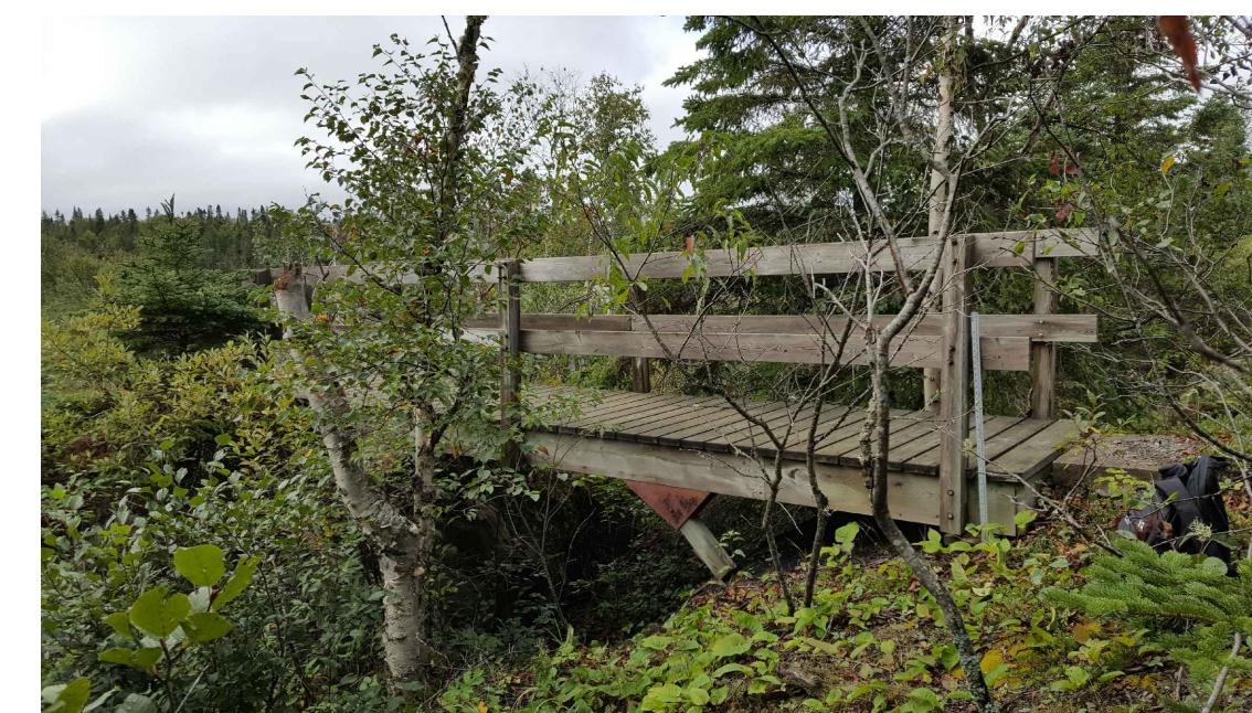
VIEW OF STRUCTURE FACING NORTHEAST
