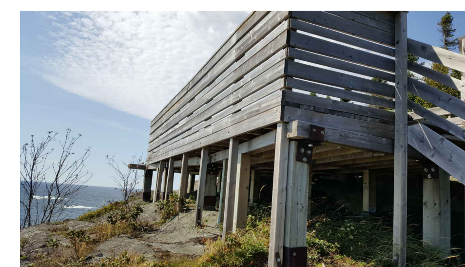
VIEW OF STRUCTURE FACING NORTHEAST
