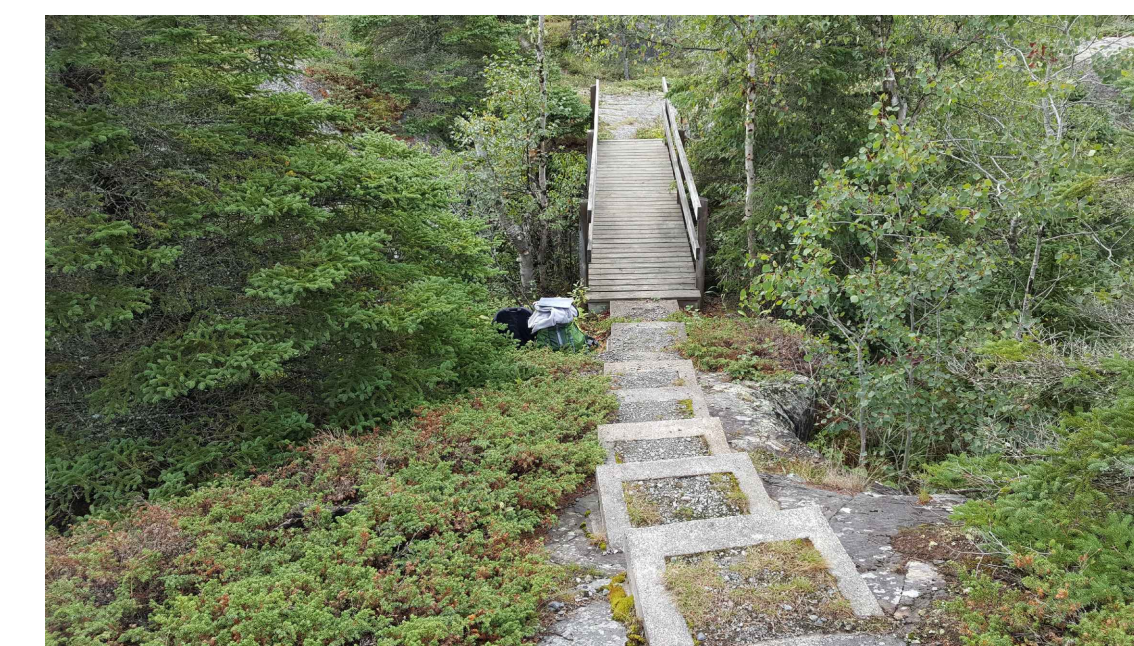
VIEW OF STRUCTURE FACING SOUTH
