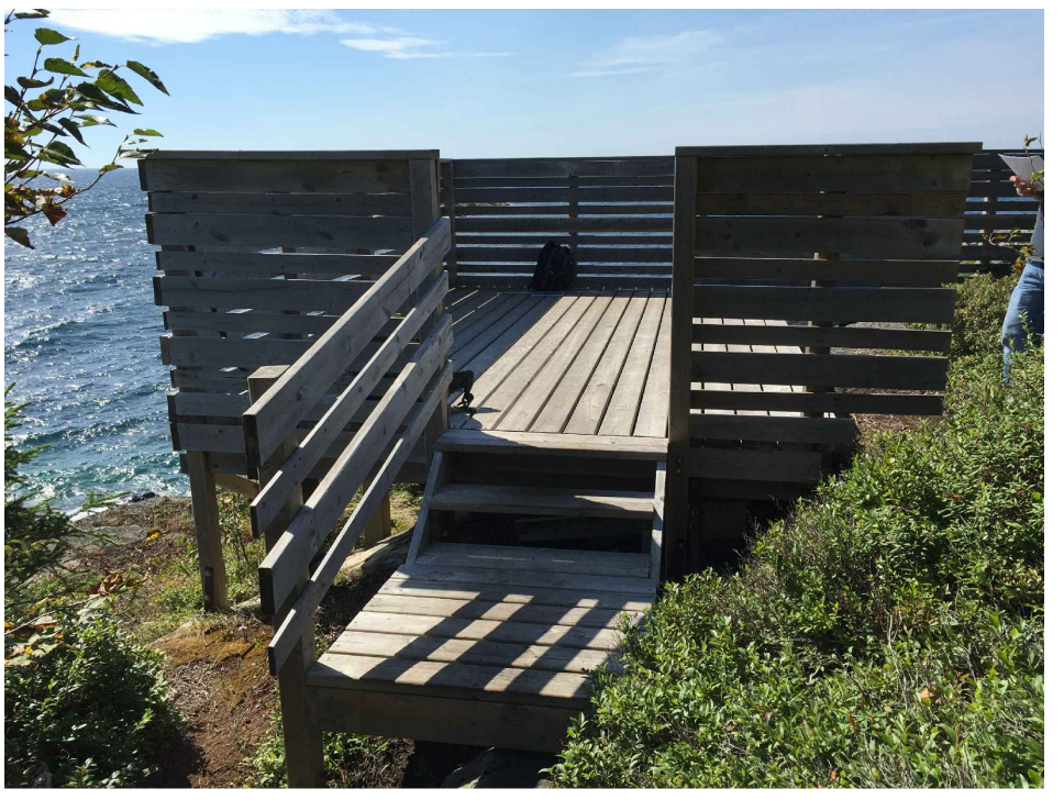
VIEW OF STRUCTURE FACING NORTH
