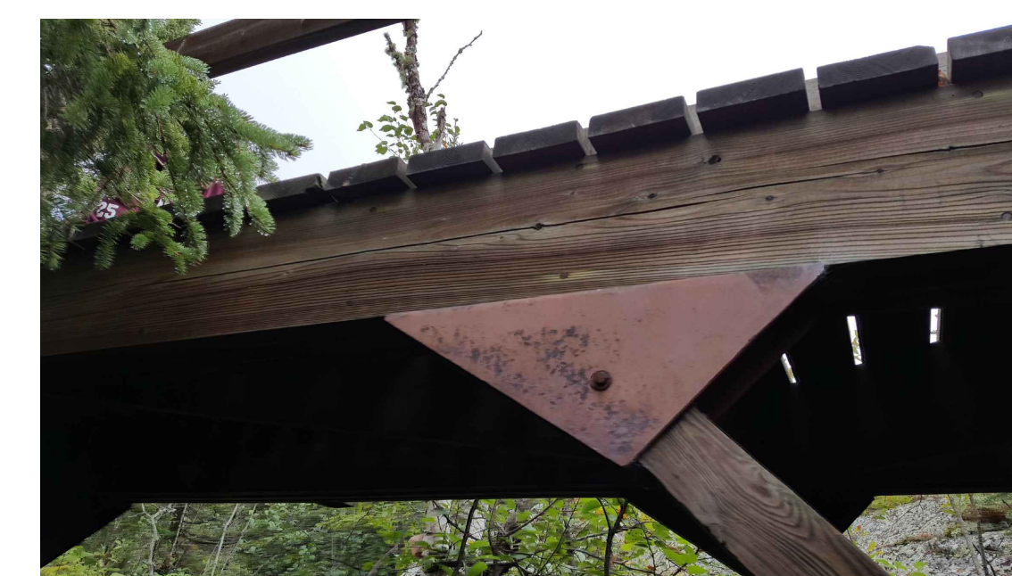
VIEW OF STRUCTURAL KNEE BRACING
