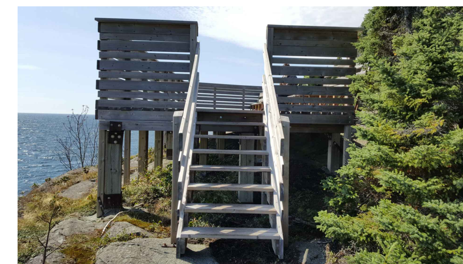
VIEW OF STRUCTURE FACING NORTH
