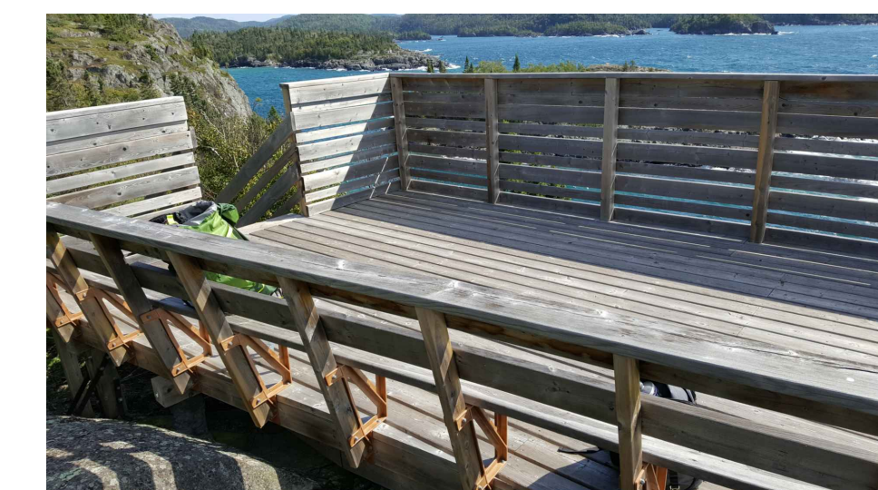
VIEW OF STRUCTURE FACING SOUTHWEST
