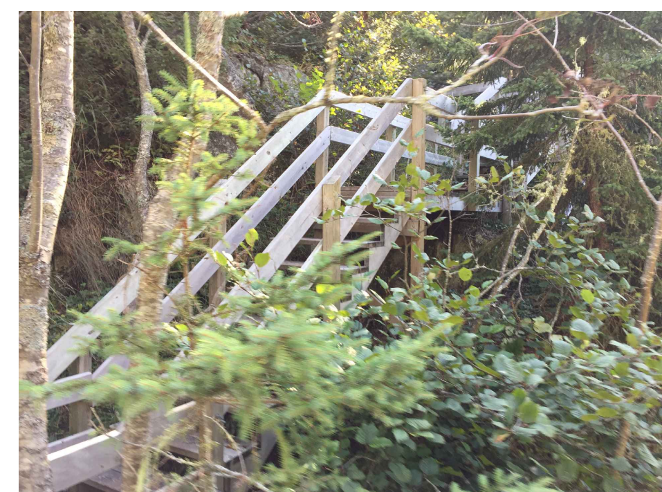
VIEW OF WEST STAIRS FACING NORTHWEST
