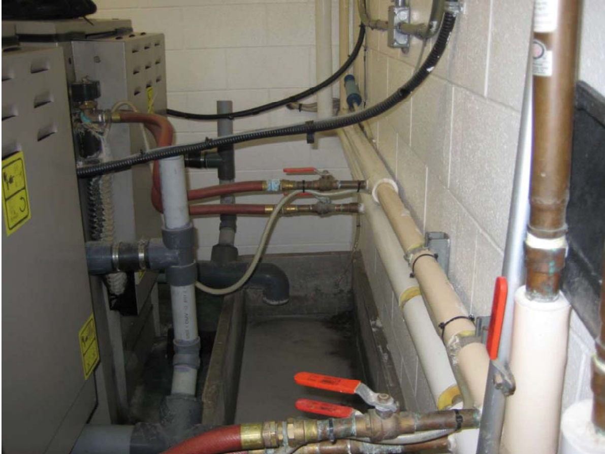
This photo presents a more in-depth look at the waterlines and the inlet connections of 1.9 cm (.75 inch). The 7.62 cm (3 inches) drain can also be seen.
