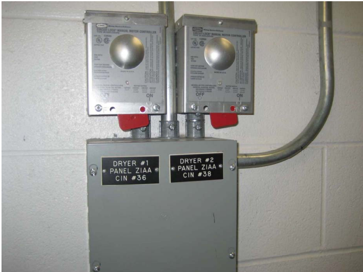
This photo shows the circuit-lock manual motor controller for the two dryers.
