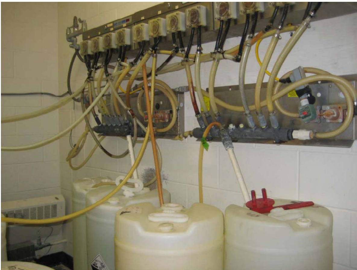
Additional photo of the wet dispensing system Knight MPL-1000, with Knight trac II- PLC controller.
