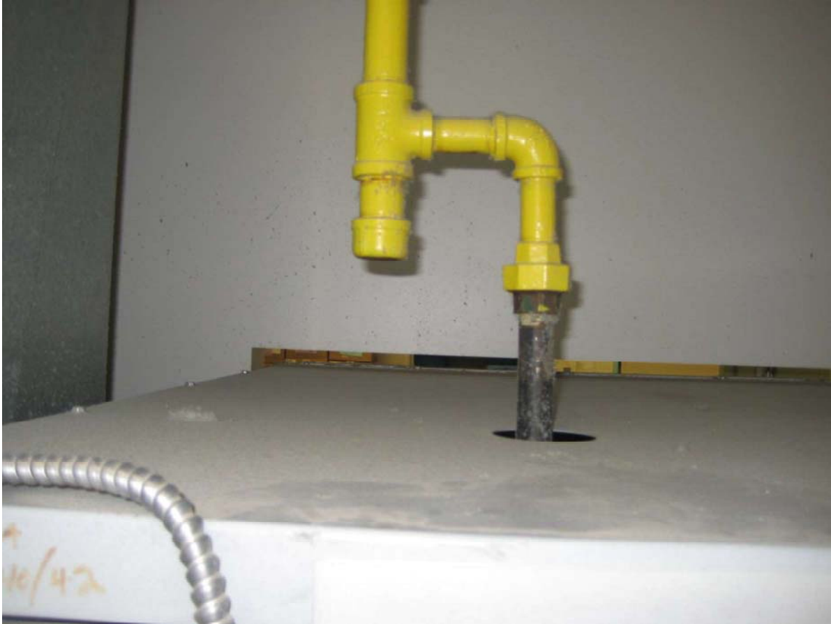
The photo shows the 1.27 cm (0.5 inch) diameter gas inlet connection. Current dryers utilize 200,000 British Thermal Units per hour
