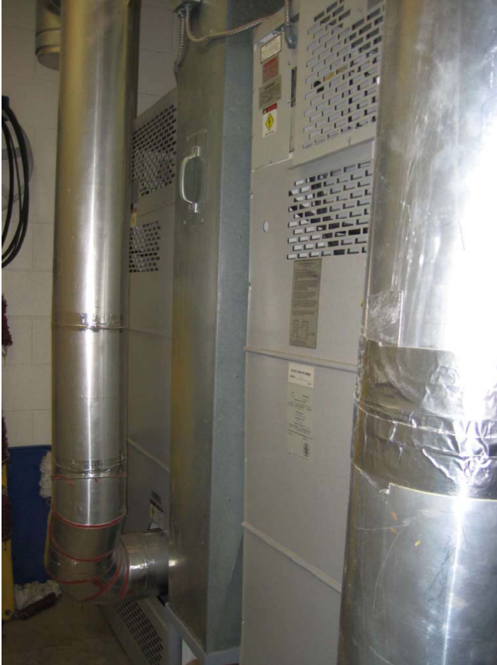
The back of the two dryers. This photo shows the 20.32 cm (8 inch) diameter venting utilized.
