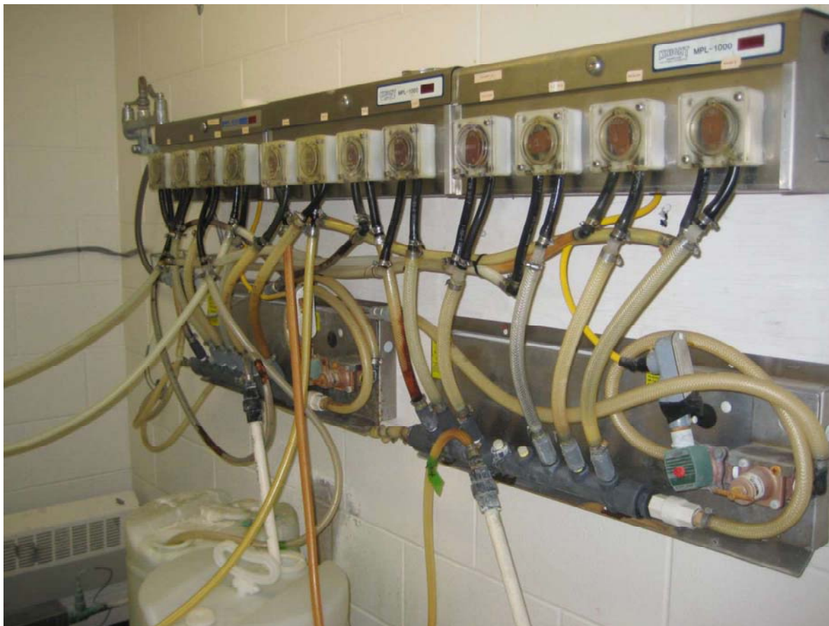
The current wet dispensing system Knight MPL-1000, with Knight trac II- PLC controller, in which installed washers must utilize.
