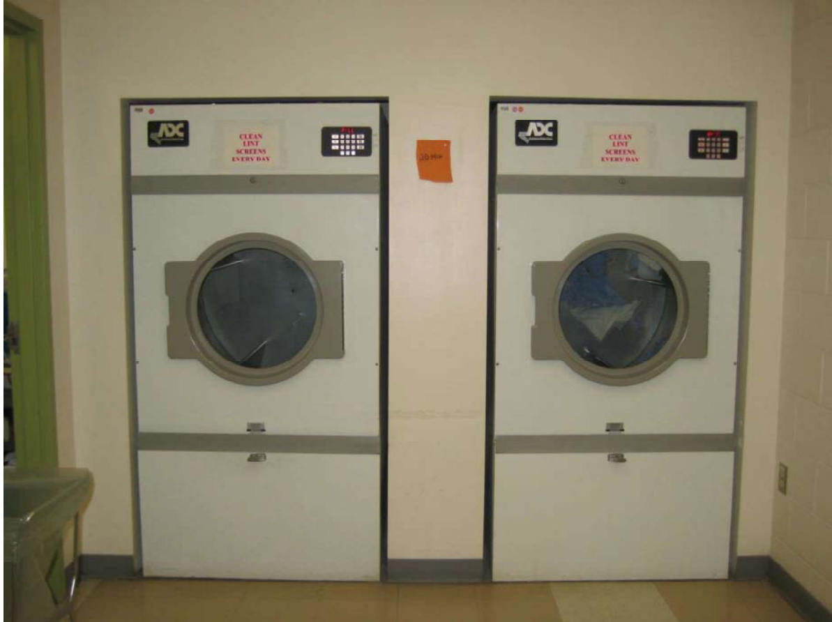
A frontal view of the two American Dryer Corp, American 75 dryers that will need to be removed and disposed of, before installing the new dryers.
