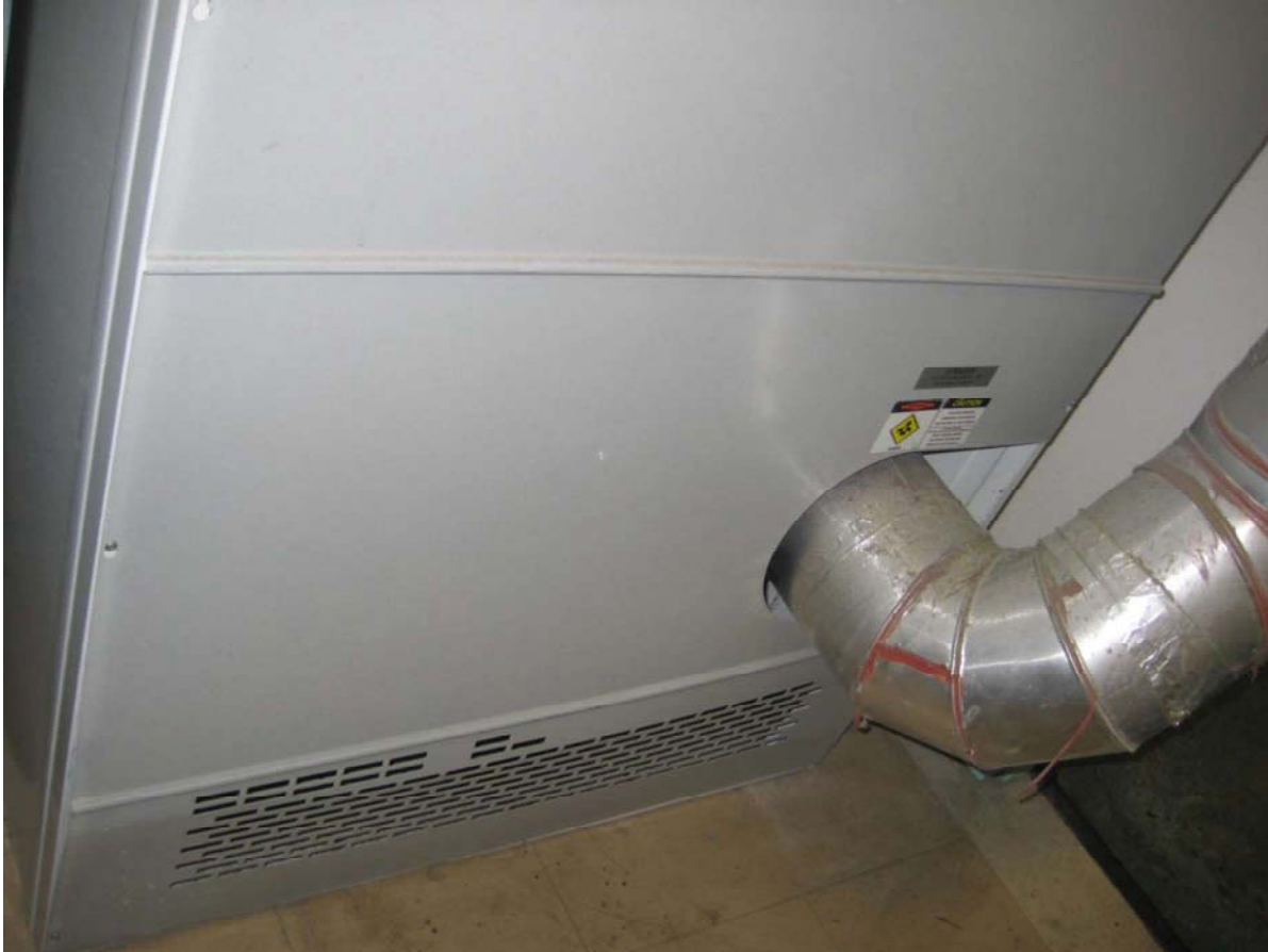
Another close up photograph of the back of the American Dryer Corp, American 75 dryer, with its 20.32 cm (8 inch) diameter vent.
