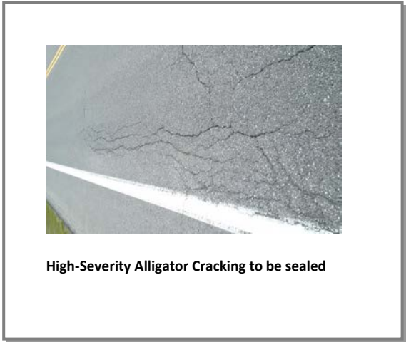
Fig. 3&4: Type of cracks observed on Aviation Parkway
