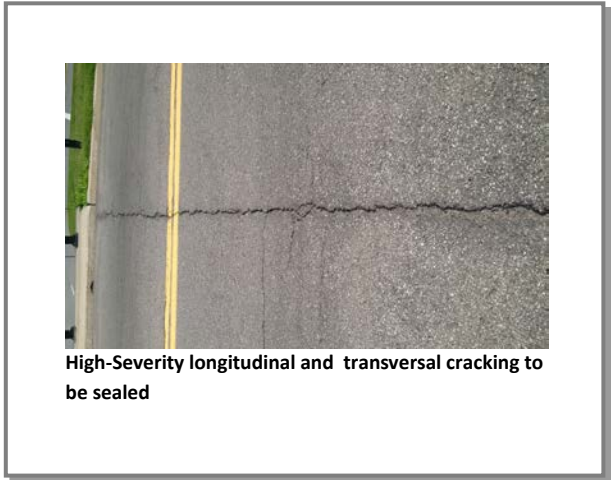
Fig. 3&4: Type of cracks observed on Aviation Parkway
