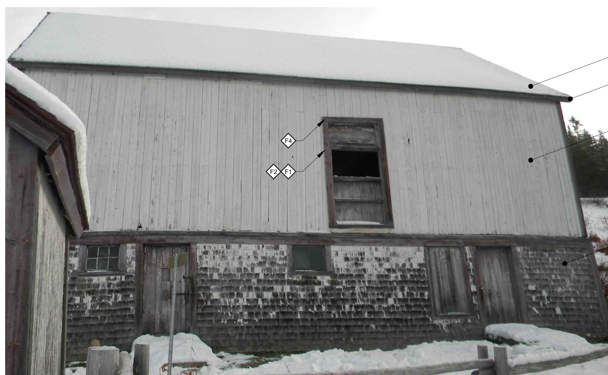
3 WEST ELEVATION (WATER SIDE) - PHOTO A21 NO SCALE
