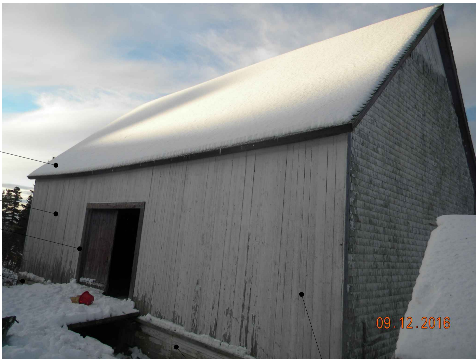
3 EAST ELEVATION (ROAD SIDE) - PHOTO A20 NO SCALE
