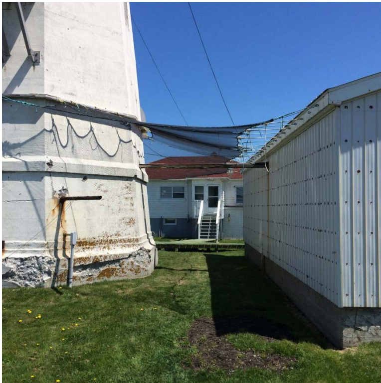
PHOTO 4: View of peeling white paint on the exterior light tower looking northeast. Note the crumbling concrete at the base of the tower.
