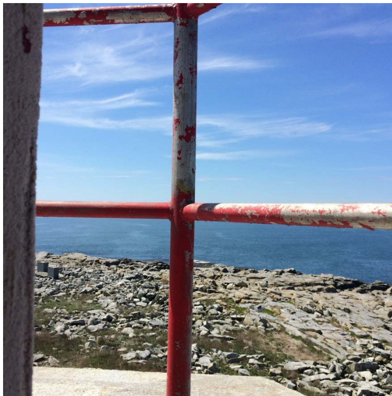
PHOTO 14: Exterior view of railing around cupola. The red paint is generally in poor condition.
