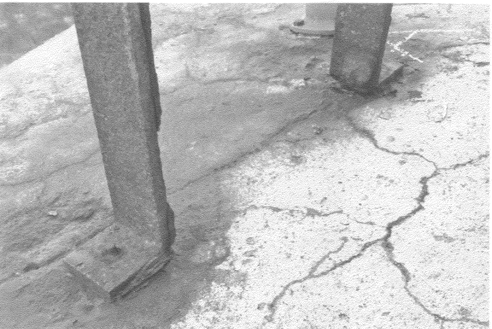
PHOTO 13 - EXTERIOR GALLERY LADDER. PROVIDE NEW METAL BOLTED CONNECTIONS. REFER TO DETAIL 2/A501.
