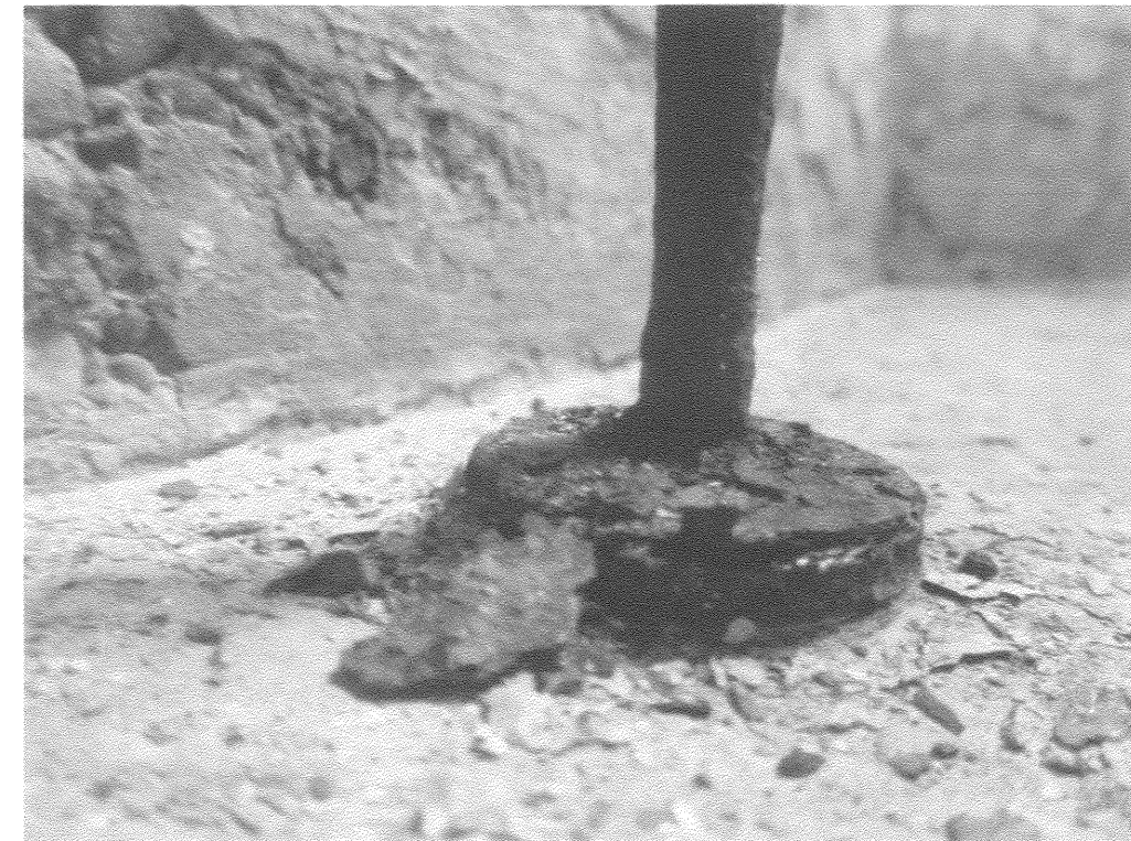
PHOTO 04 - DETAIL OF EXISTING R05 BOOT TO BE REPLACED
