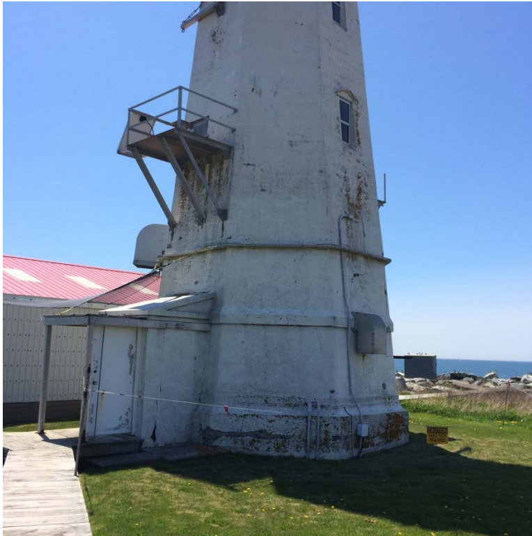
PHOTO 3: View of peeling white paint on the exterior of the light tower looking south.
