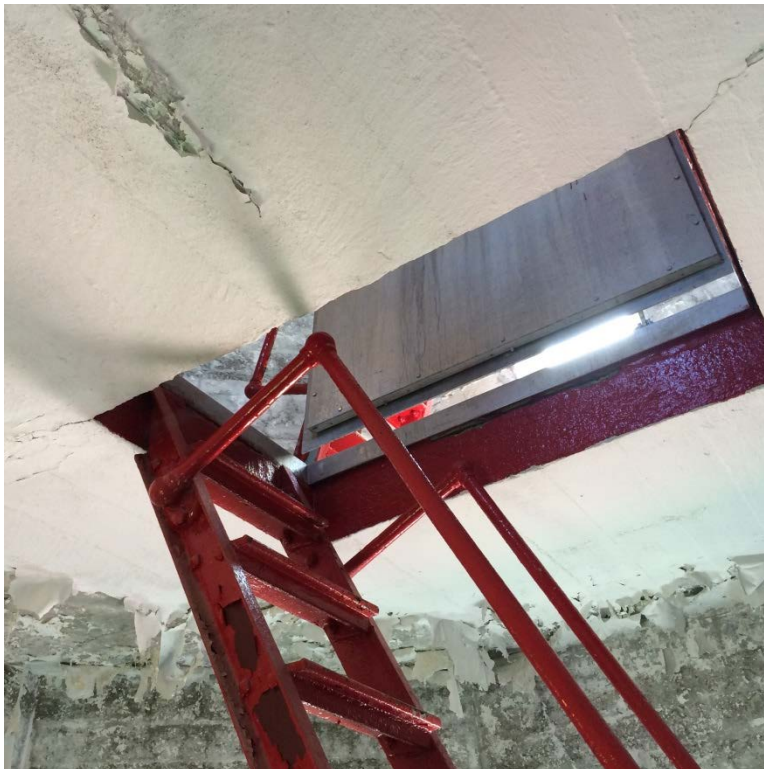
PHOTO 16: Interior view of Level 3. White ceiling paint and wall paint, both on concrete, is in poor condition.
