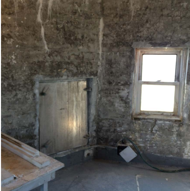
PHOTO 15: Interior view of Level 3. White paint on concrete walls is in poor condition.
