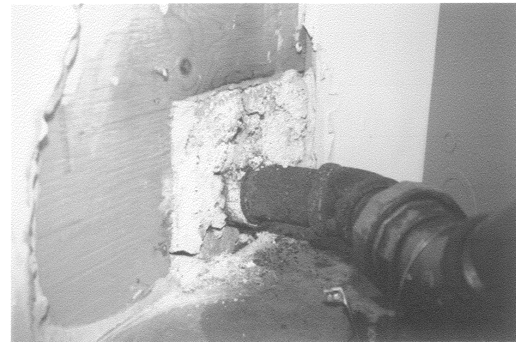
PHOTO 02 - EXTERIOR WALL PENETRATIONS AT FIRST LEVEL TO BE PROPERLY SEALED WITH FIRE PROTECTION AROUND EXHAUST. PROVIDE NEW DRYWALL FINISH, PRIME & PAINT.
