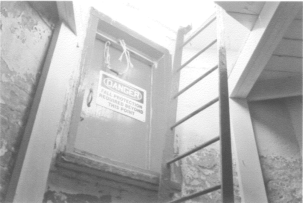
PHOTO 16 - INTERIOR OF GALLERY HATCH. SILL AND HEAD CASING ARE ORIGINAL AND ARE TO BE RETAINED. JAMBS AND DOOR TO BE REPLACED. REFER TO DETAIL 3/A500
