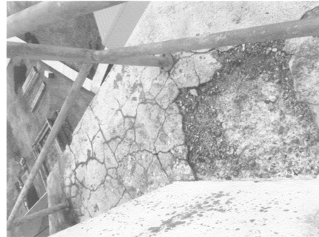
PHOTO 06 - NEW TRAFFIC COATING PROVIDED. NEW RAIL TO BE 125mm FROM GALLERY EDGE. REFER TO DETAIL 1/A500.
