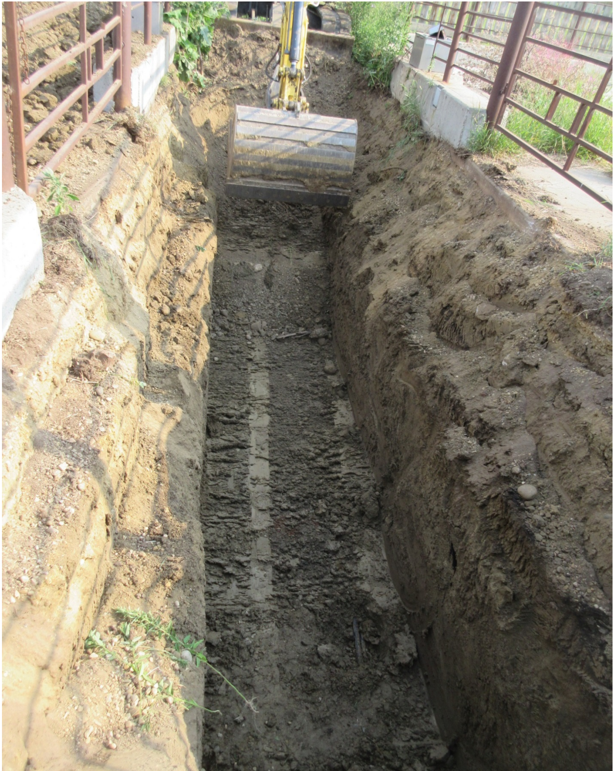
Figure 2: Trench is approximately 40' long x 3+ feet wide, with 8-foot deep sides. The ground is composed of stable clay soils. There is no slumping or water infiltration.
