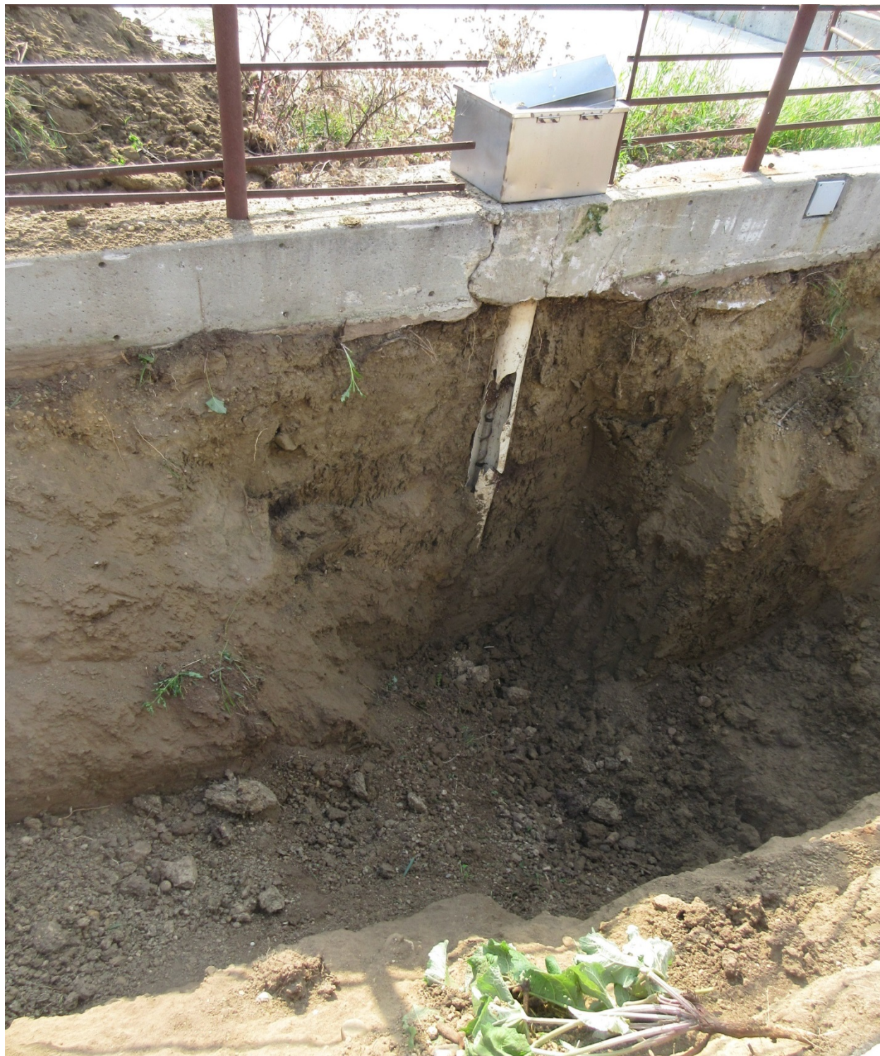
Figure 3: Vertical riser to waterer. Water line curves to upstanding. There are no joints. The riser casing was damaged by excavation work.
