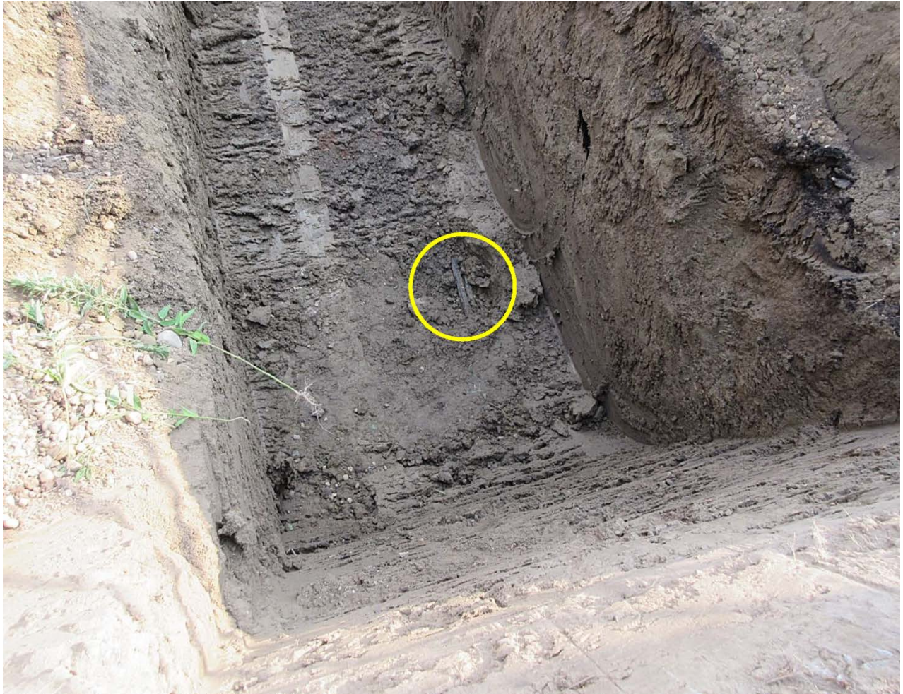
Figure 1: Exposed horizontal waterline. The water line is approximately 8 feet below grade.
