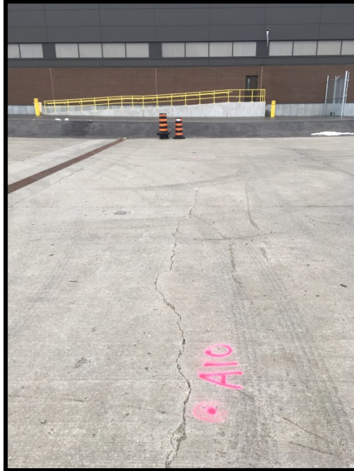
Photograph 7: View from concrete apron (north of former Hangar 6) looking east towards new Hangar 6
