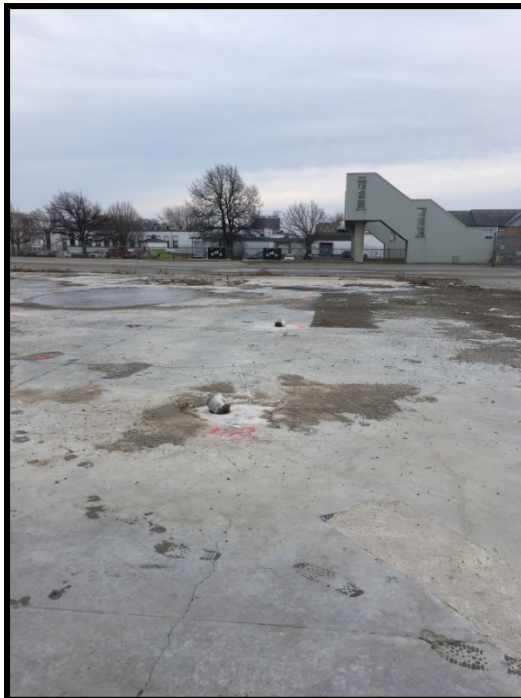
Photograph 2: View from north edge of concrete pad (to be removed) of former Hangar 6 looking south at pedestrian bridge over Highway 2
