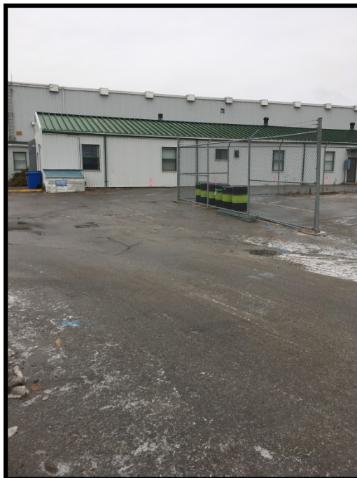
Photograph 10: View from North Star Drive: southwest end of area to be excavated looking, west towards Building 65 (part of Hangar 7)
