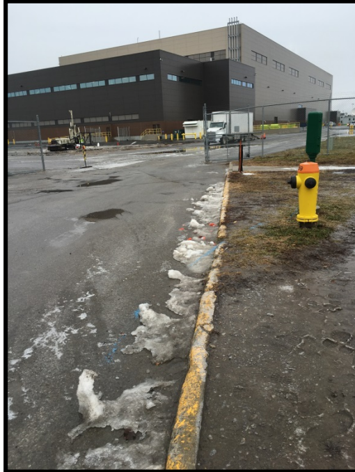
Photograph 9: View from south North Star Drive (west of pedestrian bridge), looking east at concrete pad of former Hangar 6 and new Hanger 6 beyond
