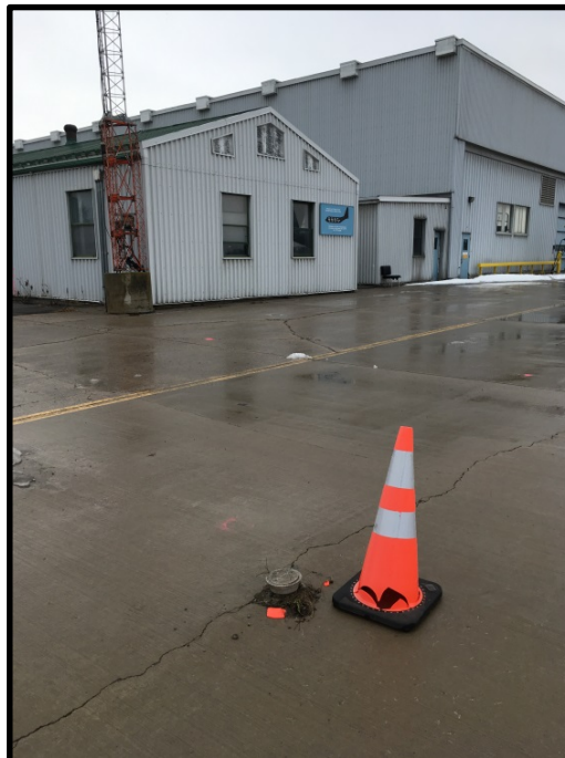
Photograph 12: View from north end of apron (by monitoring well MW14-131), looking south west, Building 65 and Hangar 7 beyond
