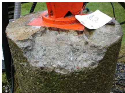
Figure 1-1 - Lightning strike on tower causing part of foundation to break apart
