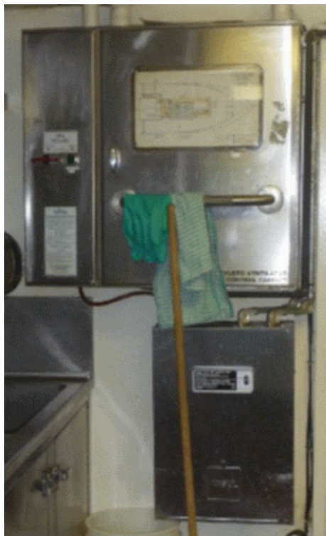
Exhaust hood control cabinet and fire suppression system
