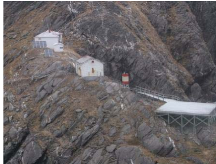
Photo 5: View of Baccalieu Island Lightstation.
