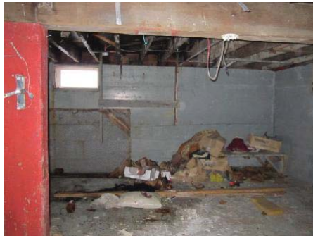
Photo 26: View of Basement 2 in double dwelling.
