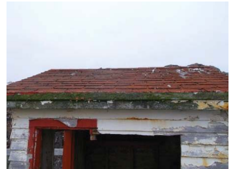
Photo 3: View of roof of upper winch house.
