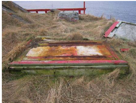
Photo 8: View of concrete foundation at location of former winch house (BLI-PS27).
