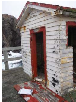
Photo 2: View of northwest side of upper winch house.
