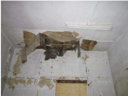
Photo 10: View of Room 2 in old equipment building. Note: fluorescent light fixture.
