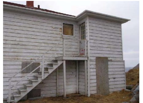
Photo 3: View of southeast side of double dwelling.
