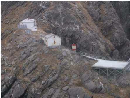
Photo 1: View of Site exterior structures at Baccalieu Island Lightstation.
