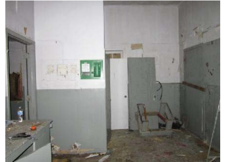
Photo 9: View of Room 2 in old equipment building.
