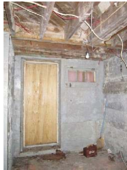
Photo 20: View of Basement 1 in double dwelling.
