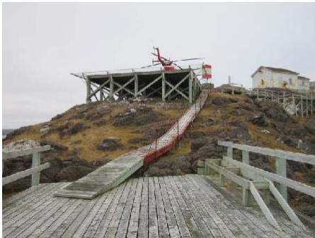
Photo 1: View of old equipment building (next to helicopter landing pad and walkway).
