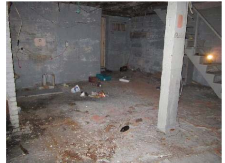
Photo 21: View of Basement 1 in double dwelling.
