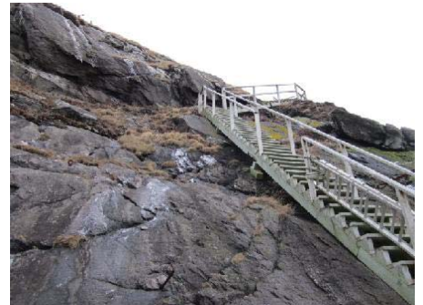
Photo 12: View of stairway to lower landing area.
