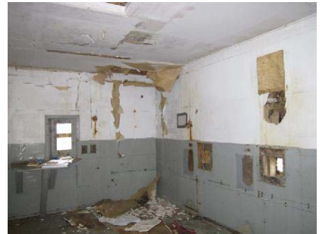
Photo 15: View of Room 3 in old equipment building.
