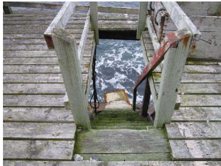
Photo 14: View of lower landing deck stairway.
