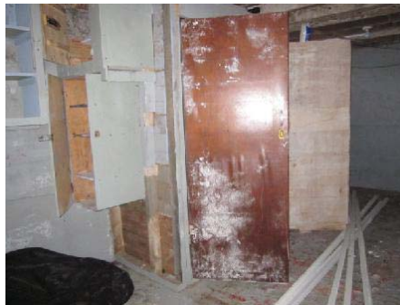
Photo 23: View of Basement 1 in double dwelling.
