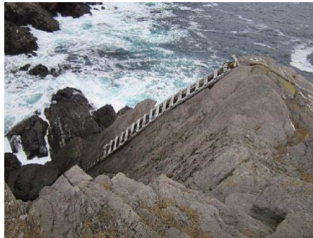
Photo 2: View of ladder to upper landing area.
