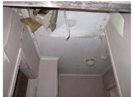
Photo 72: View of smoke detector on ceiling in Hallway 2.
