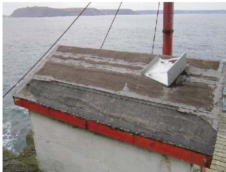
Photo 5: View of southeast side of lower winch house.
