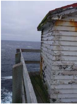
Photo 4: View of northeast side of upper winch house.
