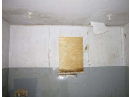
Photo 8: View of Room 1 in old equipment building.
