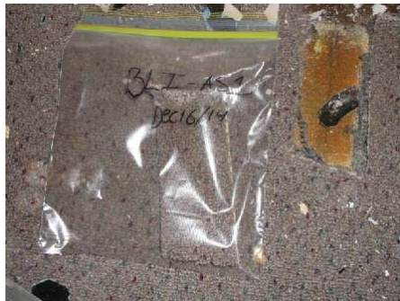
Photo 29: View of carpet and mastic sample BLI-AS1.
