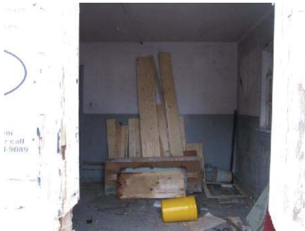
Photo 5: View of Room 1 in old equipment building.
