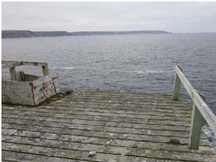
Photo 13: View of lower landing deck and railing.
