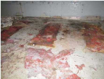
Photo 13: View of Room 3 in old equipment building.
