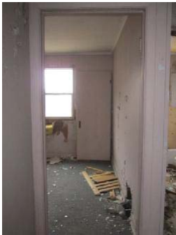
Photo 13: View of Bedroom 3-1 in double dwelling.
