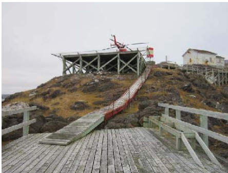
Photo 4: View of upper landing deck and stairway to helicopter landing pad.
