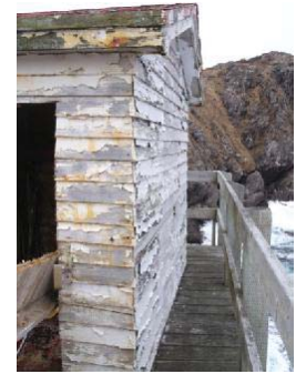
Photo 6: View of southeast side of upper winch house.
