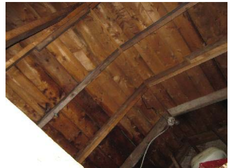
Photo 18: View of attic in old equipment building.
