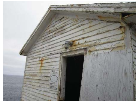
Photo 3: View of north side of old equipment building.
