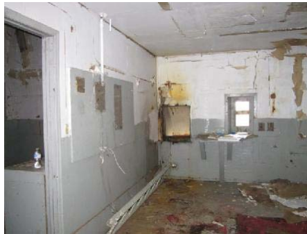
Photo 14: View of Room 3 in old equipment building.
