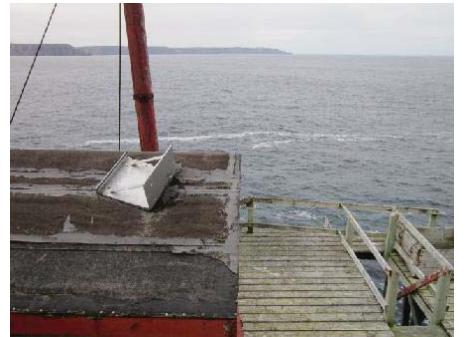
Photo 3: View of lower landing deck and winch house.
