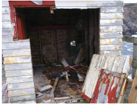
Photo 5: View of southwest side of upper winch house.
