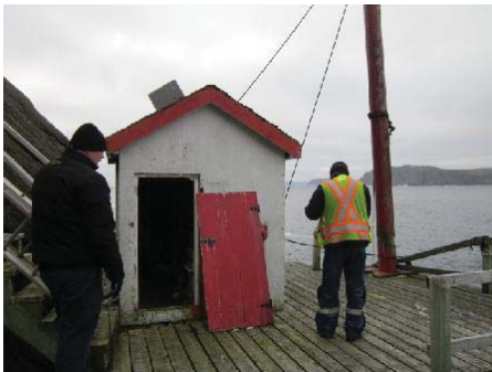
Photo 4: View of lower landing deck and winch house.
