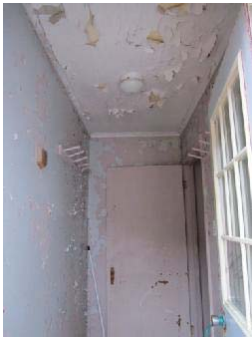
Photo 7: View of Porch 1 in double dwelling. Note: flaking paint.
