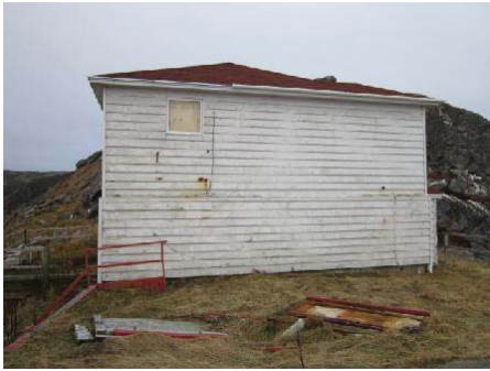
Photo 4: View of southwest side of double dwelling.
