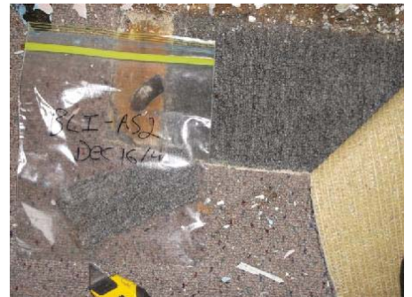
Photo 30: View of carpet and mastic sample BLI-AS2.
