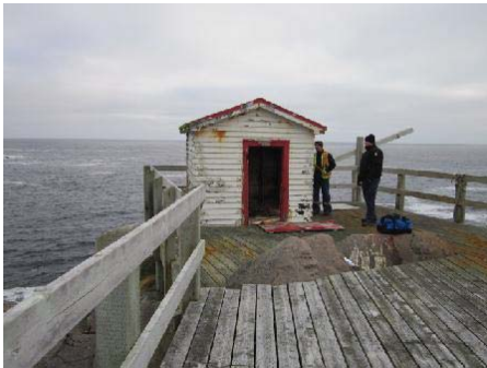
Photo 1: View of upper landing deck and winch house.
