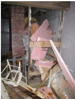
Photo 28: View of Basement 2 in double dwelling. Note: rigid foam insulation.
