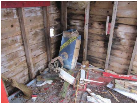
Photo 7: View of interior of upper winch house.
