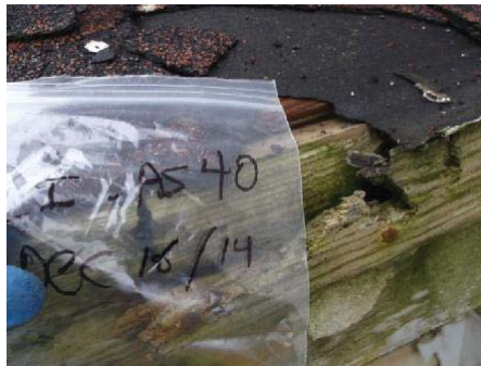
Photo 29: View of tar paper and caulking sample BLI-AS40.
