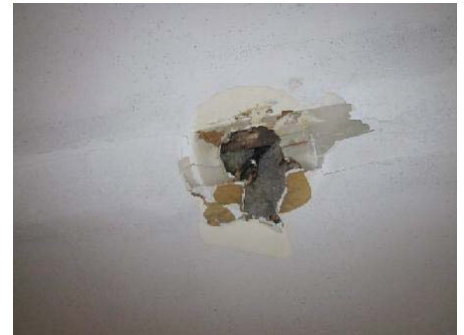
Photo 39: View of location of insulation sample BLI-AS11.
