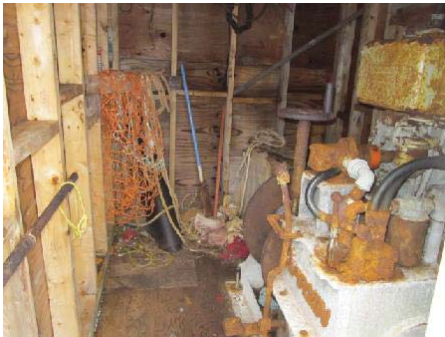
Photo 7: View of interior of lower winch house.
