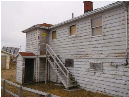
Photo 1: View of southeast side of double dwelling.
