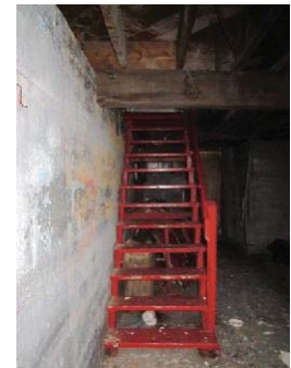
Photo 24: View of Basement 2 in double dwelling.
