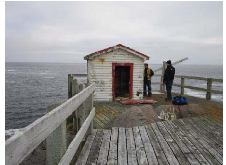
Photo 3: View of upper landing deck and winch house. Note: missing spar and boom.
