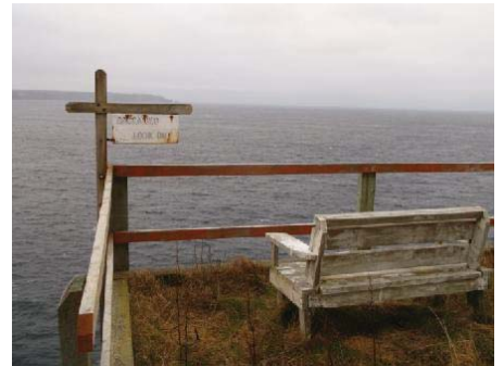
Photo 9: View of railing around lookout area next to double dwelling.
