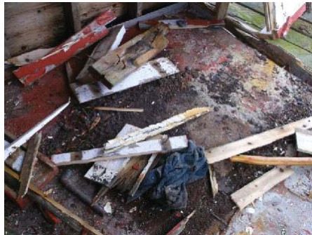
Photo 8: View of interior of upper winch house.
