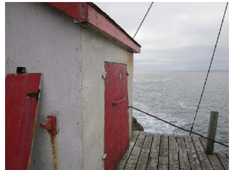
Photo 6: View of northwest side of lower winch house.
