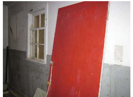
Photo 6: View of Room 1 in old equipment building.
