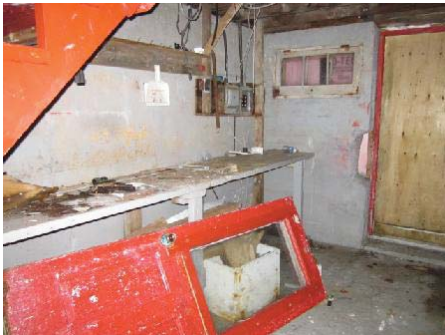
Photo 25: View of Basement 2 in double dwelling.
