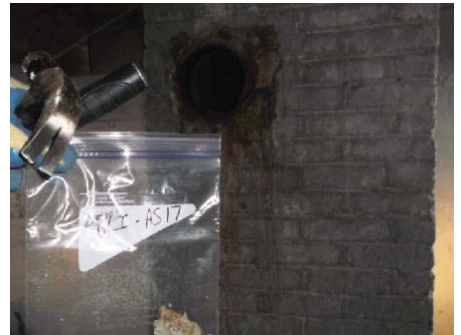
Photo 45: View of brick mortar sample BLI-AS17.
