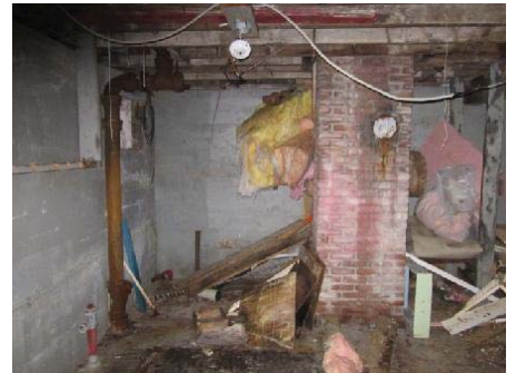
Photo 27: View of Basement 2 in double dwelling.
