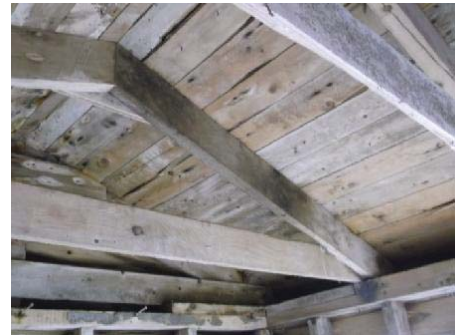
Photo 9: View of interior of upper winch house.
