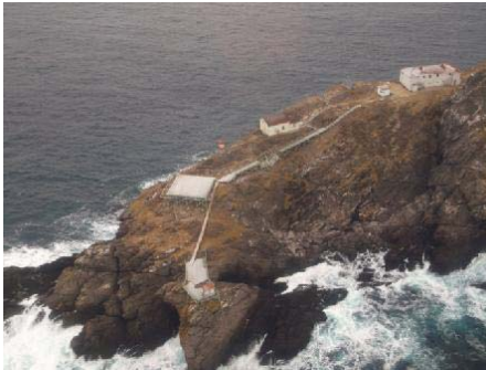
Photo 4: View of Baccalieu Island Lightstation.
