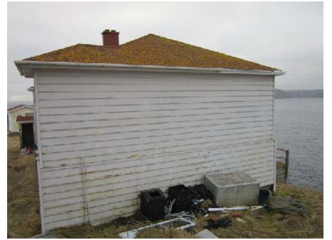
Photo 6: View of northeast side of double dwelling.
