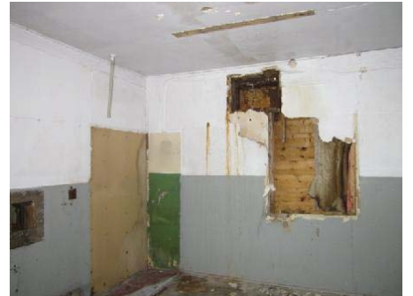
Photo 12: View of Room 3 in old equipment building.
