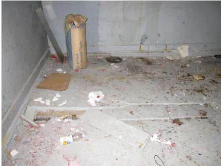
Photo 7: View of Room 1 in old equipment building.
