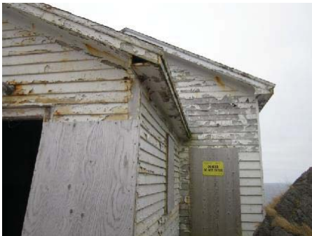
Photo 4: View of north side of old equipment building.
