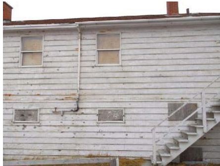
Photo 2: View of southeast side of double dwelling.
