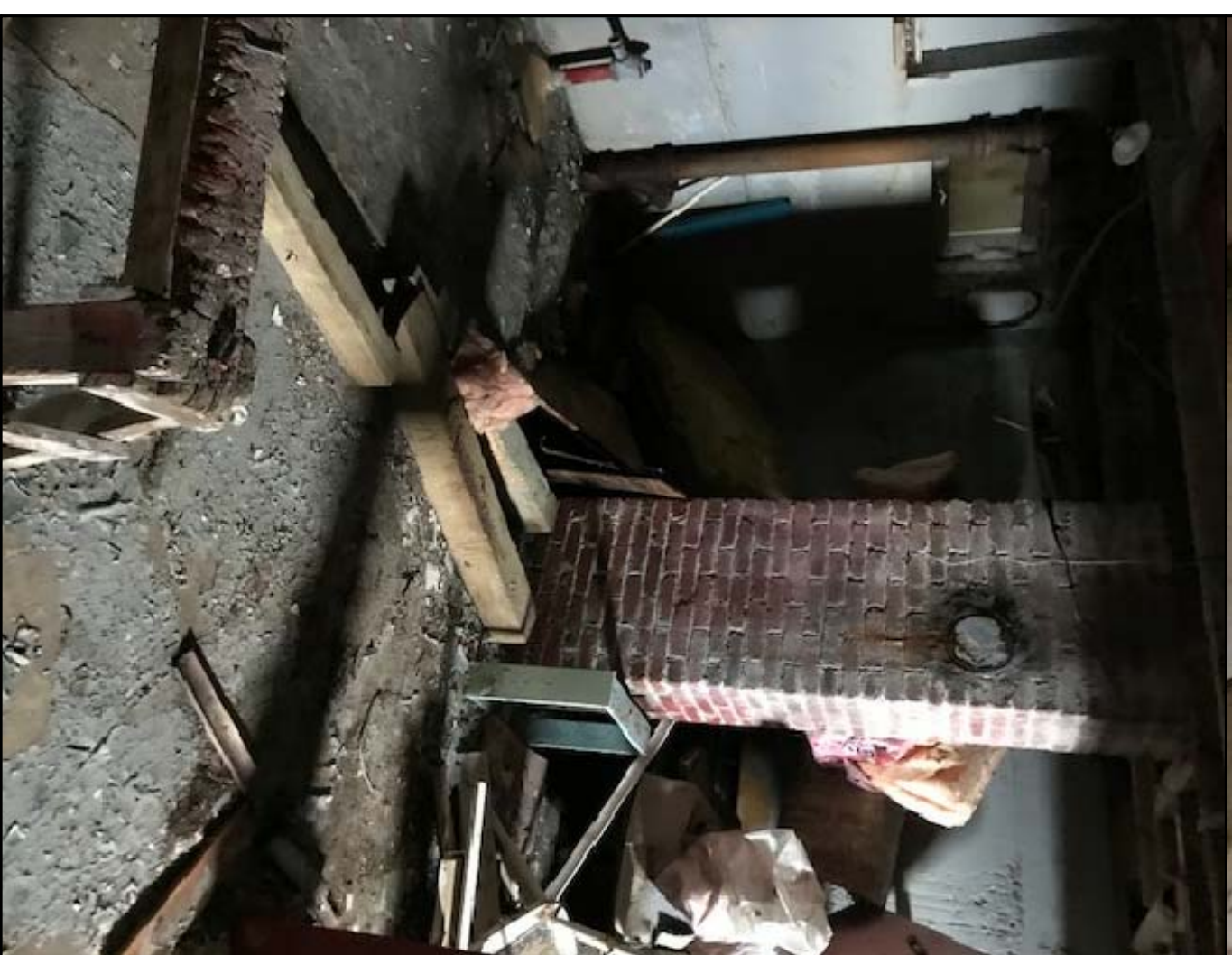
REMOVAL OF VARIOUS SURPLUS INFRASTRUCTURE AT THE BACCALIEU LIGHTSTATION, NL
