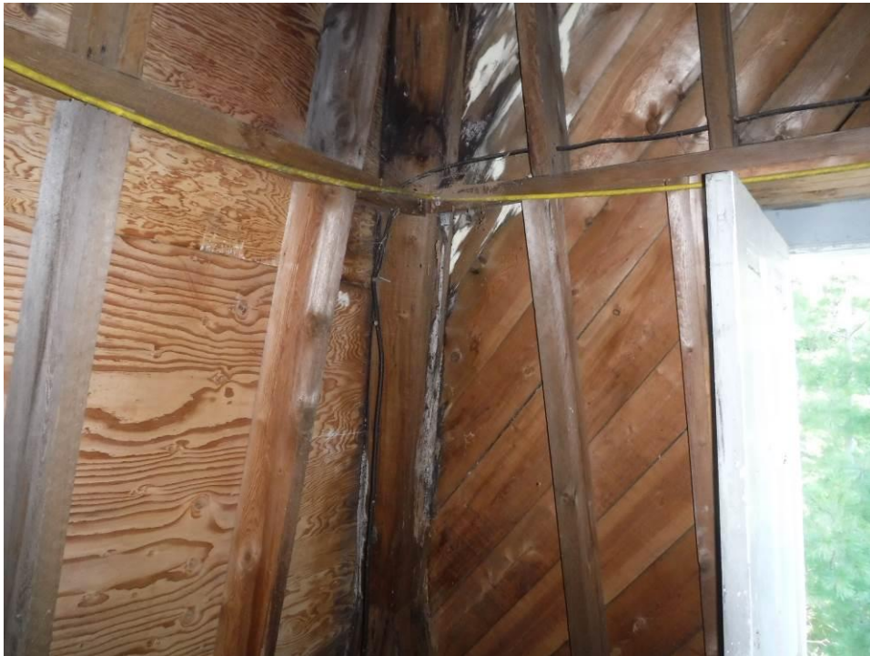
Figure 10 – Existing tower, interior rott
