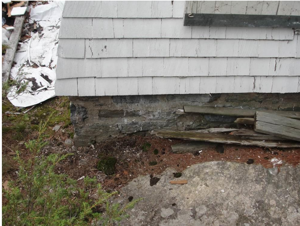
Figure 9 – Stone foundation to be demolished. Height varies around perimeter of structure.
