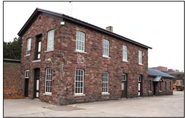
Figure 2: The east elevation of the Workshop. [CLA-PWGSC/November 2012]
