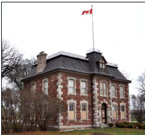
Figure 3: The south elevation of the Office Building. [CLA-PWGSC/November 2012]
