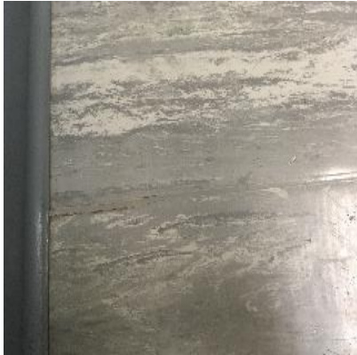
Photo 3: Vinyl sheet flooring observed in building.
